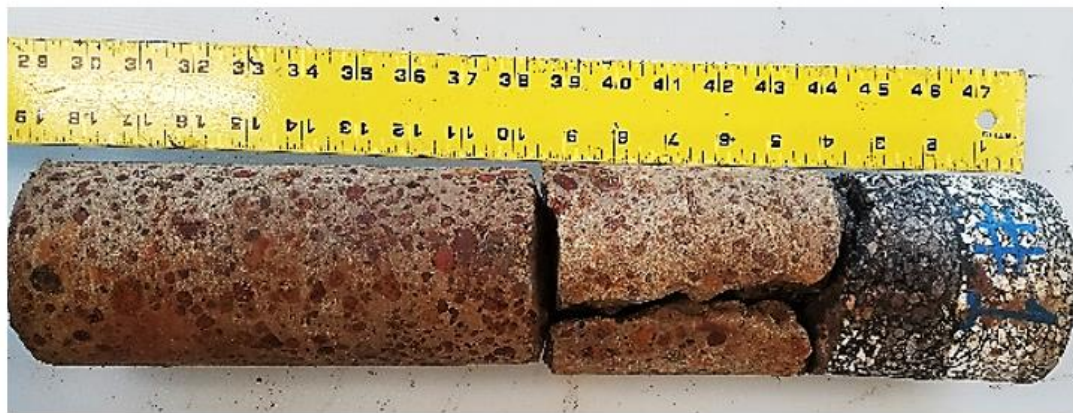
Figure 27. Main Pavement Core.
