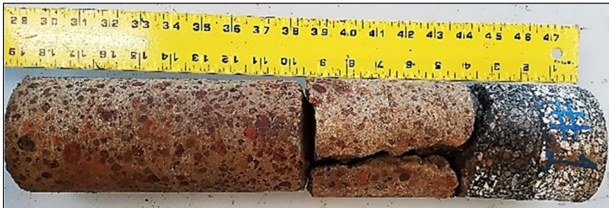
Figure 36. Existing Pavement Core.
