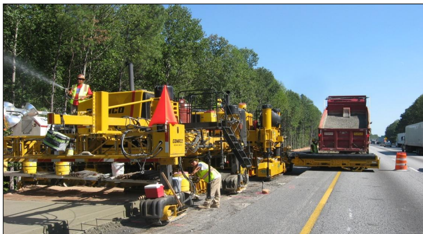
Figure 5.11 Gomaco 2600 Placer/Spreader as solution to work area issues
