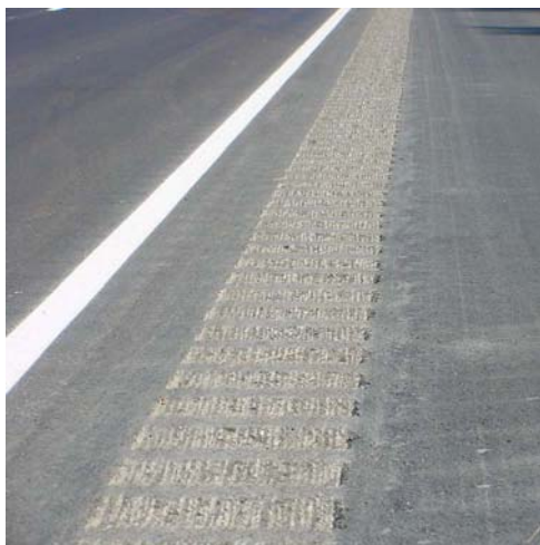
Figure 1. Picture of Milled Rumble Strips (Courtesy of WSDOT)
