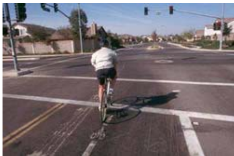
Figure 2. Bicyclist near rumble strips
