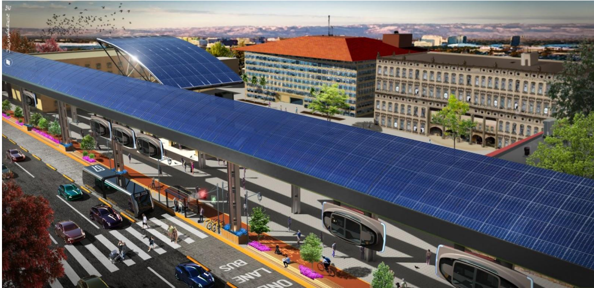
Figure 39. Solar canopies covering the guideway and station.
