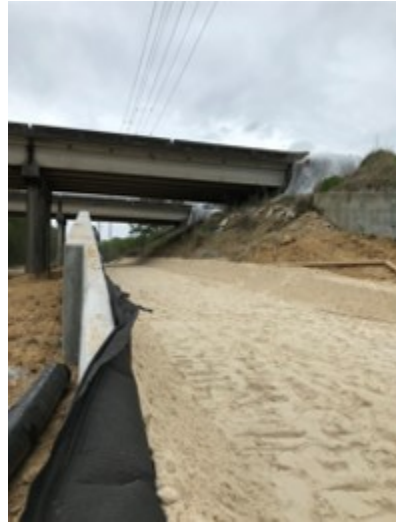
b. North retaining wall
