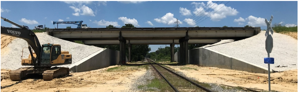
Figure 26. I-55 embankment wall completion
