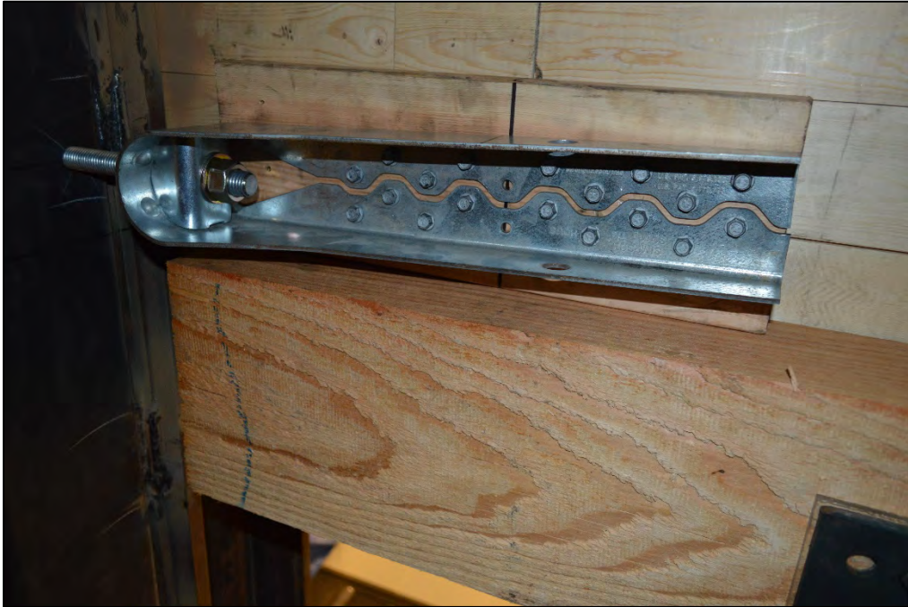
Figure A.19 HDU Hold-down
