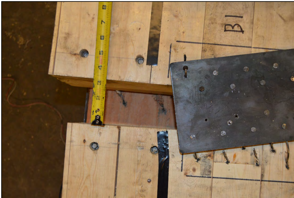
Figure 4.4 Gap between CLT Panels 3 and 4 after the Test
