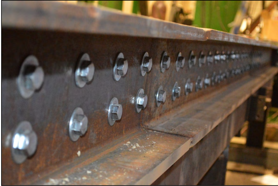
Figure 2.7 West End Steel I-Beam
