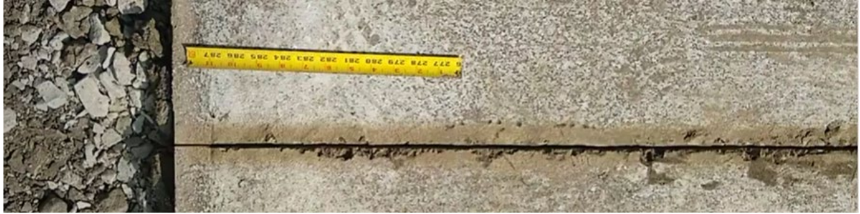
A. Control mix: saw cut after 4 hours 25 minutes
