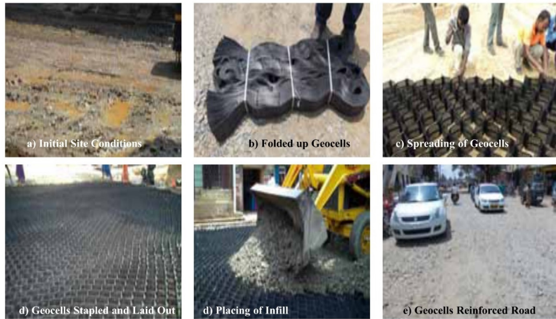
Figure 2-3 Geocell Construction Sequence.
