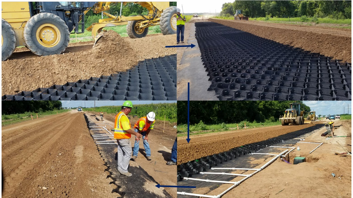
Figure A-22 Geocell Construction Sequence.
