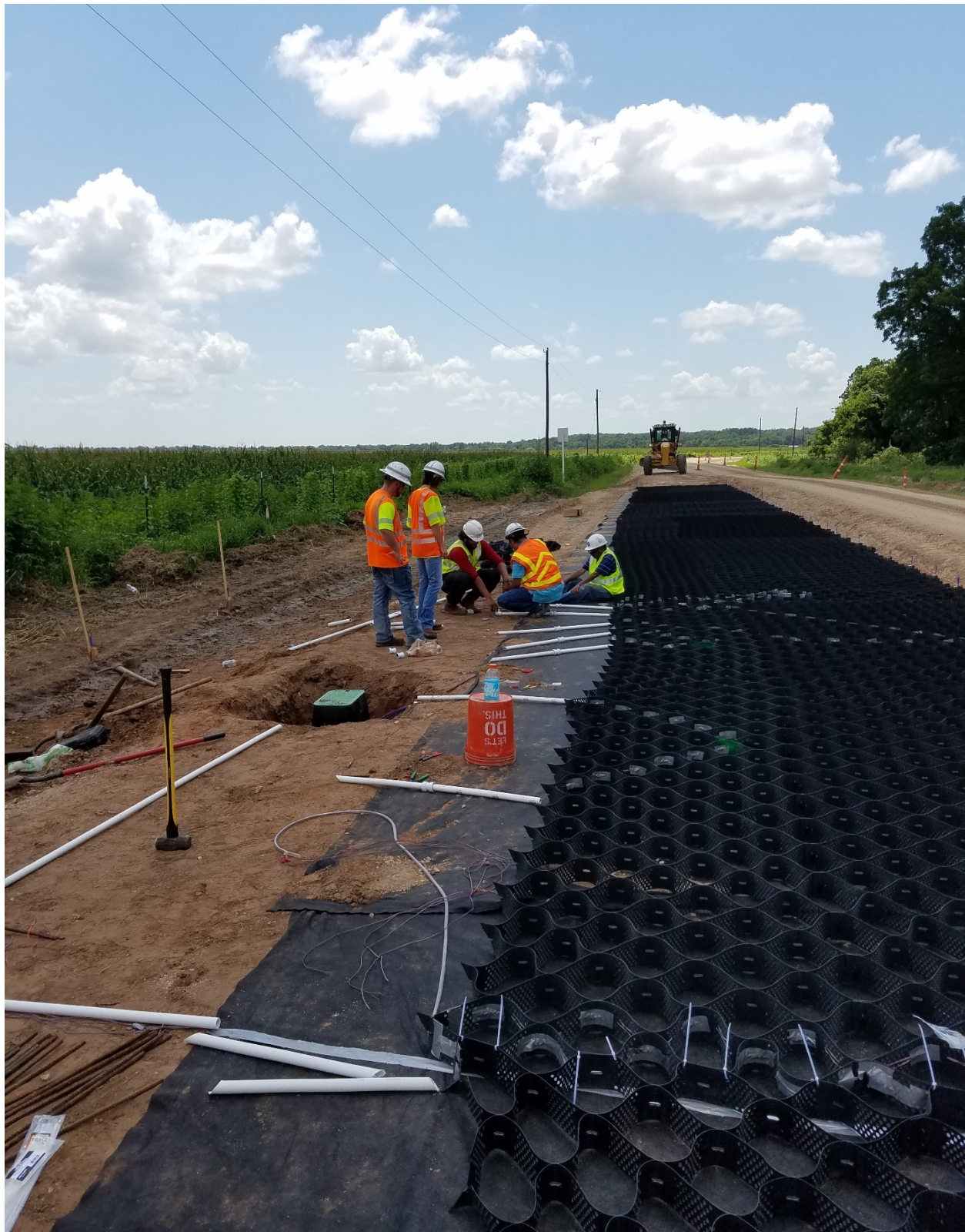
Figure A-21 Installation of Instrumented Geocells.
