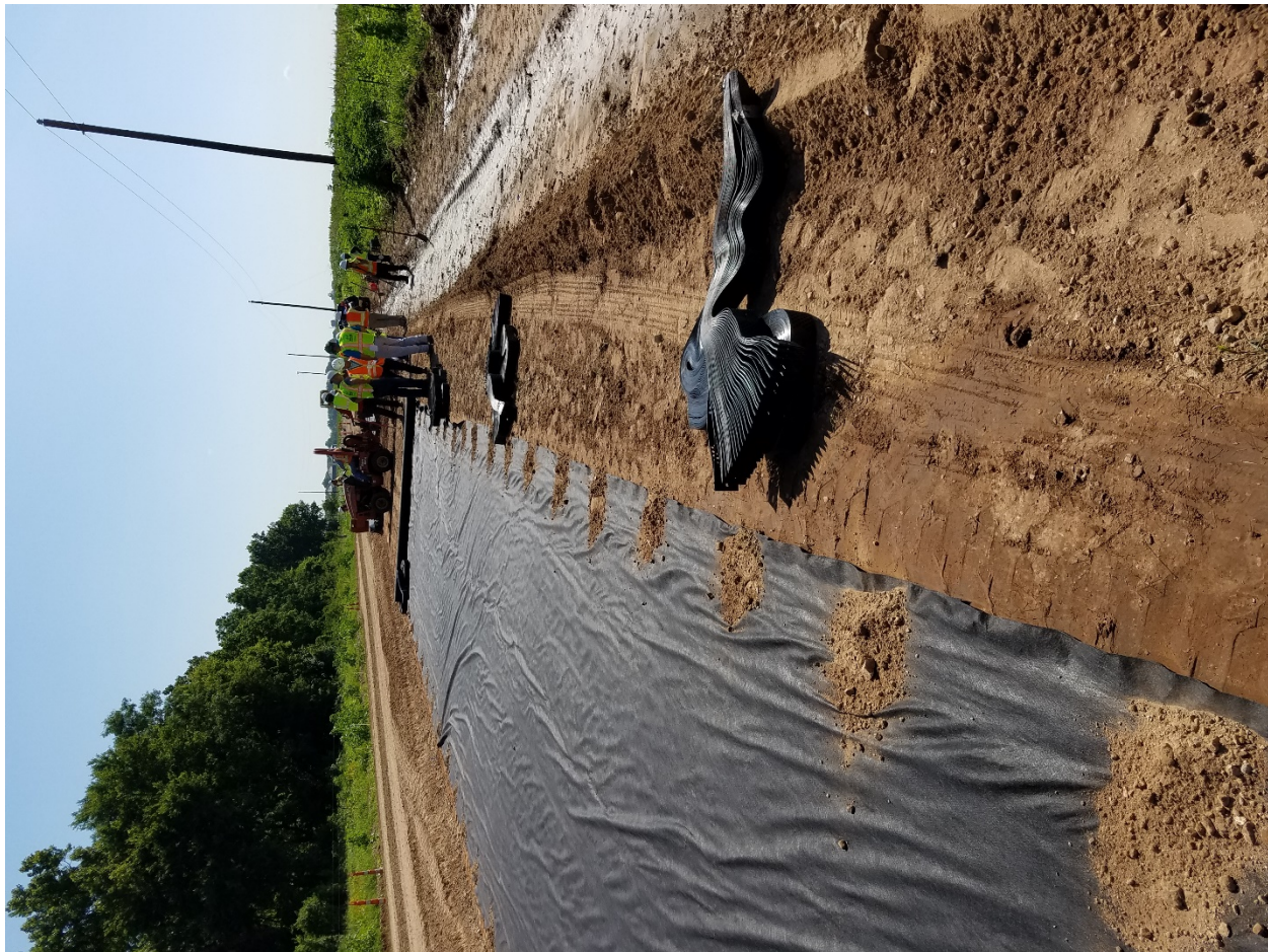
Figure A-20 Installation of Geosynthetics.
