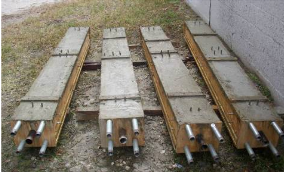
Figure 4-6 Piles with formwork (after pouring concrete).
