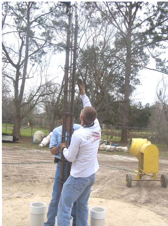
Figure 5-38 Lowering the rebar cage into PVC casing.
