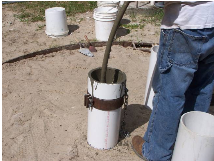
Figure 5-6 Concrete vibrated with a wand.
