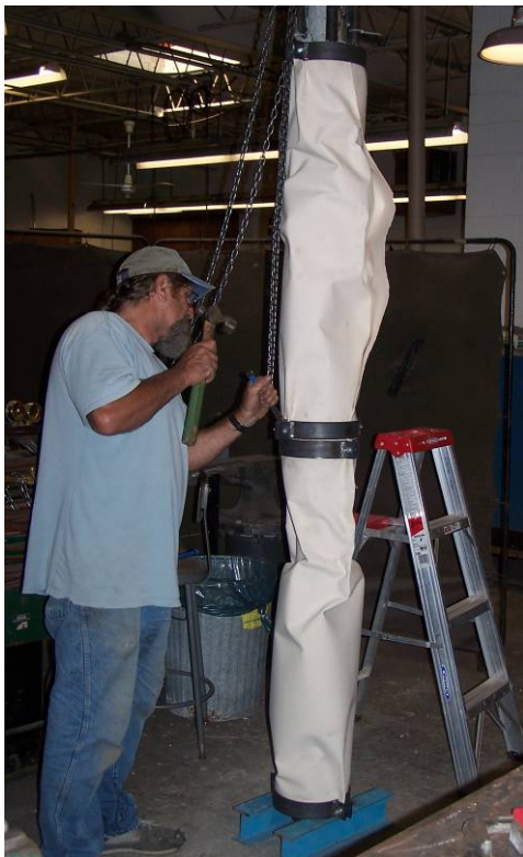
Figure 4-60 Attachment of semi-rigid membrane to pile.
