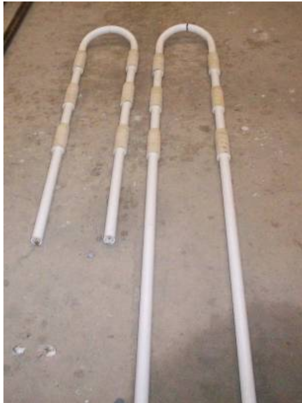
Figure 4-4 Grout delivery pipes.
