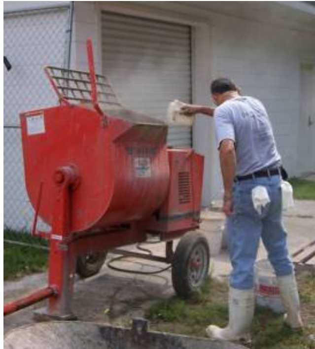
Figure 4-20 Grout mixing using mortar mixer.
