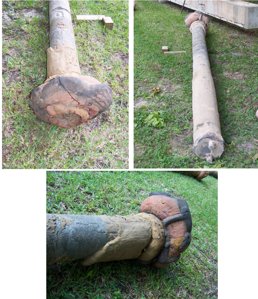
Figure 5-45 Grout zone–West shaft.
