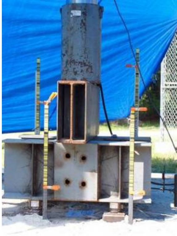
Figure 4-26 Example of barcode strips positioned on each pile for displacement monitoring.
