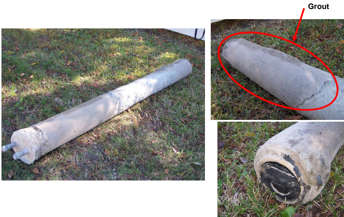
Figure 7-9 Grout-tipped drilled shaft after excavation.
