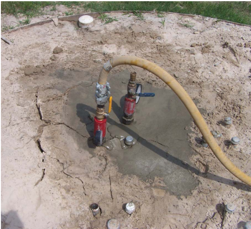
Figure 4-23 Upward grout flow through the ground surface near the pile.
