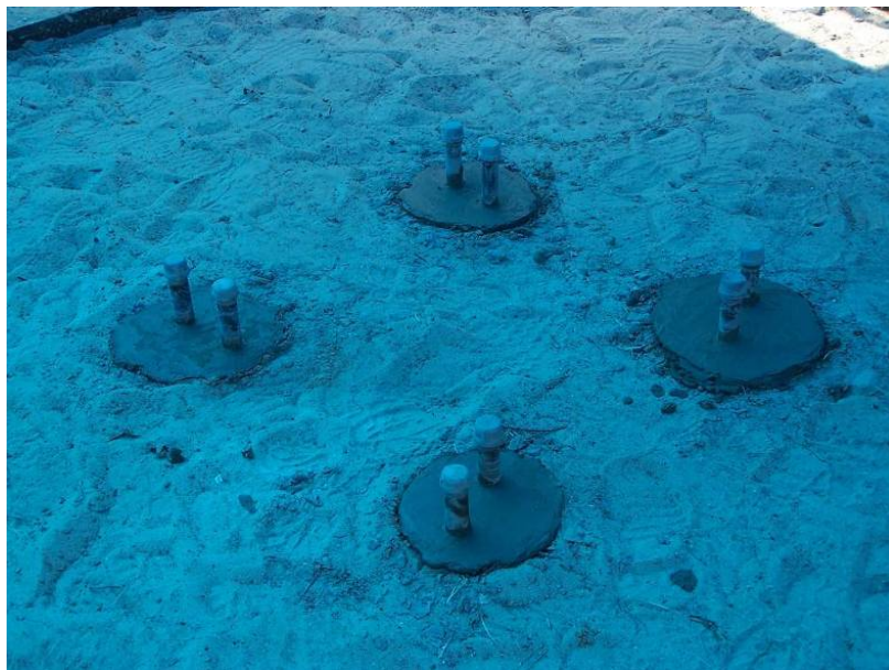
Figure 5-8 Drilled shafts.
