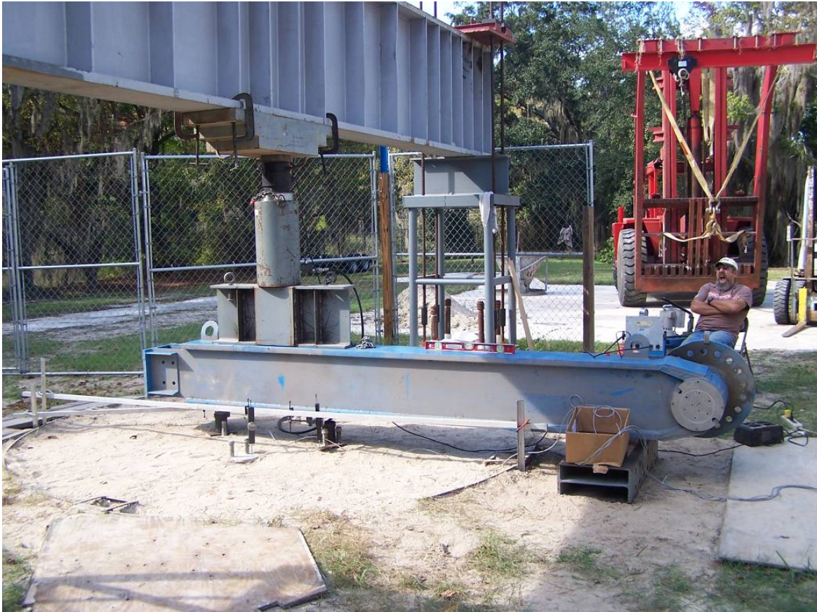
Figure 5-13 Load test setup—South shaft.
