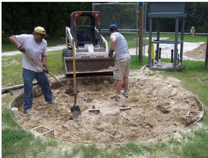
Figure 4-31 Hand excavation of the top of the pile group.
