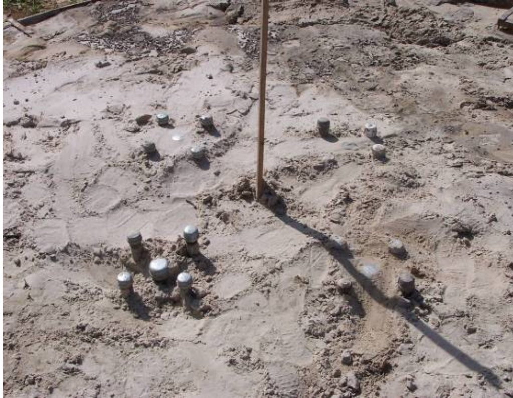
Figure 4-19. Piles jettied into the ground.
