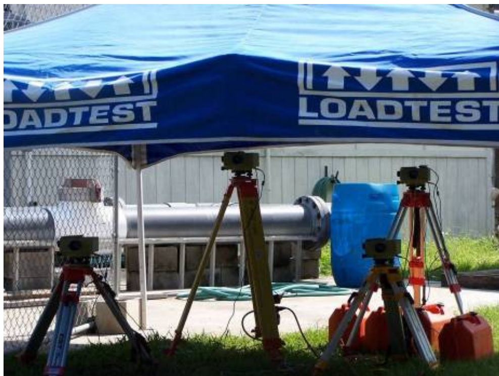
Figure 4-25 Digital levels for pile displacement monitoring.
