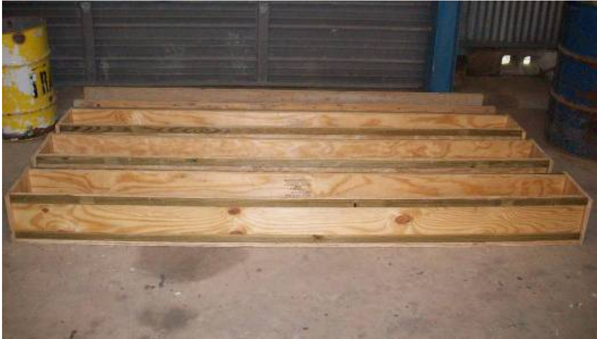
Figure 4-3 Formwork for casting piles.
