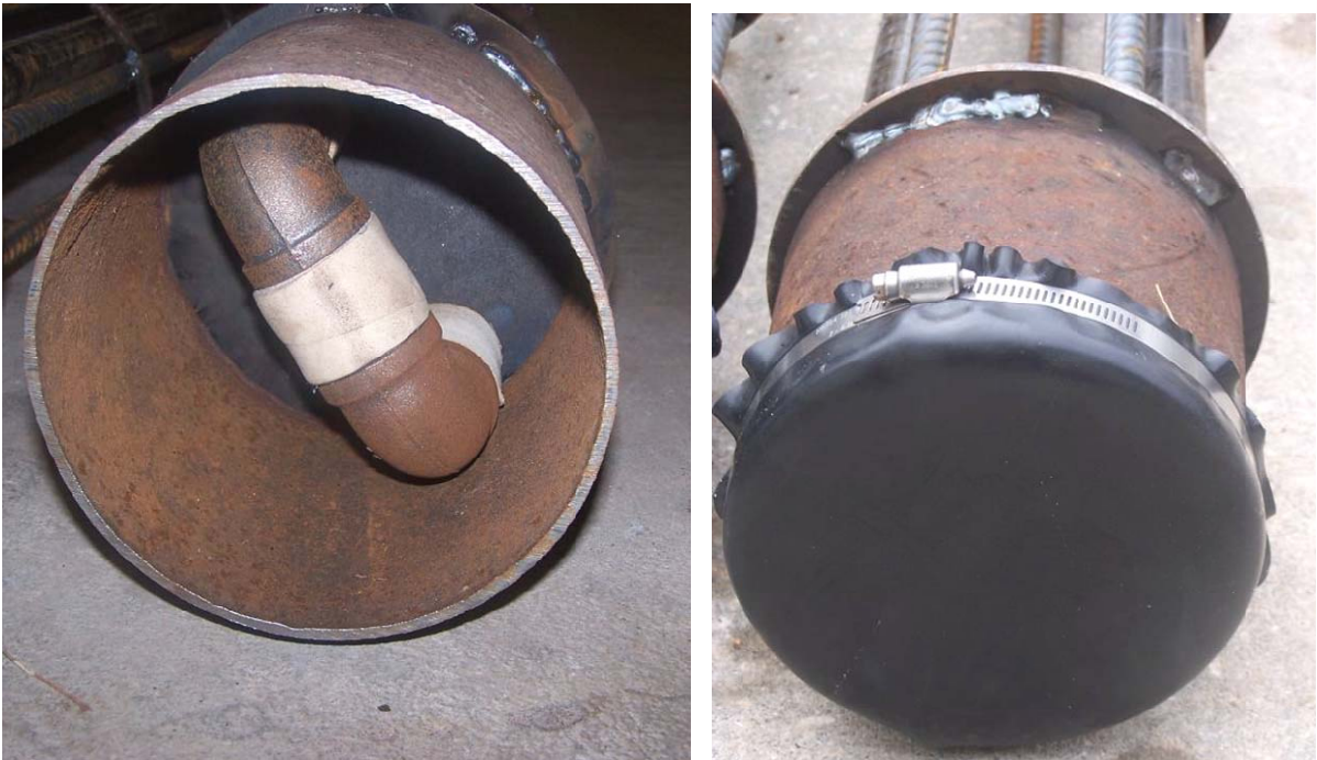
Figure 5-35 Grout exit and membrane covering.
