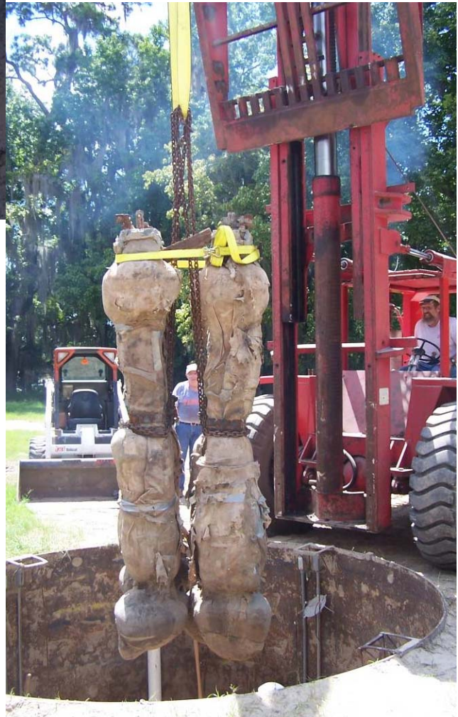
Figure 4-34 Lifting of the pile group using fork lift.
