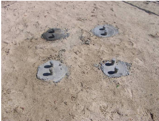
Figure 5-39 Drilled shaft group after concreting.
