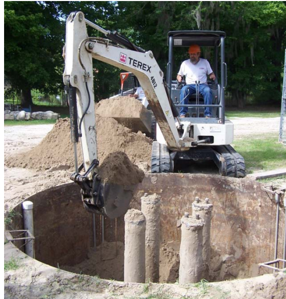
Figure 5-40 Removal of soil from the test chamber.
