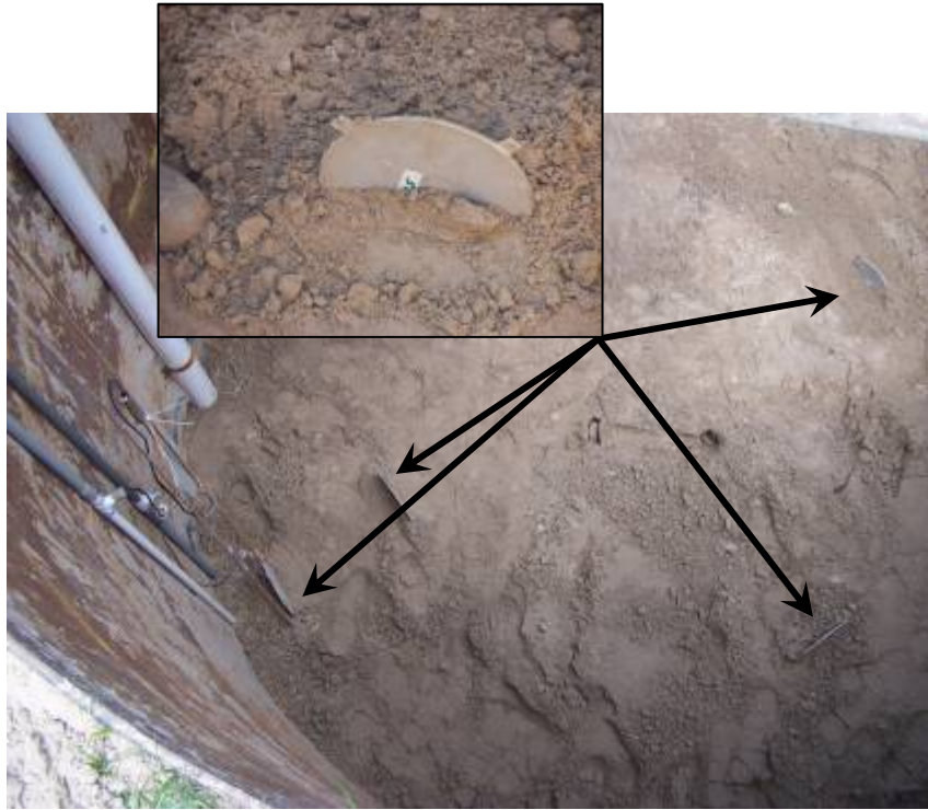
Figure 4-15 Stress gages placed vertically at 8-ft. depth.
