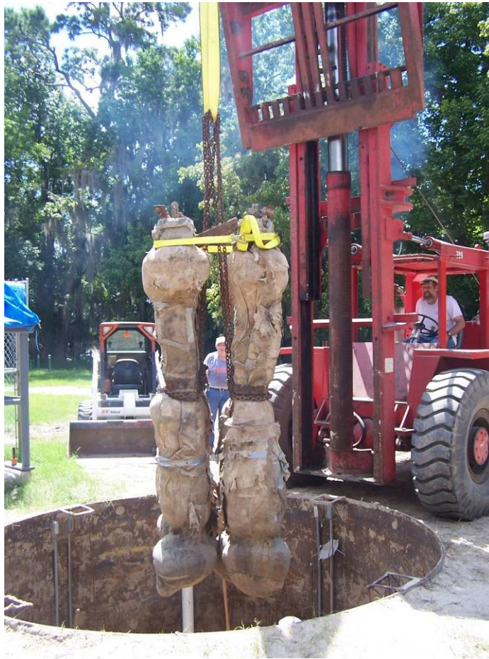
Figure 7-3 Jet-grouted pile group after excavation.
