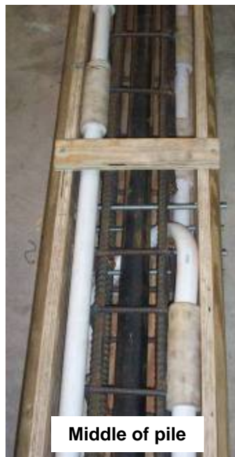
Figure 4-5 Rebar cage, jetting pipe, and grouting systems positioned in the formwork.
