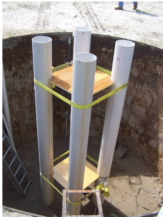
Figure 5-2 PVC casing positioned before filling the test chamber.
