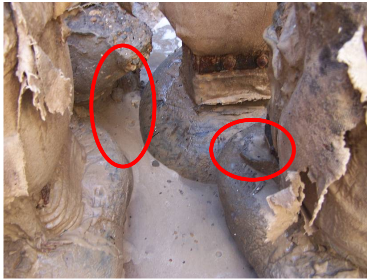
Figure 4-37 Overlapping of tip bulbs.
