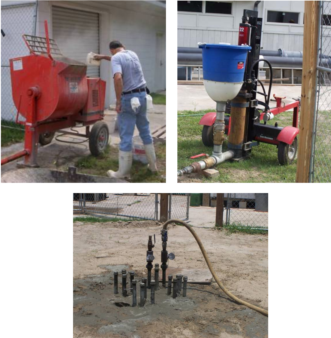
Figure 4-64 Side grouting.
