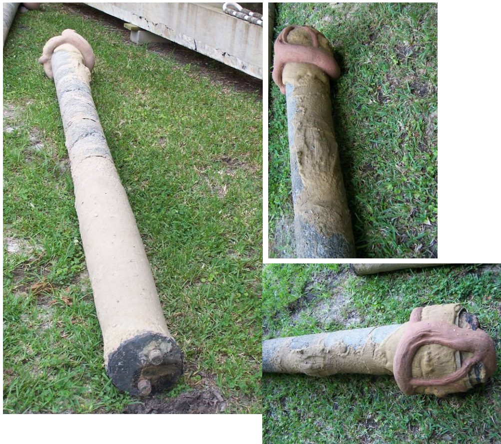
Figure 5-43 Grout zone—South shaft.
