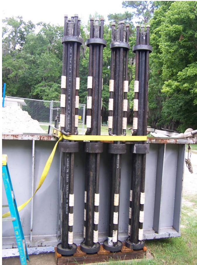
Figure 7-4 Group of 4.5-inch diameter jet-grouted piles with grout delivery systems.
