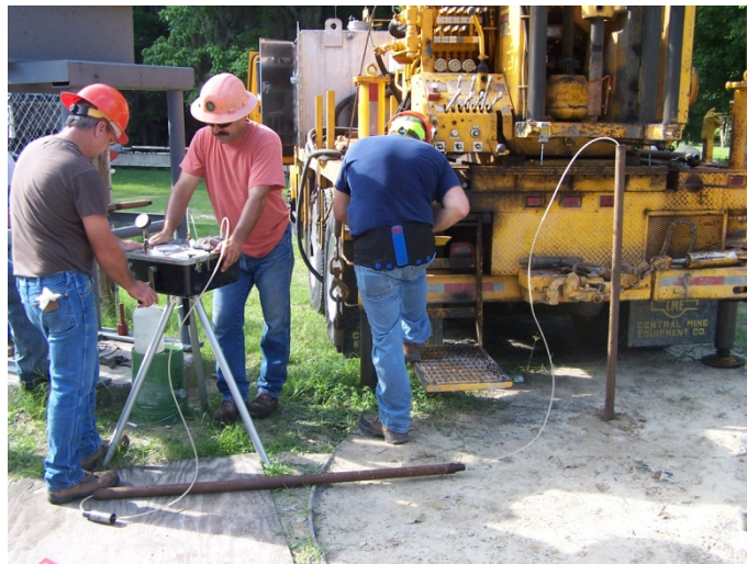
Figure 3-5 Pressure meter testing.
