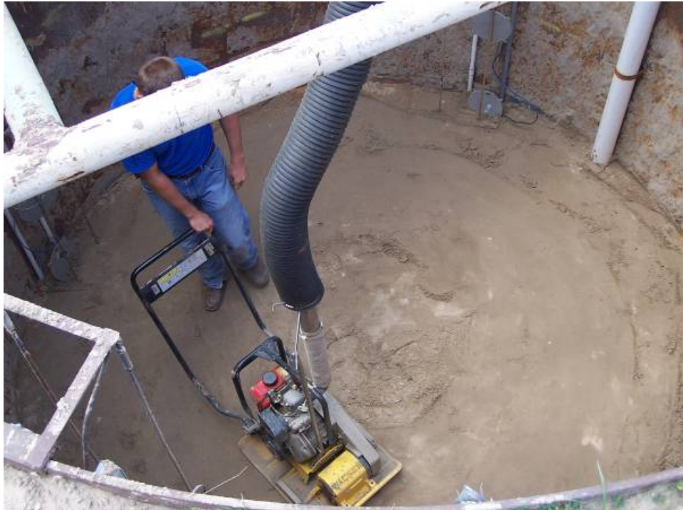
Figure 4-12 Soil compaction using vibratory plate compactor.
