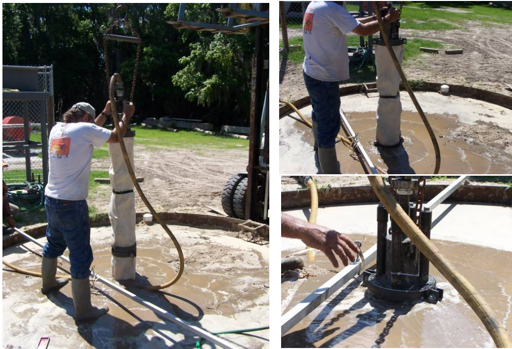
Figure 4-63 Pile jetting.
