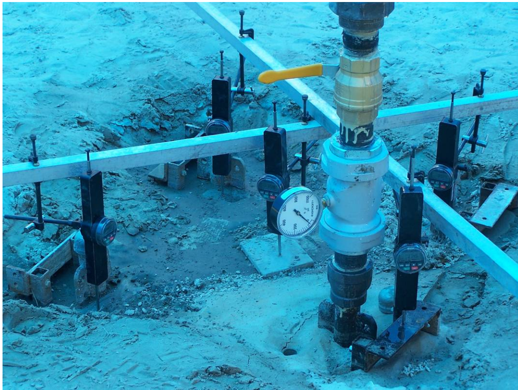
Figure 4-28 Tip grouting of pile.
