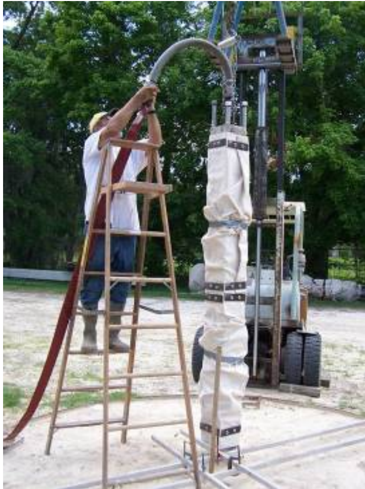
Figure 4-17 Pile prior to jetting.
