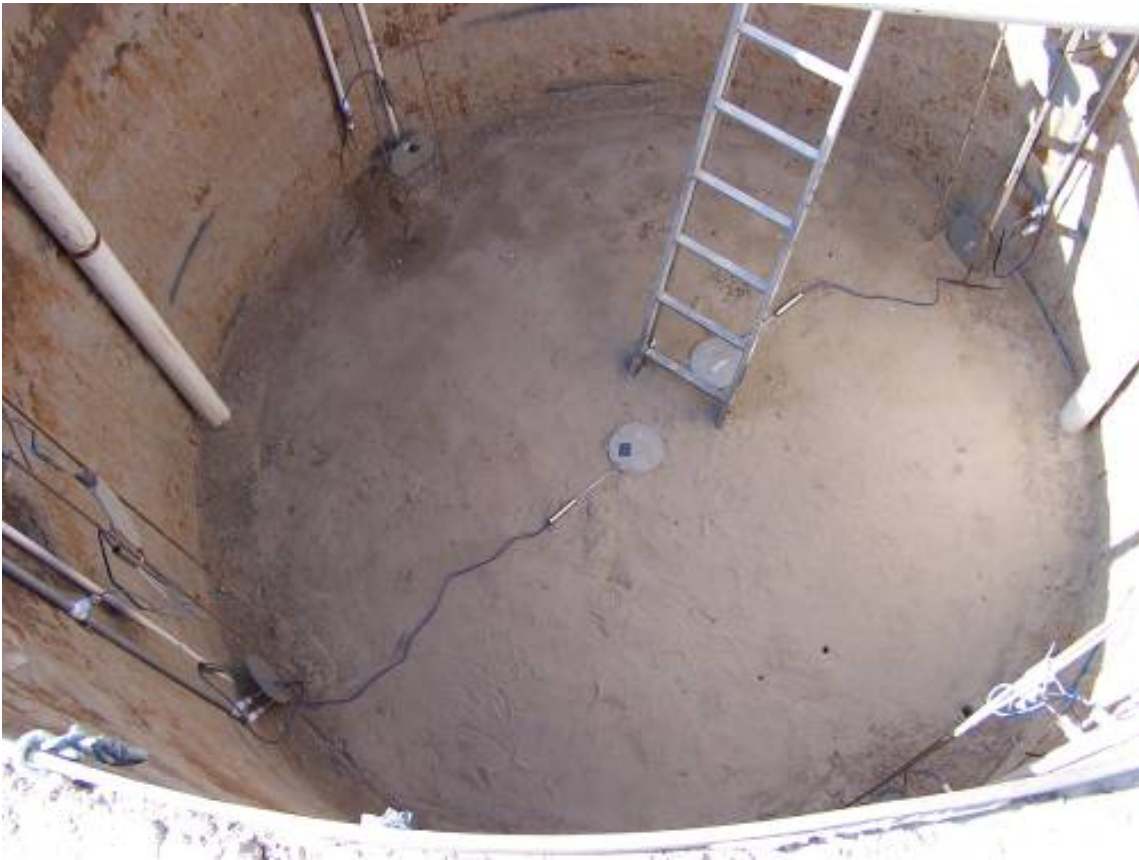
Figure 4-14 Stress gages placed horizontally at 10-ft. depth.
