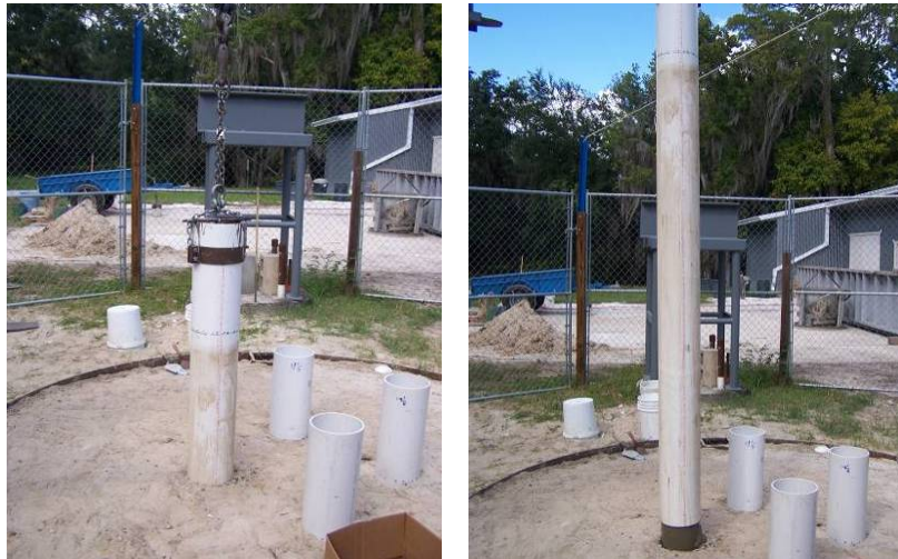
Figure 5-7 Pulling the casing out.
