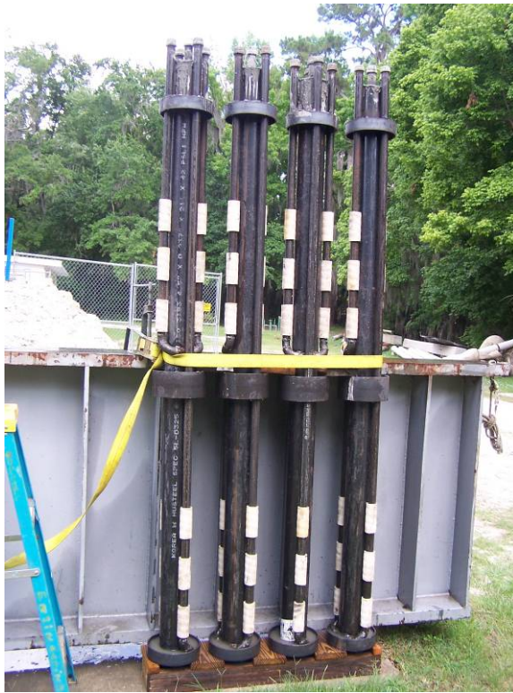
Figure 4-59 Piles after pouring concrete.
