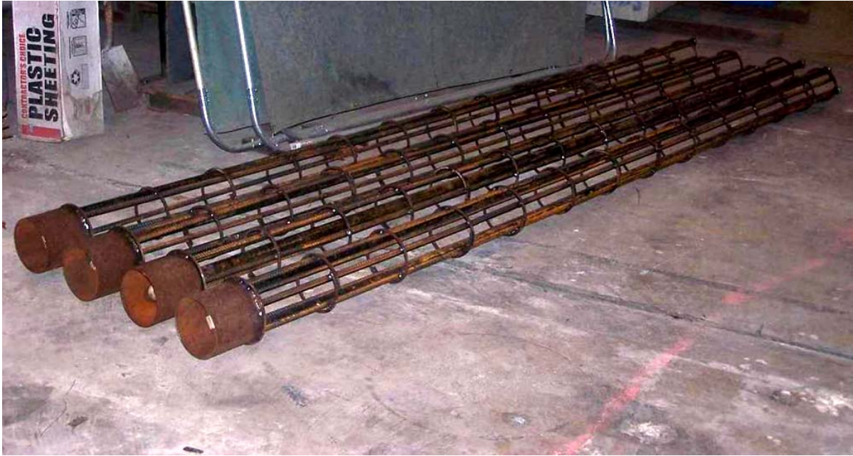
Figure 5-34 Rebar cage for the drilled shafts.
