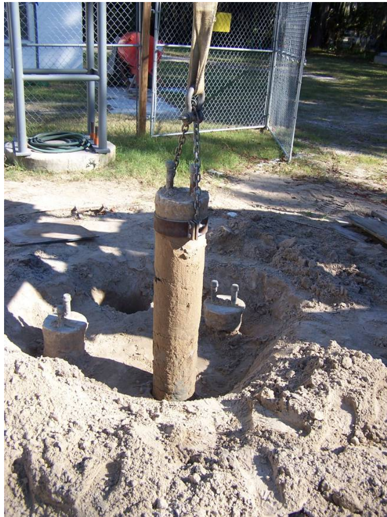
Figure 5-14 Pulling out drilled shaft.
