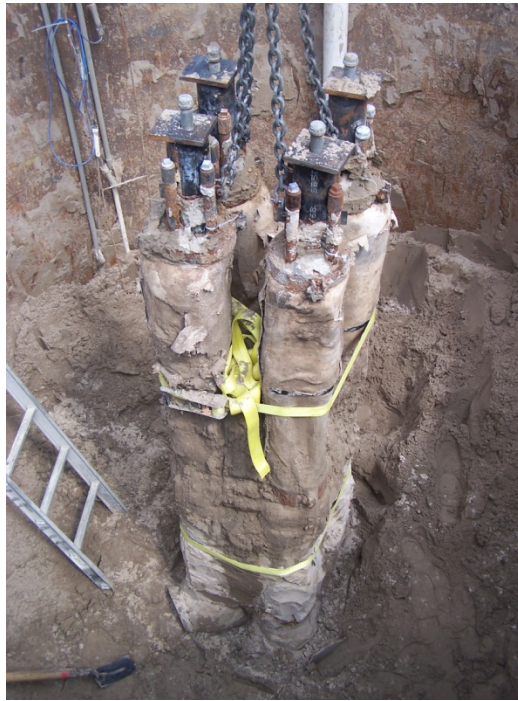
Figure 4-65 Jet-grouted pile group in the test chamber.
