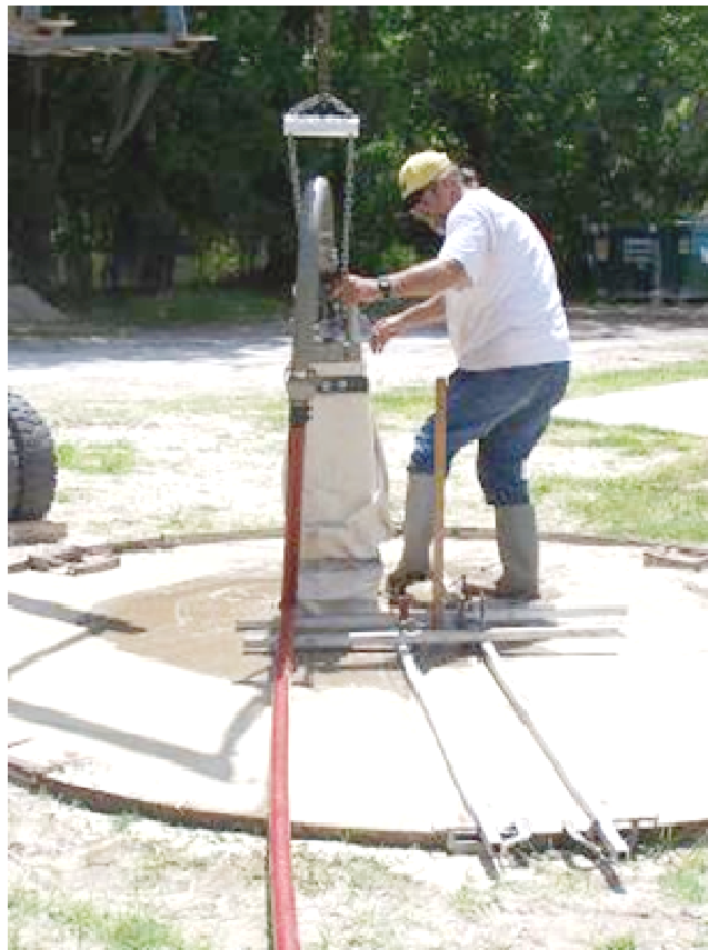
Figure 4-18 Pile during jetting.
