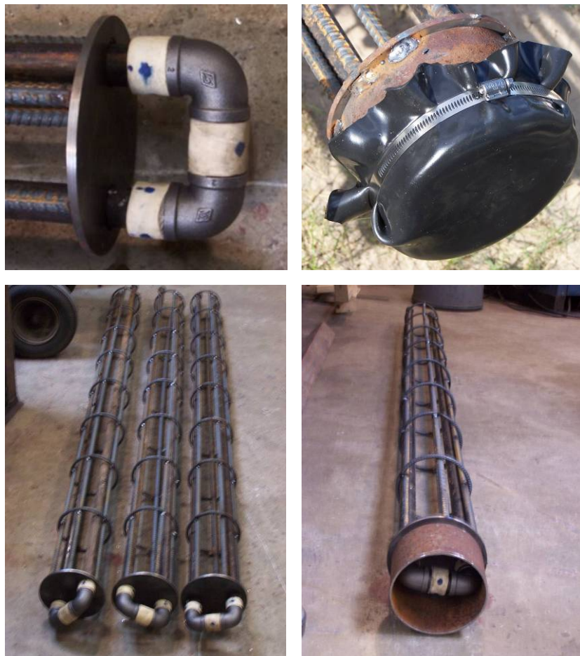
Figure 5-1. Rebar cage and grout system.
