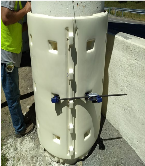
Figure A 7 - Using a bar clamp to pull the seam together.
