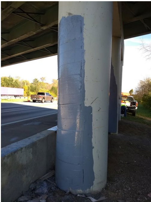
Figure C 8 Citadel patch FRA 270-960 west column after 2 years.
