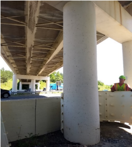
Figure A 9 - Wrapping the shields
