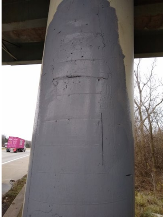
Figure C 10 - Creative Materials patch FRA 270 960 center column after 2 years.
