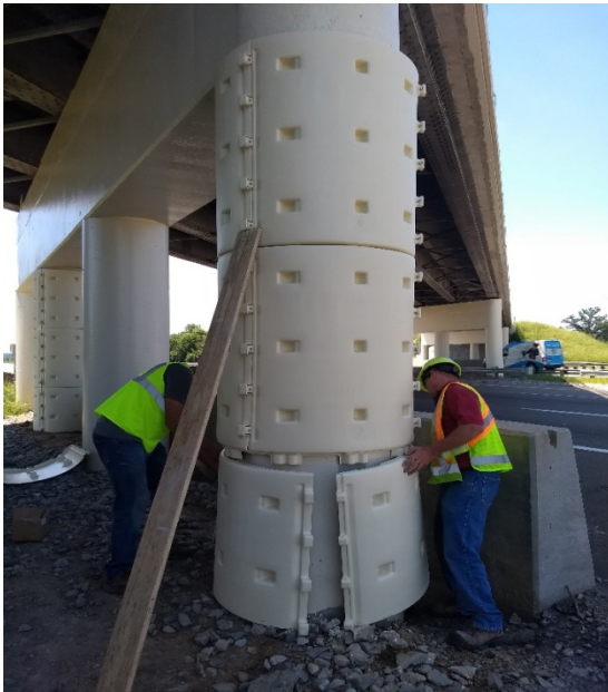
Figure A 10 Assembling a stack of rings.
