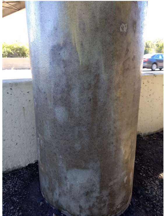
Figure C 2 - Column with first coat of primer applied.
