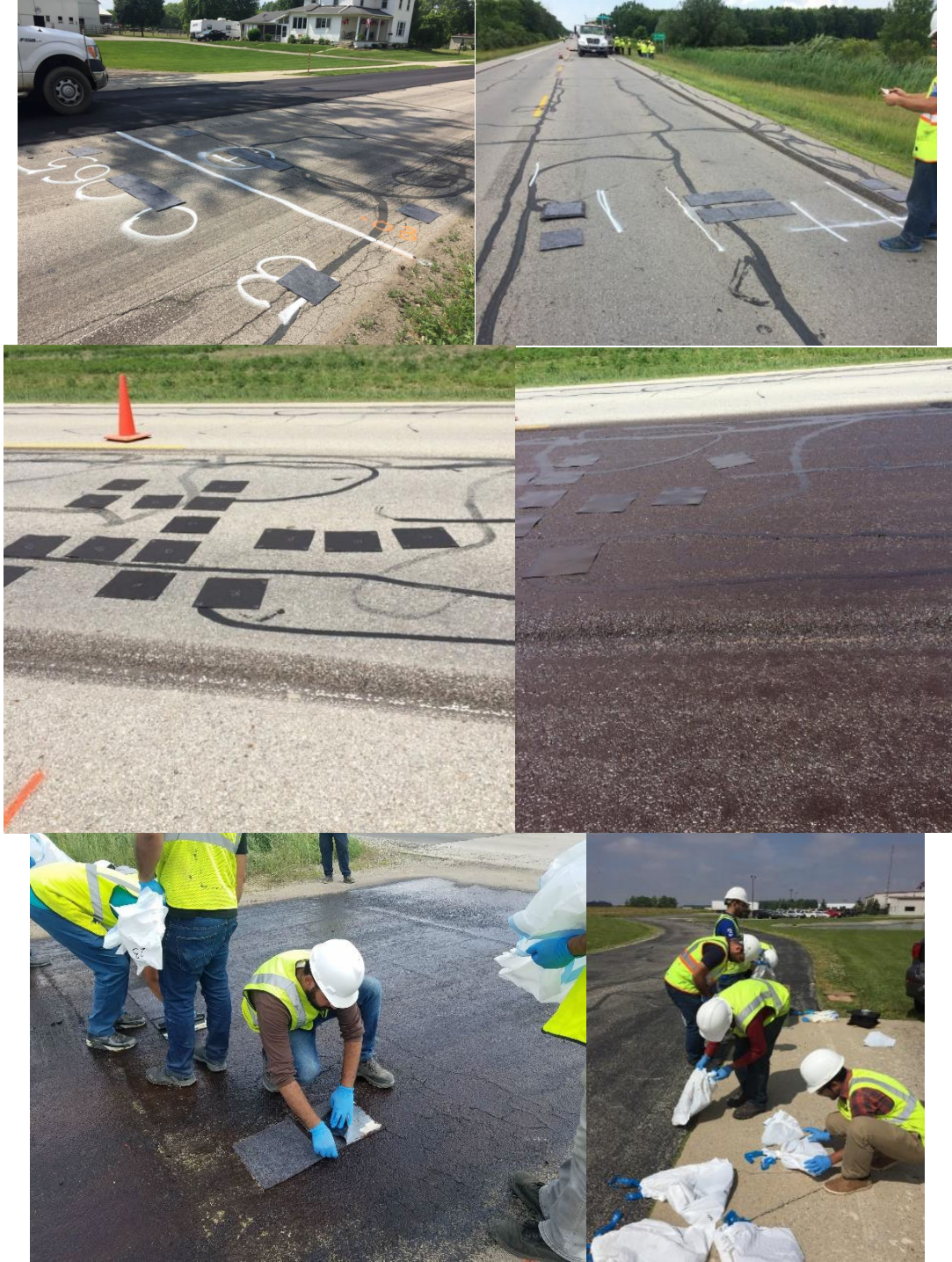
Figure A.5 Photographs taken during measuring the tack application rate.
