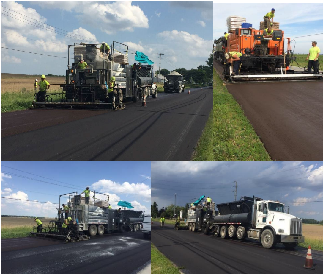
Figure A.6 Photographs taken during the installation of micro-surfacing course.
