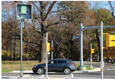
Battery-powered AVTS radar housed in weatherproof case on adjustable-height tower. Source: FHWA.
