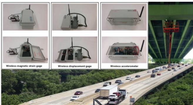
The sensors pictured in the inset image—wireless magnetic strain gauge (left), wireless displacement gauge (middle), and wireless accelerometer (right)—were tested on this 11-span viaduct carrying Interstate 76 west of Philadelphia, PA. © Drexel University.
