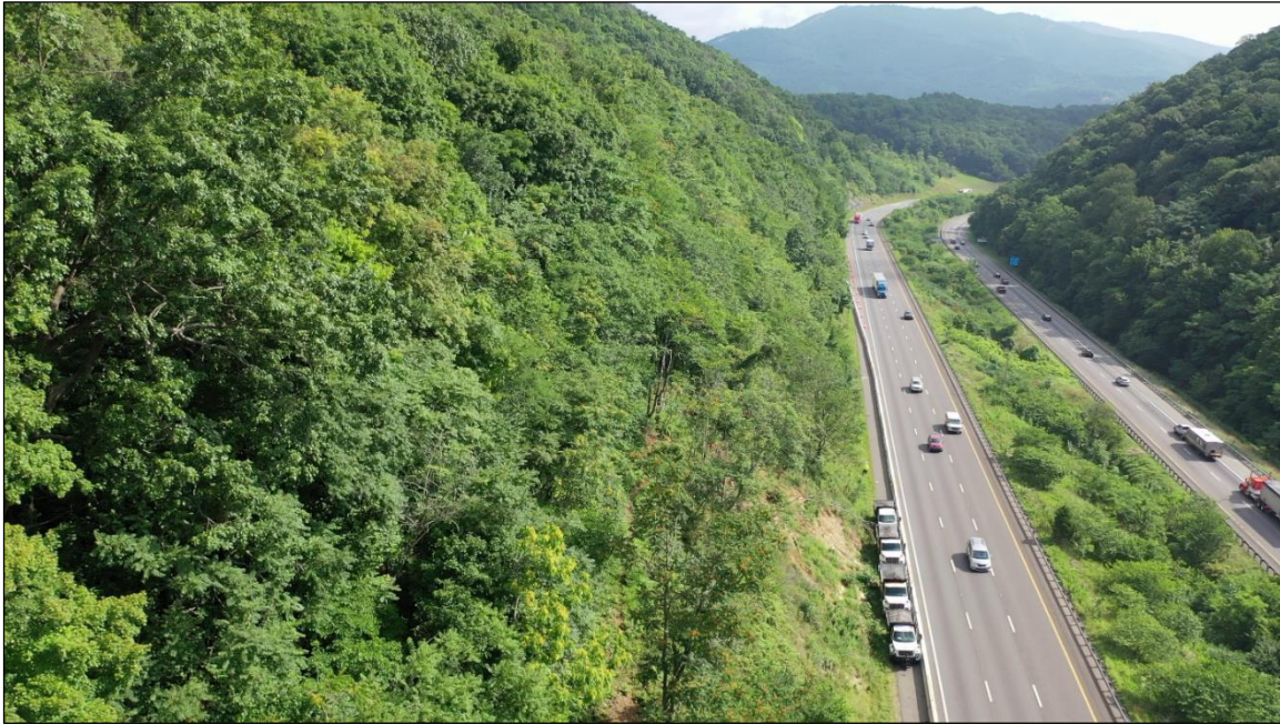
Figure 7. UAS photograph of Site #6, I-81 at MP 126.5 southbound, looking northbound. The current landslide is adjacent to the trucks placed as temporary rockfall barriers. The site of a massive 1969-70 landslide is at, and rising to the left above, the grassy area just beyond the curve in the distance at about MP 127.0. This picture illustrates the challenging nature of the site for UAS flights: dense leaf-on vegetation, narrow valley, rugged median sloping down toward the northbound lanes.
