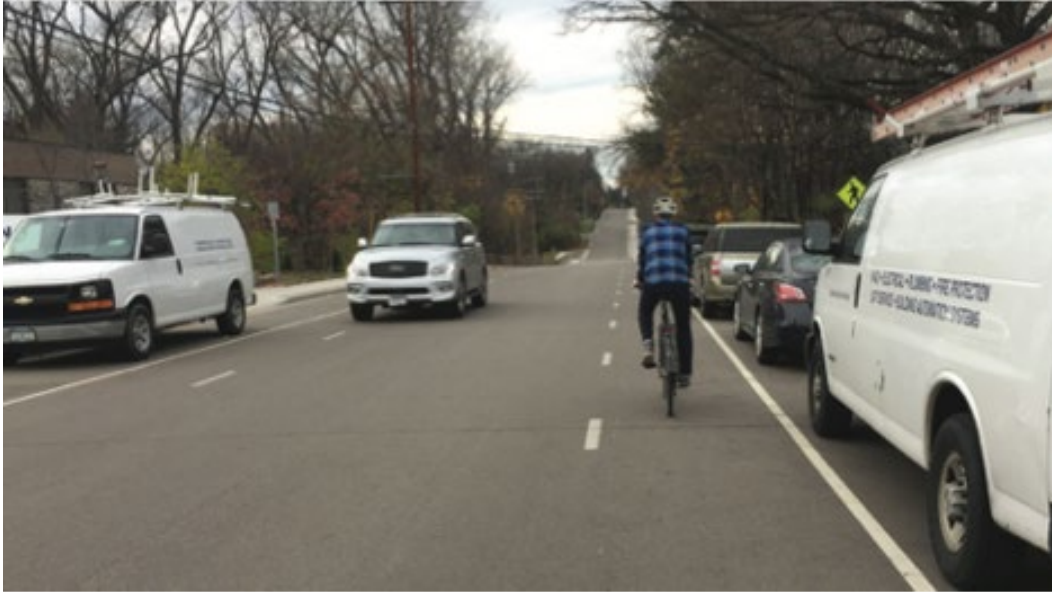
Image of dashed-line flex bicycle lanes on a narrow yield-type roadway. Existing+ micro lanes create flex zones for motorized micro vehicles within roadway travel lanes. (Image: Alta Planning + Design)
