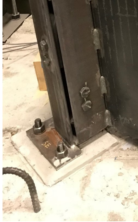
Figure 4.5: Hold-down base plate
