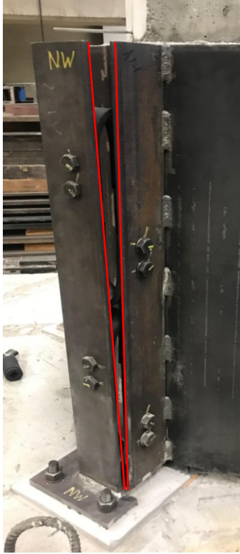
Figure 5.3: Residual hold-down deformation
