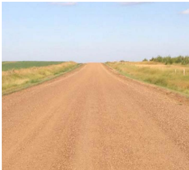
Figure 2.10 Gravel road with adequate crown.
