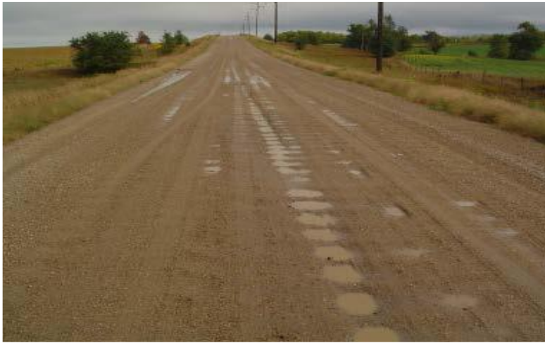
Figure 2.11 Gravel road with inadequate crown
