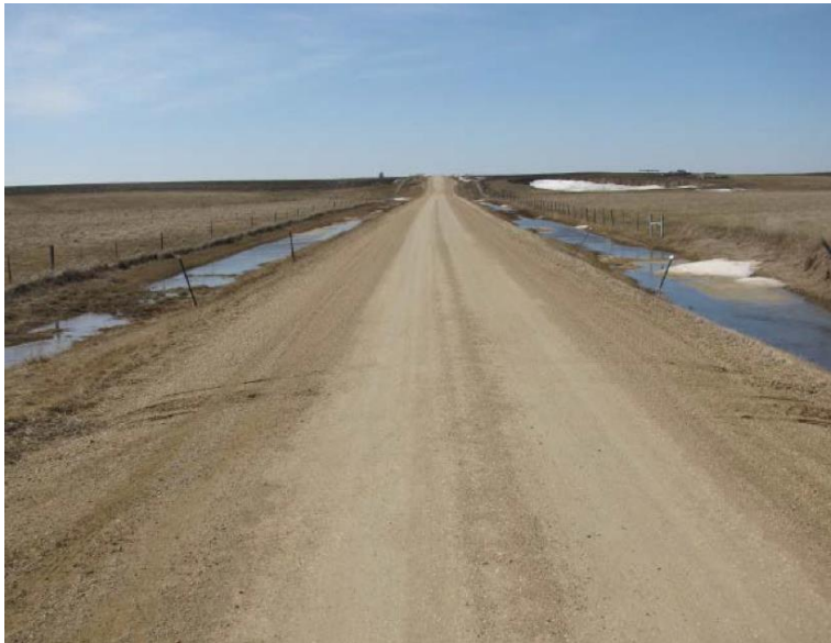
Figure 2.12 Gravel road with excessive crown.
