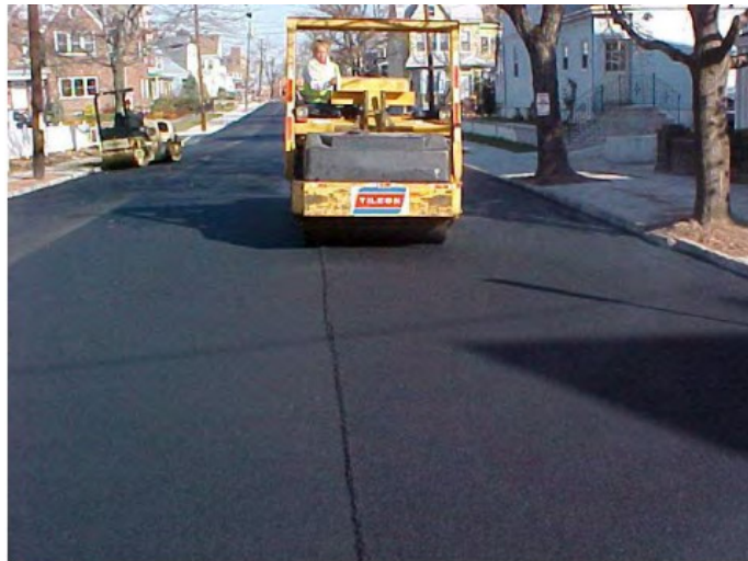
Figure 2.22. Rolling pattern of hot side of the longitudinal joint (Benson and Scherocman 2006)
