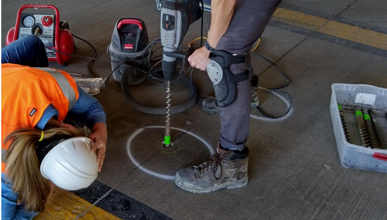
Figure 3-15 Photograph showing the drilling of the chloride penetration sample collection on the ground floor. Current image is of drilling the sample in the wheel-path (according to the paint) and at the epoxy-filled joint.
