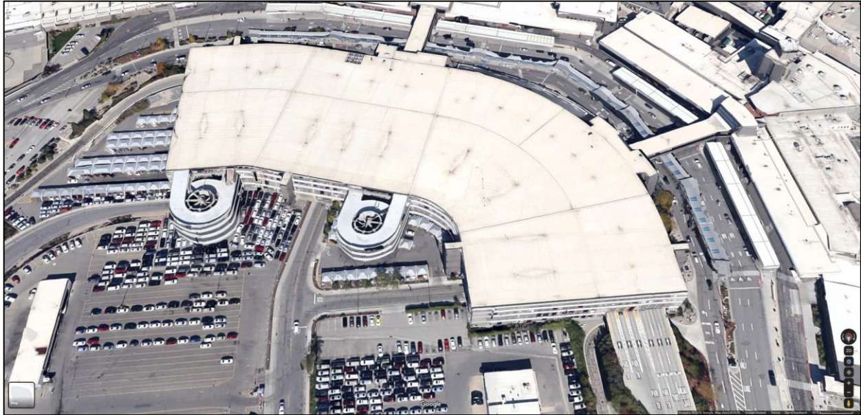
Figure 1-2 3D rendering looking north onto the parking garage, obtained from Google Maps, image from 2020 before demolition began.
