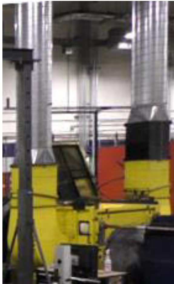
Fig 1: CV dynamometer before starting the conversion
