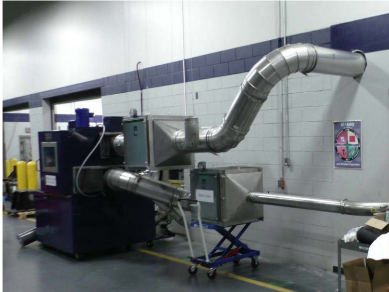
Fig 4: Assembling duct connections to the CCU
