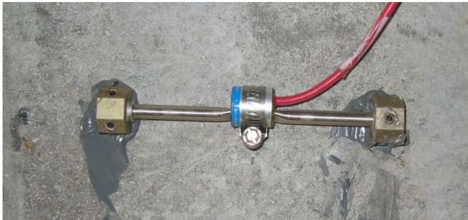
Figure 2.28: Photograph of Mounted Strain Gage on Bottom Flange of Girder
