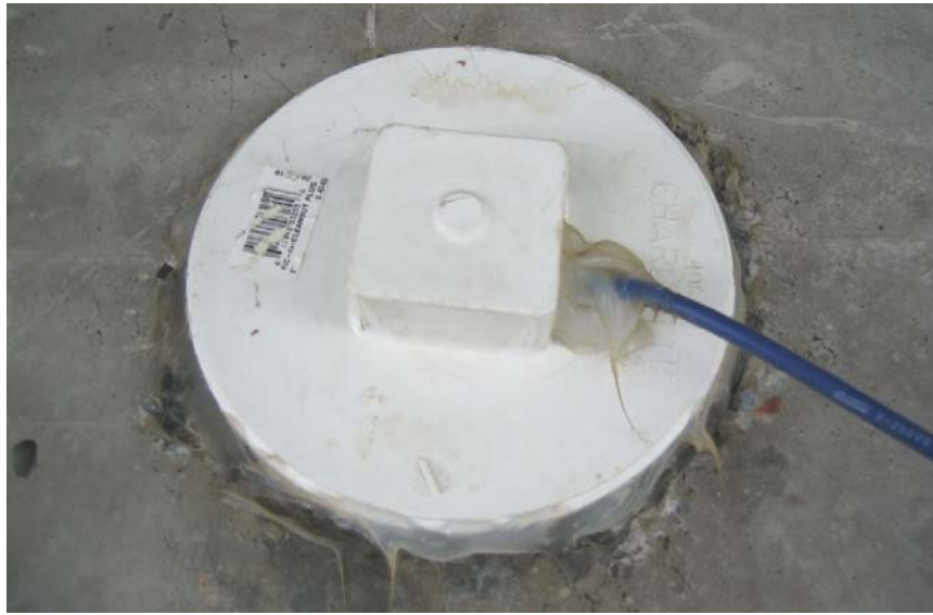
Figure 2.26: Photograph of Extensometer on Front Face of Abutment
