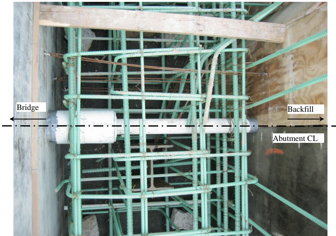
Figure 2.25: Photograph of Plan View of Installed Plastic Tube for Extensometer
