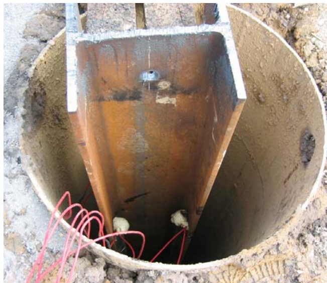
Figure 2.21: Photograph of Strain Gage on H-Pile After Driving
