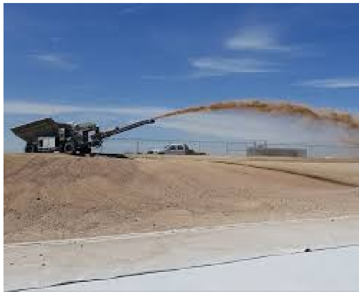
Figure 7 Non-contact placement of unconsolidated soil with a soil slinger
