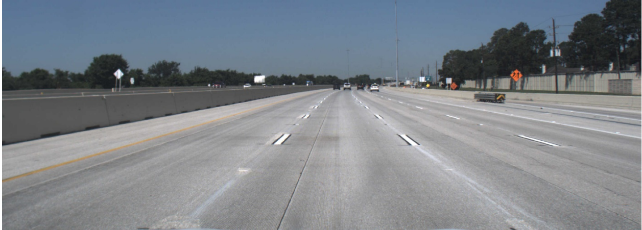
Figure 21: Image of a road segment with white pavement markings with a black border (driving westwards).
