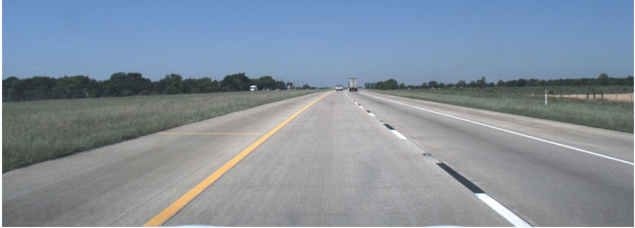
Figure 18: Image of a road segment with white pavement marking followed by black (driving westwards).
