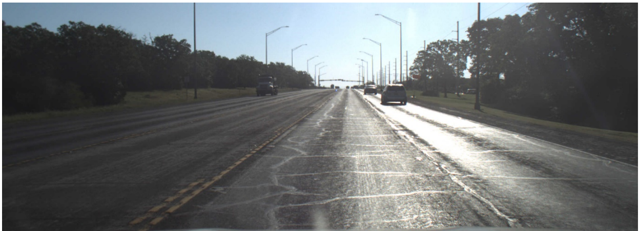
Figure 22: Image of a road segment with white pavement markings, and significant sun glare (driving eastwards).
