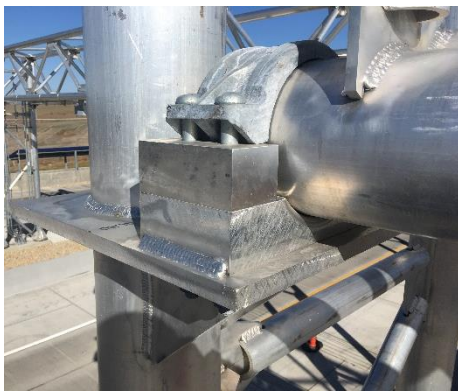
(a) Connection for Bottom Chord
