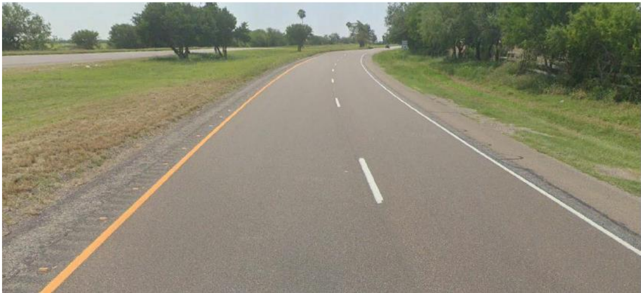
Figure 5. Pharr District US 281 Corridor in Street View (Source: © 2020 Google Earth).
