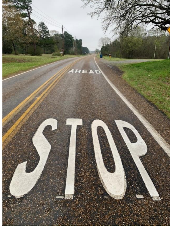
b. STOP AHEAD Pavement Markings.
