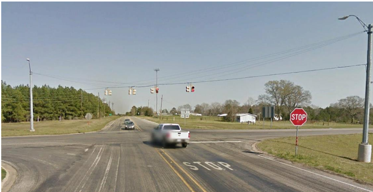
Figure 28. Minor-Street Approach before ICWS (Source: © 2020 Google Earth).
