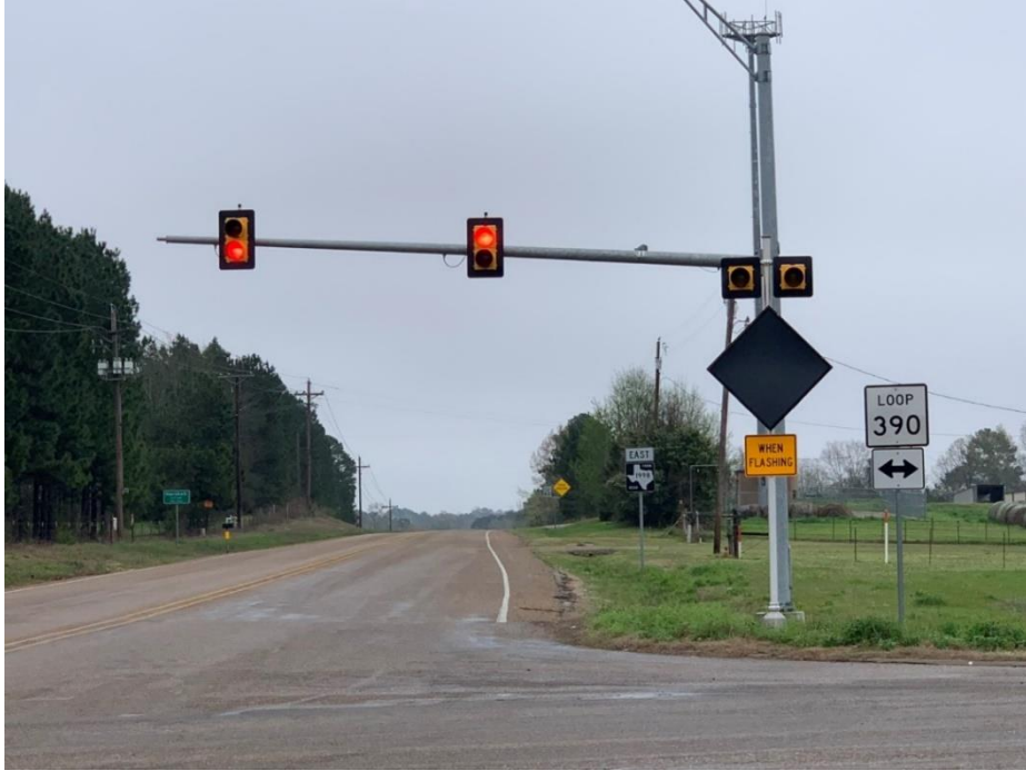
Figure 34. Example of a Warning Sign Assembly on the Minor Street (System Not Activated).
