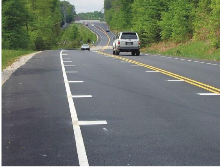
Figure 17. Texas MUTCD–Compliant Optical Speed Bars (22).
