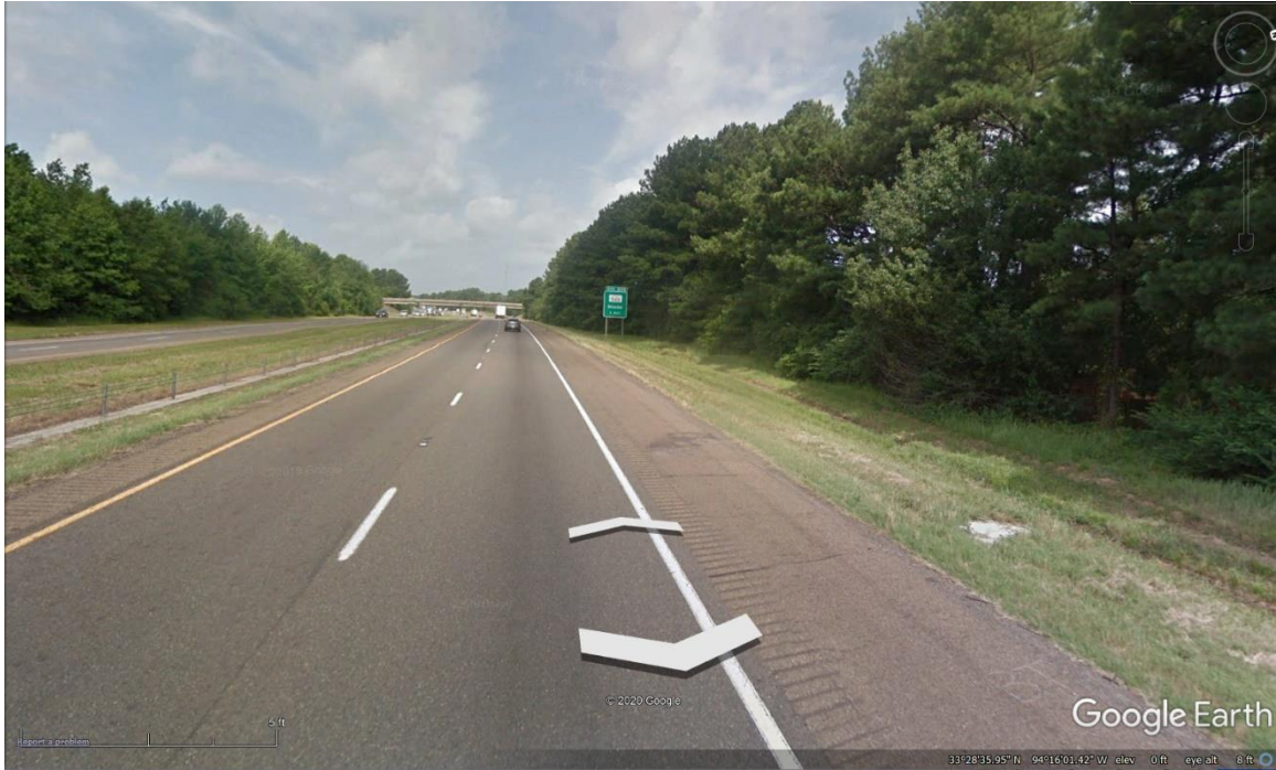
Figure 3. Atlanta District I-30 Curve in Street View (Source: © 2020 Google Earth).
