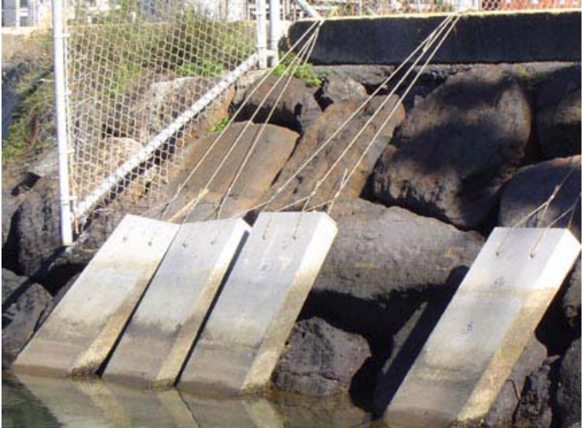
Figure 3.4. Panels hanging along Pier 38 rip-rap.
