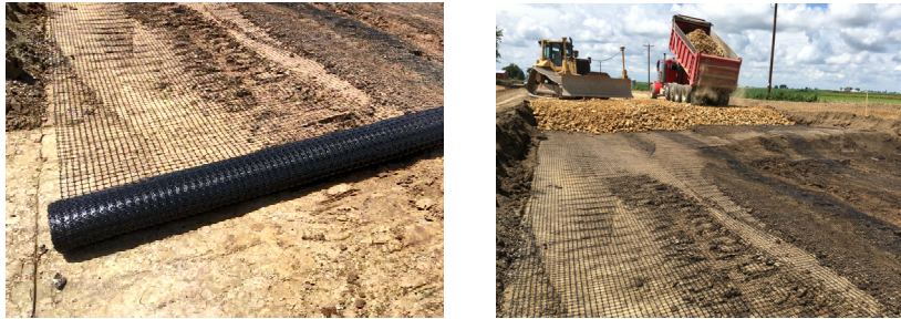
Figure 4.6: Use of biaxial geogrid for subgrade improvement/stabilization and base reinforcement in Wisconsin (Pictures by Titi, 2016).
