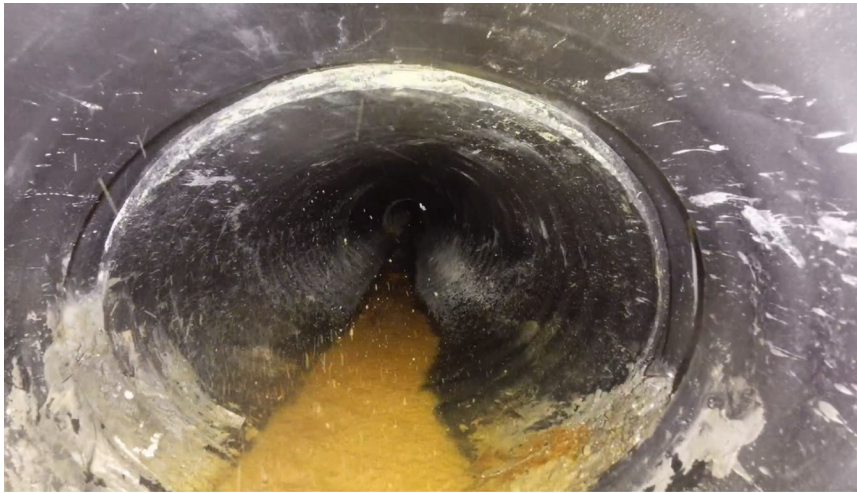
Figure 10. Imagery from the Elios 2 inside Pipe 1.
