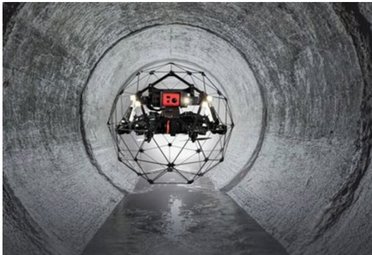
Figure 1. Flyability Elios 2 UAS conducting culvert inspection.
