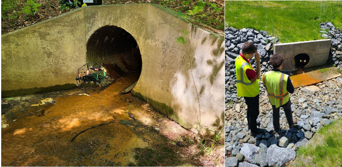
Figure 8 (Left). Elios 2 being flown into Pipe 3.
