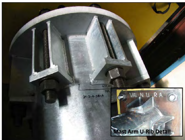
Figure 1.2: U Rib Stiffener and Stool Base Details
