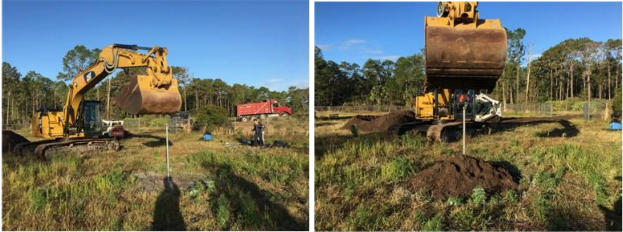
Figure 3-12. Equipment used in the conical load tests
