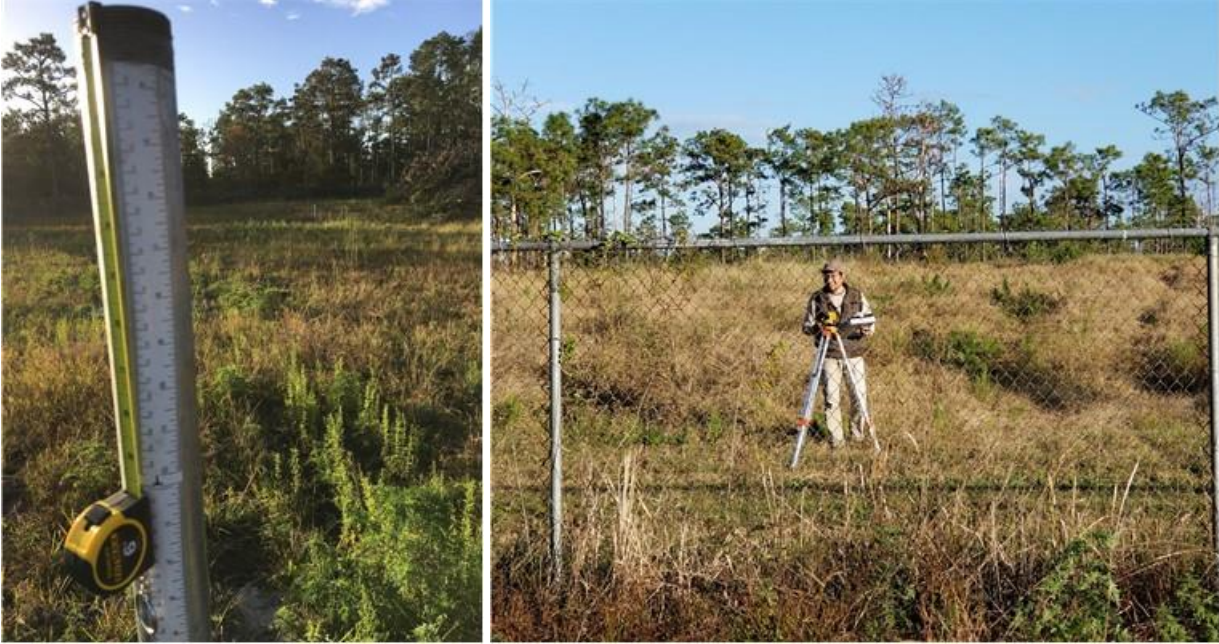
Figure 3-14. Topographic survey equipment to control settlement of riser pipes
