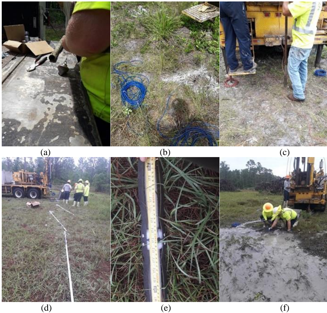
Figure 3-6. (a) Sacrificial tip used for piezometer installation, (b) piezometers at Cone 2, (c) piezometers in place, (d) installation of magnetic extensometers at Cone 3, (e) magnetic extensometer preparation, (f) use of water to avoid buoyancy at Cone 3. Pictures taken on April 8-10, 2019
