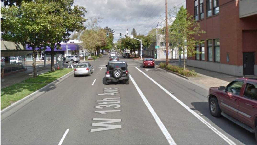
Figure 1.3: The view approaching the first signal on the corridor. The bike lane is on the right.
