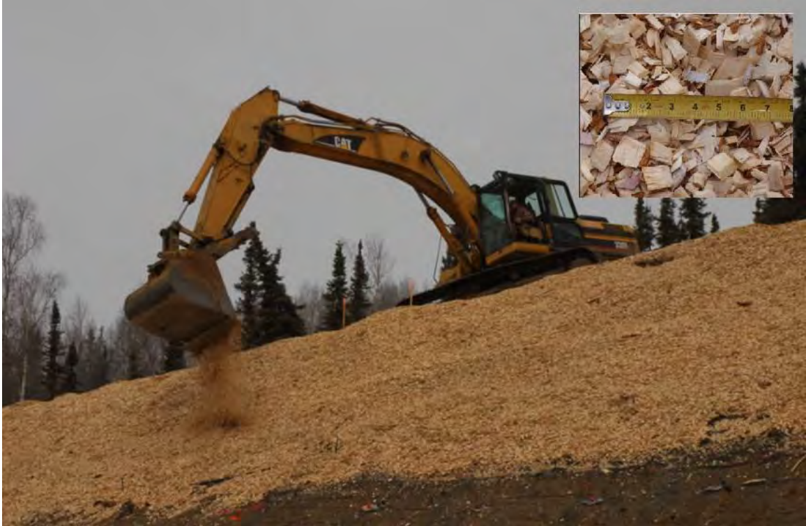
Figure 4.25 Spreading wood chips along top portion of cut slope
