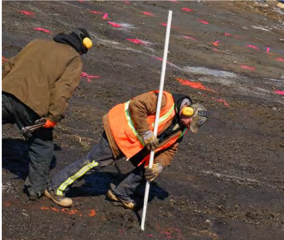
Figure 4.5 Installation for sensor housing
