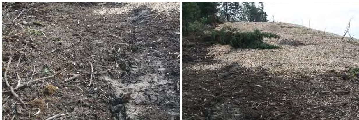
Figure 6.9 Start of thaw related damage at top of Experimental Feature cut slope
