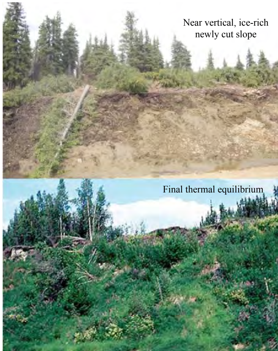
Figure 2.1 Ice-rich cut slope (Mageau and Rooney, 1984)
