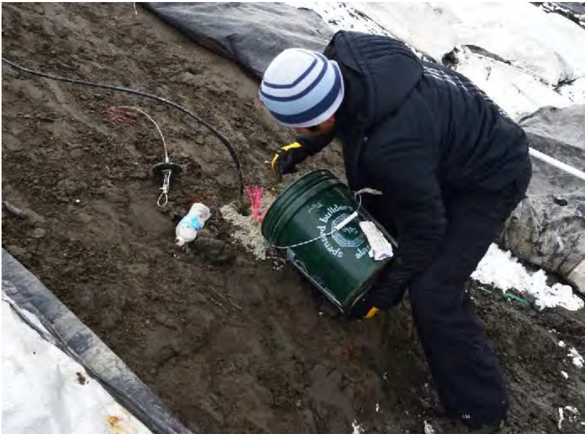
Figure 5.1 Backfilling with sand after insertion of temperature sensor string
