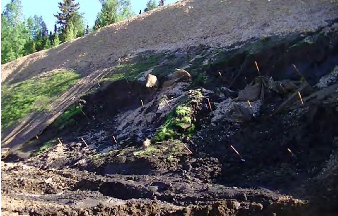
Figure 6.5 Section C without Tecco-mesh and coconut blanket
