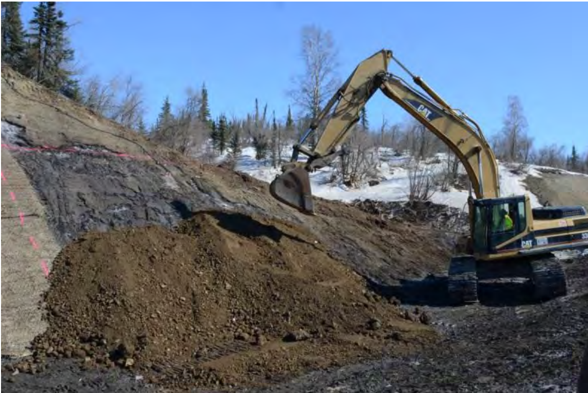
Figure 4.24 Construction of Section D
