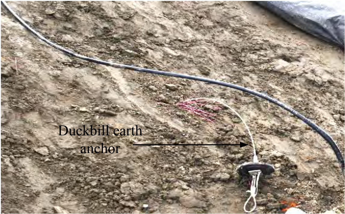
Figure 4.11 Cable end of installed Duckbill earth anchor
