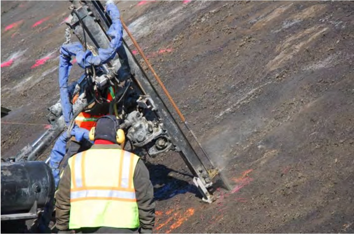
Figure 4.3 Drilling on the cut slope
