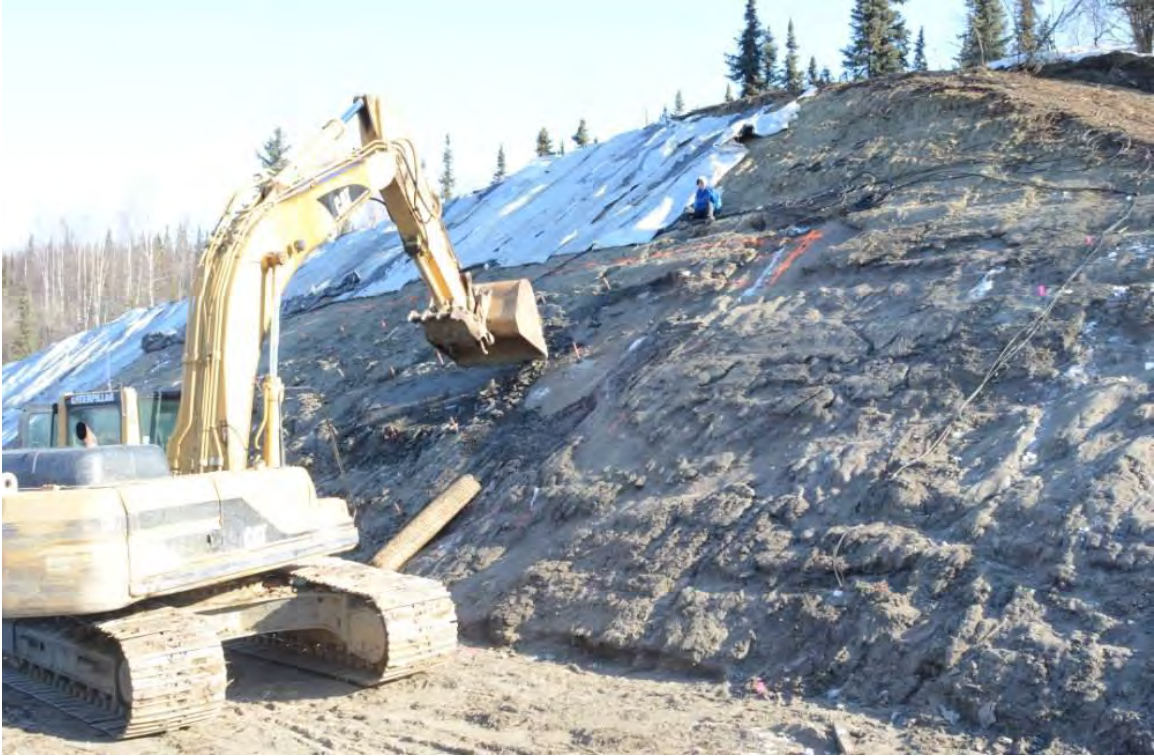
Figure 4.13 Re-smoothing the cut slope surface
