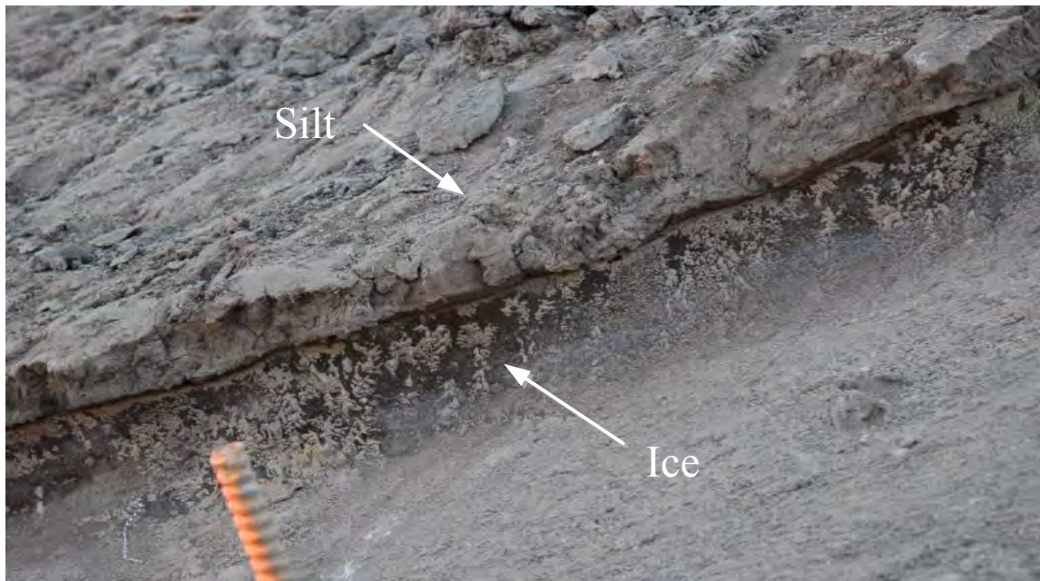
Figure 4.8 Ice in the cut slope
