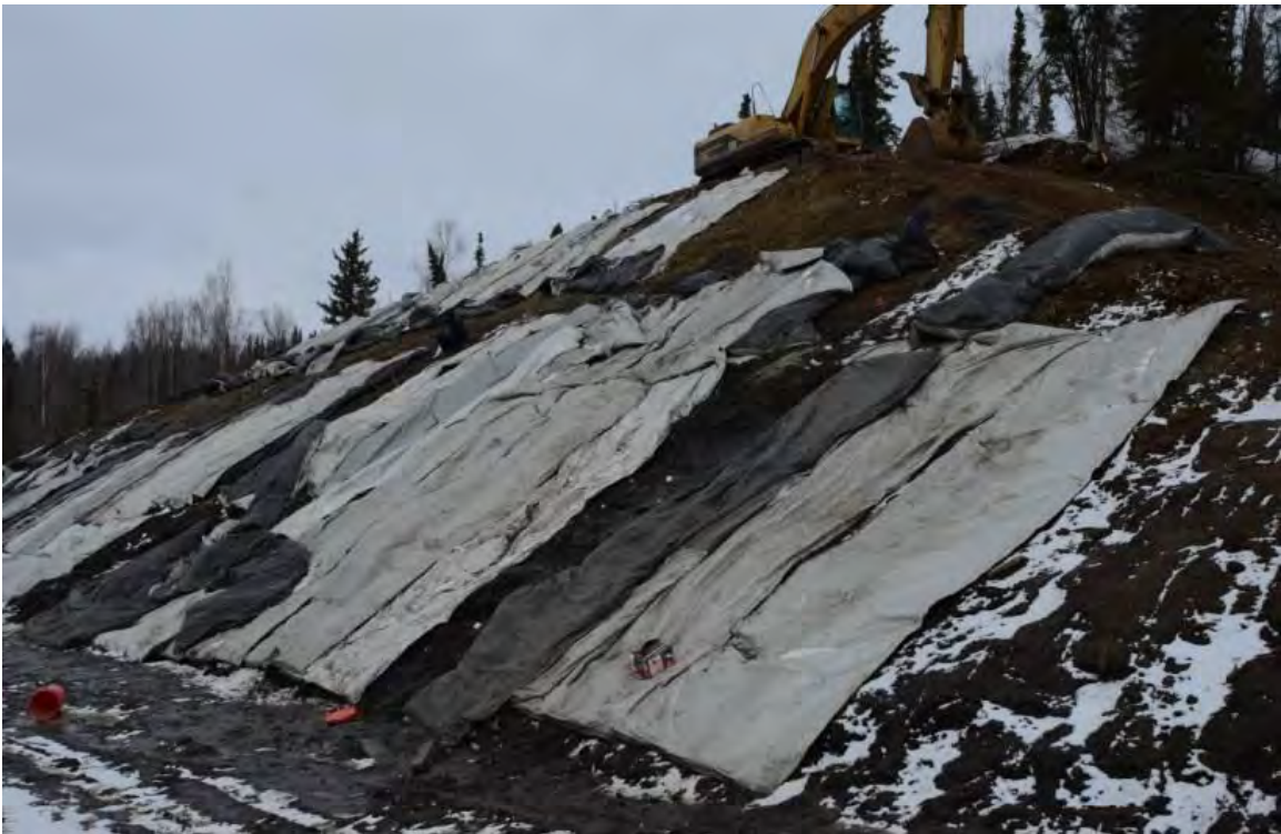
Figure 4.10 Cut slope protected from erosion during drilling
