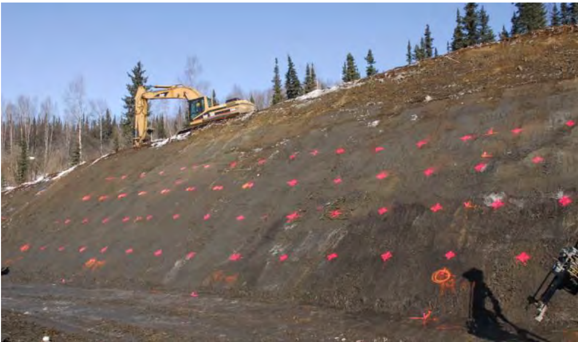
Figure 4.2 Layout on the cut slope
