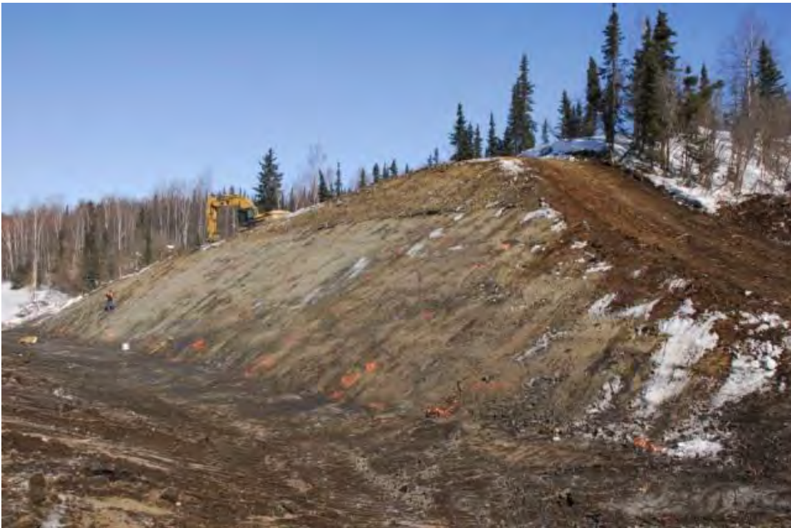
Figure 4.1 Cut slope at Dalton Highway 9-mile construction project location
