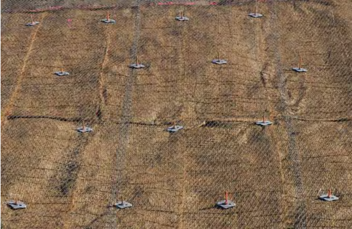
Figure 4.22 Section C appearance after construction
