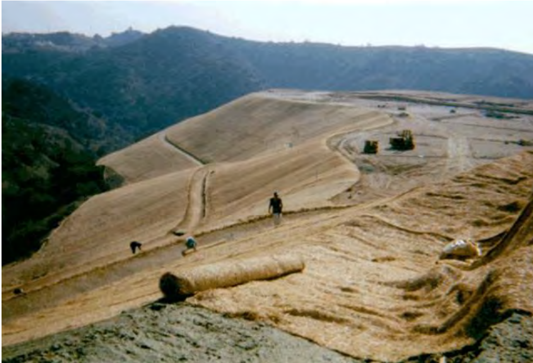
Figure 2.4 Erosion control blanket (from http://www.thelandstewards.com/blankets.htm )
