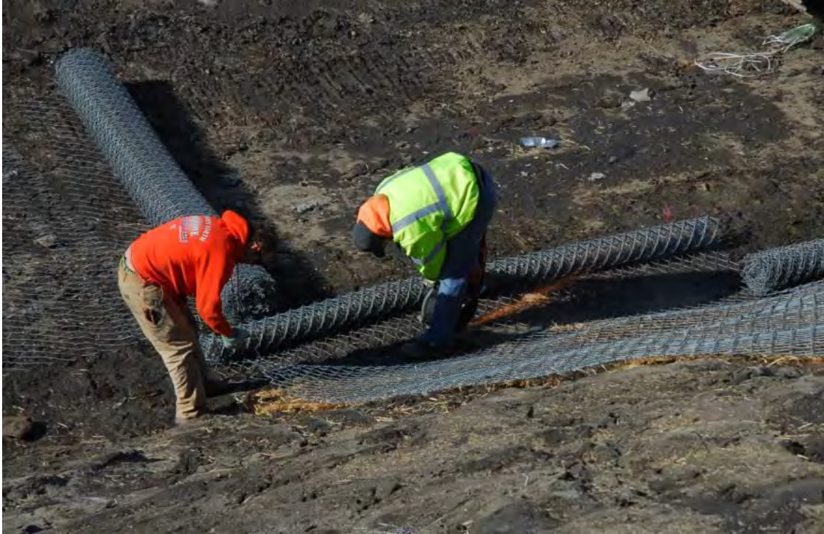
Figure 4.20 Cutting away excess Tecco-mesh
