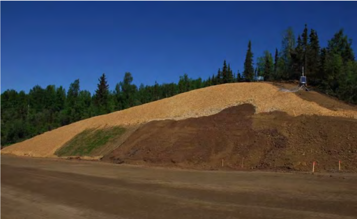
Figure 6.8 Cut slope after construction on Section C
