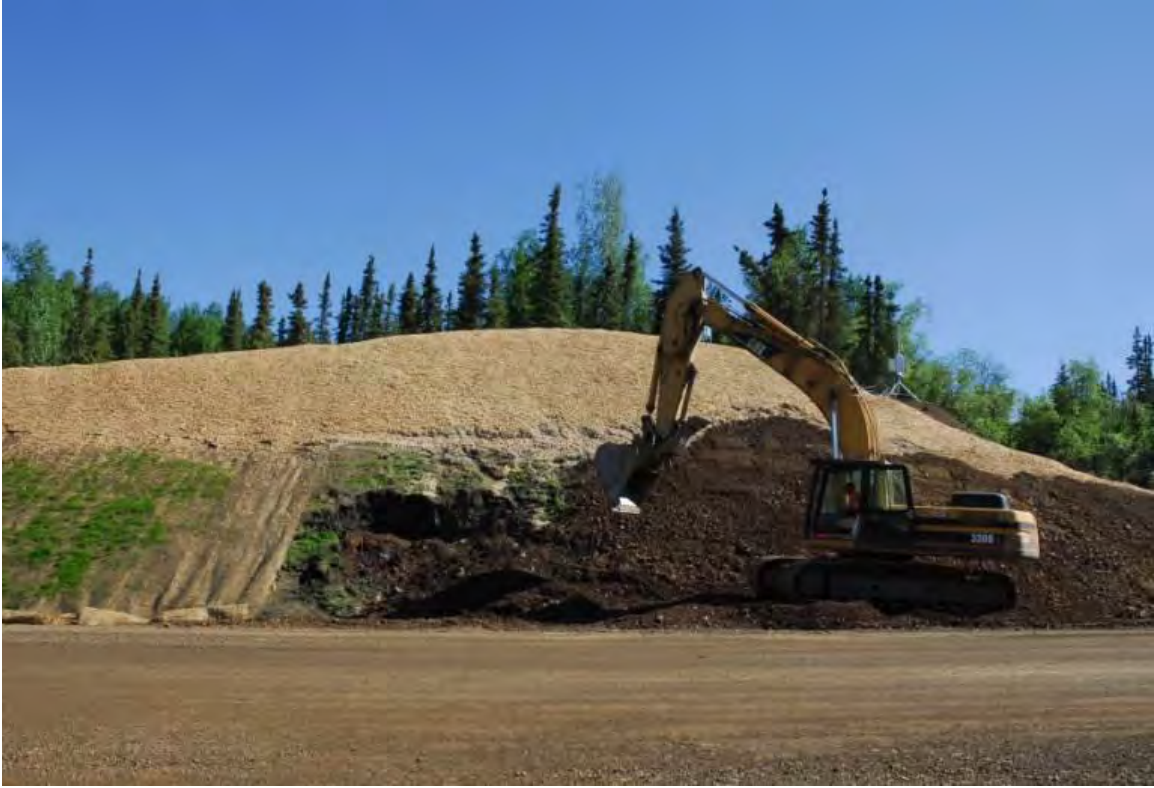
Figure 6.7 Covering Section C with crushed rock
