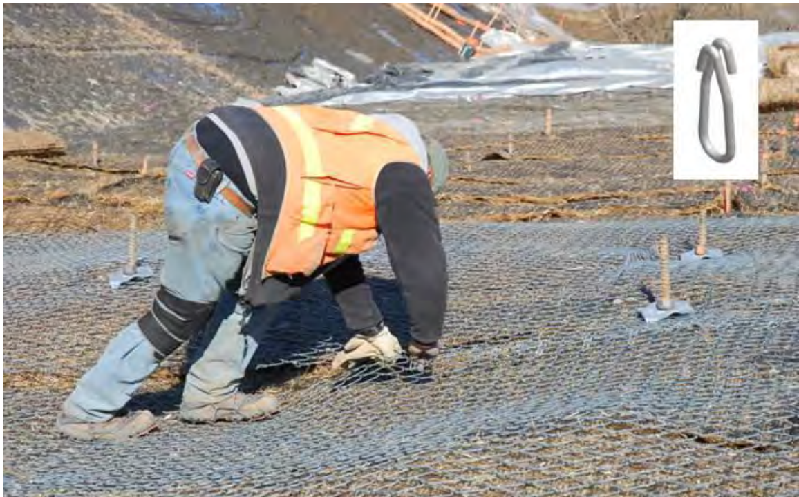
Figure 4.21 Connecting adjacent Tecco-mesh strips
