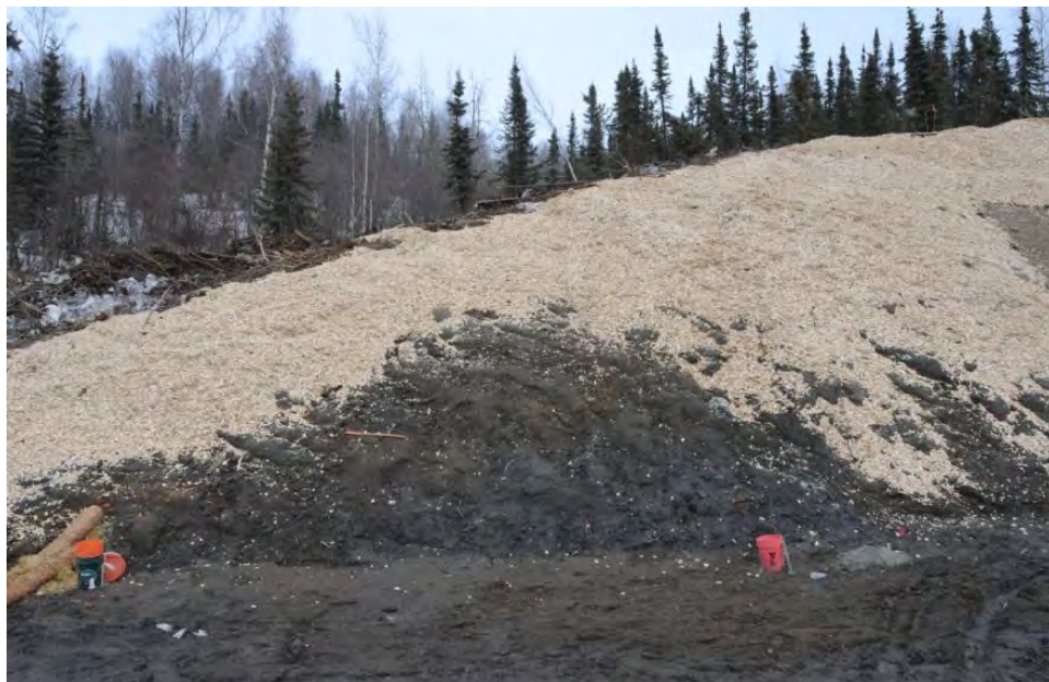
Figure 7.23 Section A after construction on April 26 th , 2013
