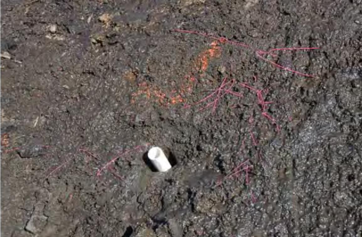
Figure 4.6 Instrumentation hole with sensor housing installed
