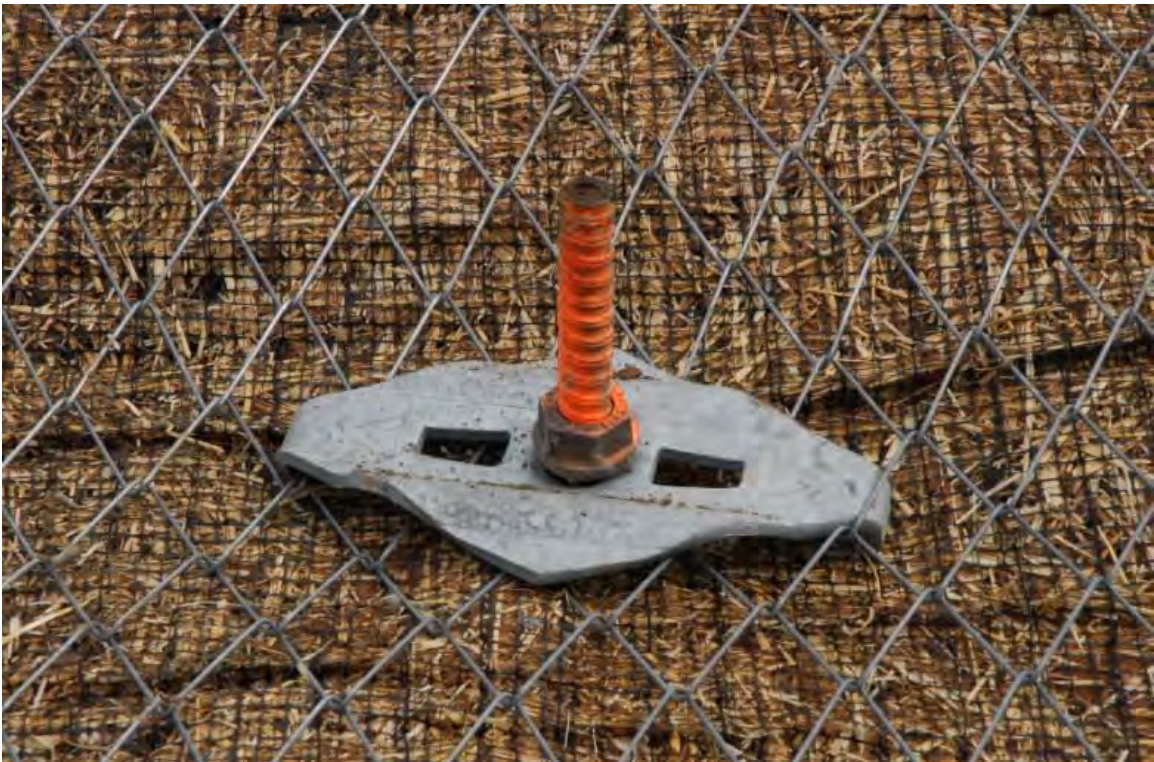
Figure 4.23 Close-up view of Tecco-mesh at an anchoring point
