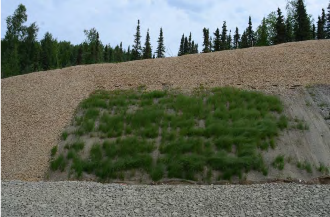
Figure A.3 Typical image captured for erosion monitoring
