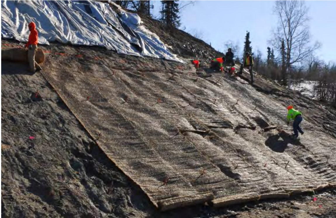
Figure 4.16 Placement of coconut erosion control matting
