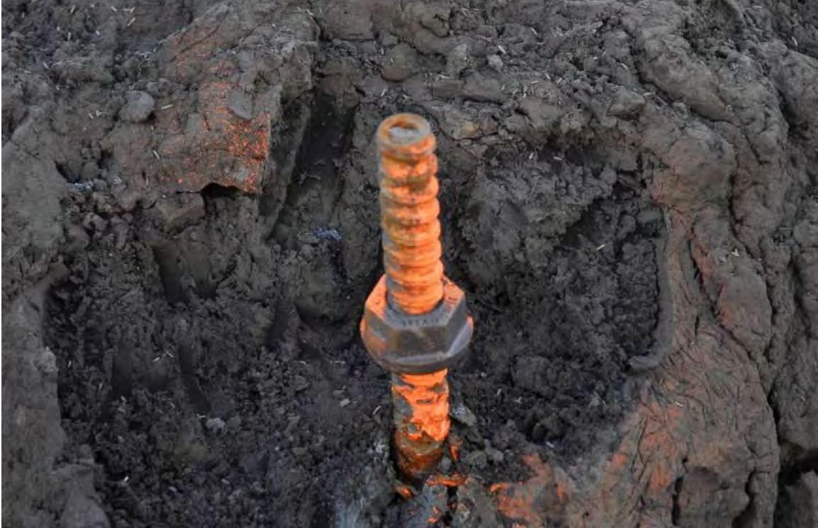
Figure 4.12 Installation of hollow rebar anchor
