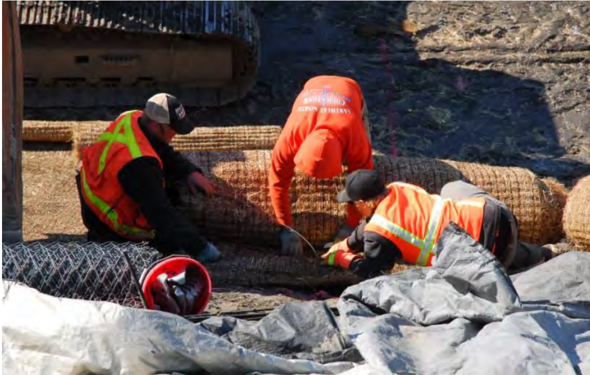
Figure 4.15 Placement of coconut erosion control matting
