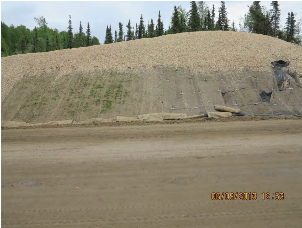
Figure 6.4 Surface protection matting in areas showing no grass growth are not in direct contact with ground surface
