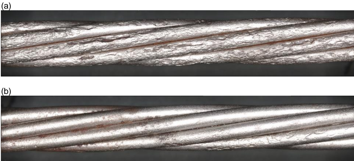
Figure 5-12: Steel strands after corrosion product removal extracted from 3-ft tendons: (a) not impregnated; (b) impregnated.
