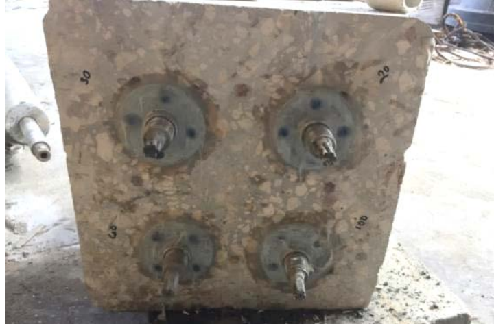
Figure 4-9: Removal of PVC fittings leaving grouted strands exposed.
