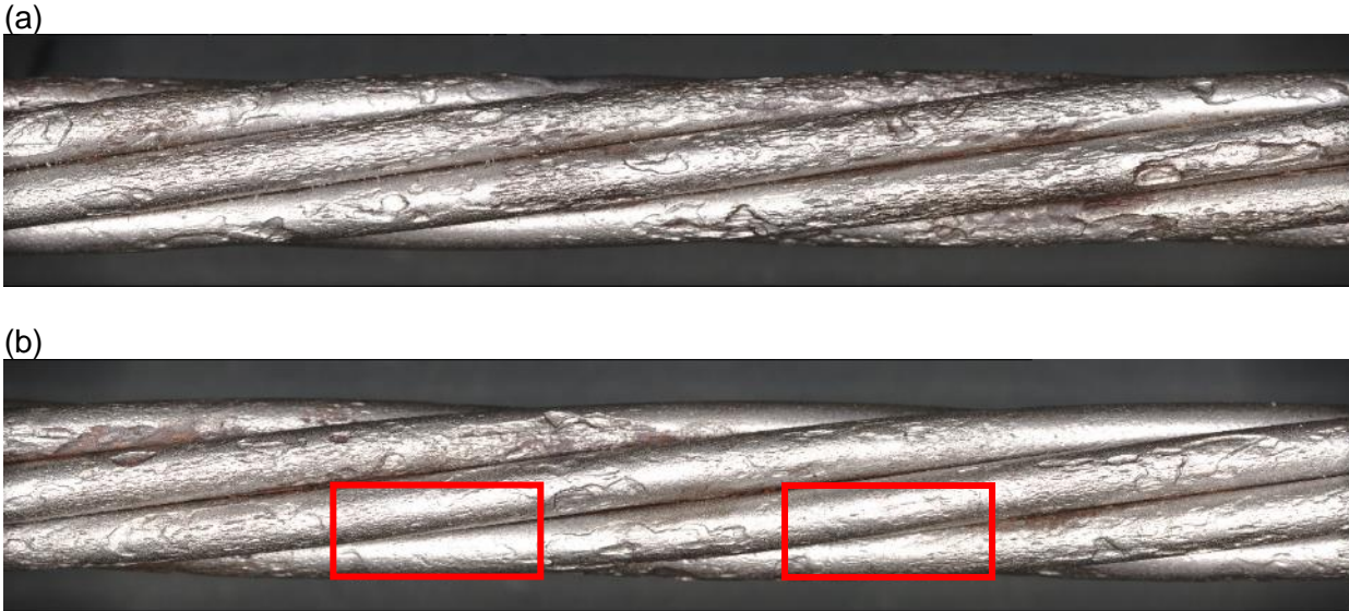
Figure 5-11: Steel strands after corrosion product removal extracted from 1-ft tendons: (a) not impregnated; (b) impregnated.
