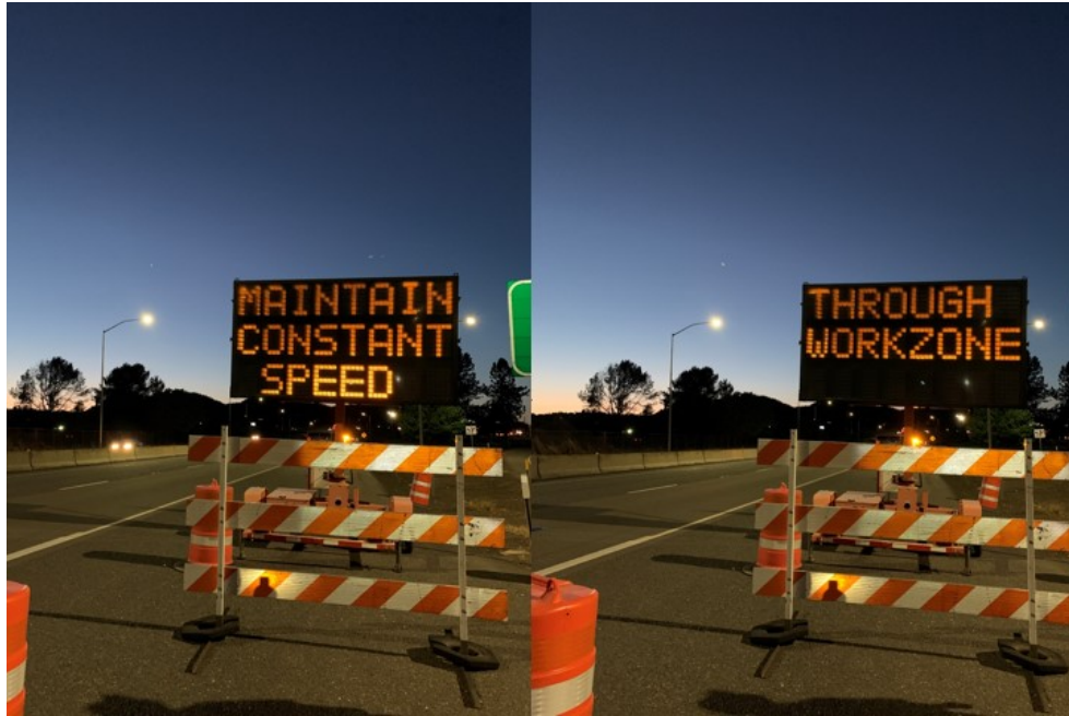
Figure 5.24: PCMS used in case study #3 showing custom messages: “MAINTAIN CONSTANT SPEED” (left) and “THROUGH WORKZONE” (right)
