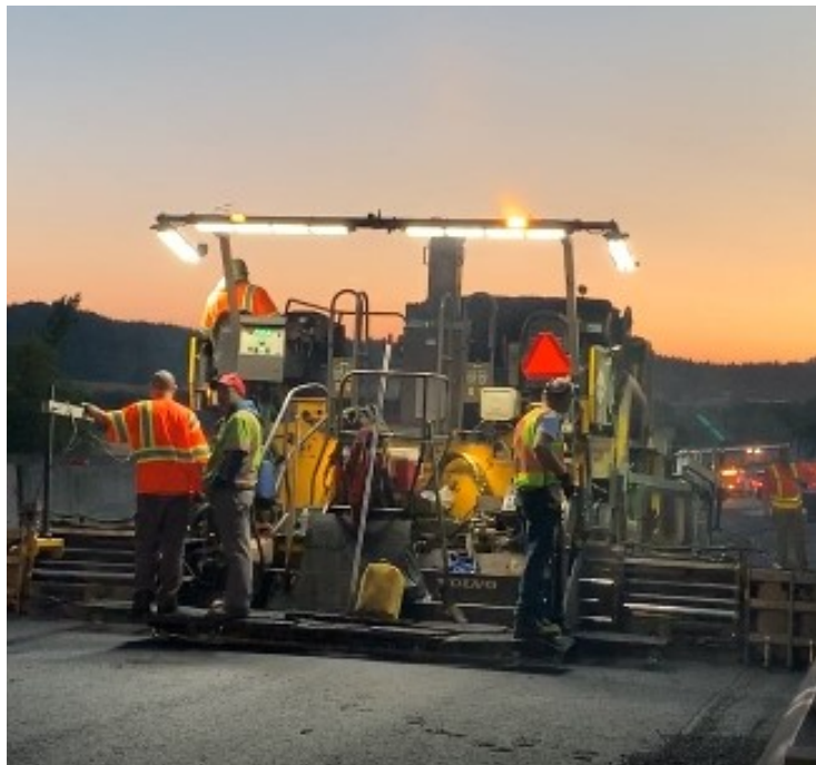
Figure 5.25: Paver with flashing amber/white lights on (case study #3)
