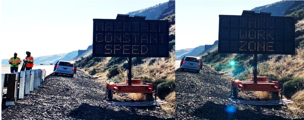
Figure 5.13: PCMS used in case study #1 showing custom messages: “MAINTAIN CONSTANT SPEED” (left) and “THRU WORK ZONE” (right)
