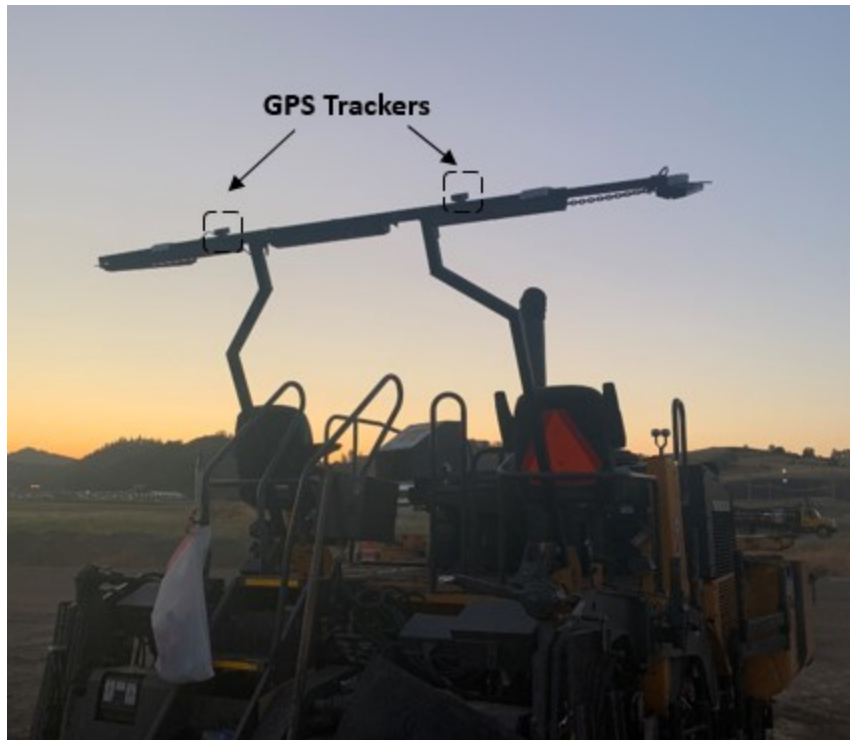
Figure 5.8: GPS trackers placed on a paver
