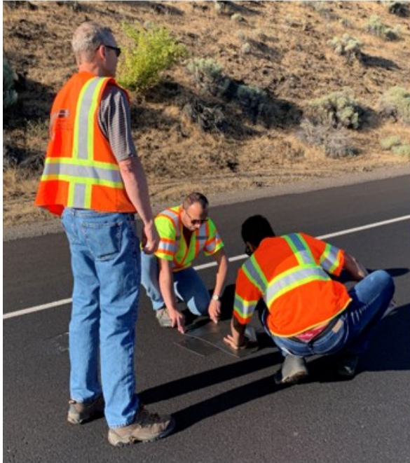
a). Sensor Installation
