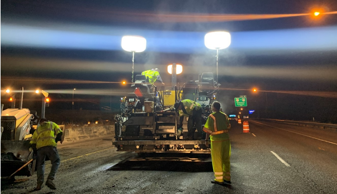
Figure 5.17: Paver performing work on the site (case study #2)
