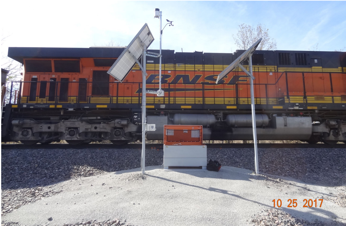
Figure 29. Typical Setup of Instrumentation Box, Solar Panels, and Weather Station
