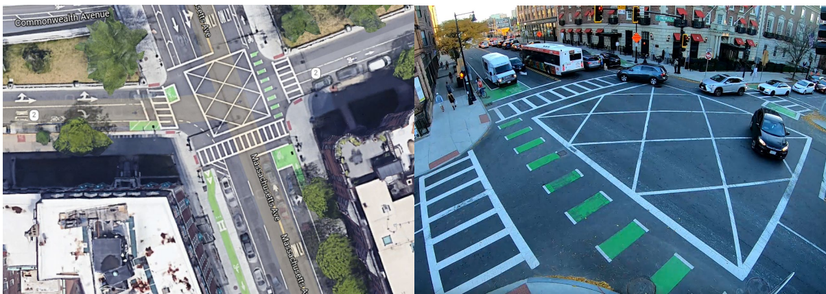
Figure 2.12: Intersection layout and camera view for Massachusetts Ave. at Commonwealth Ave.
