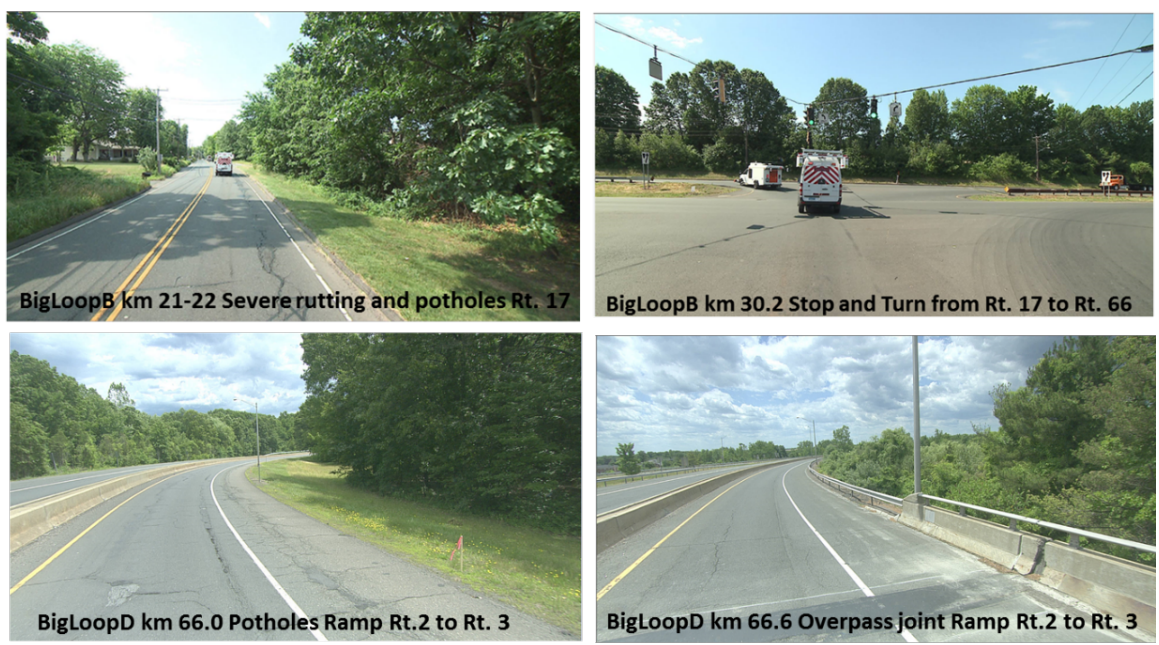
Figure 5.8 Roadware Vision ROW images of sections with extreme IRI values.
