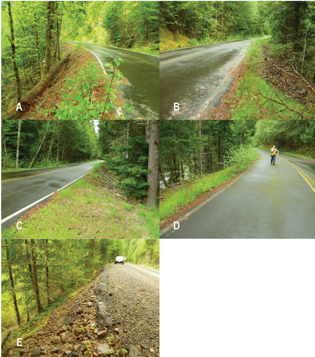
Figure 27: Photos of deep patch repairs on Road 63, Mount Hood National Forest, at a) Sta. 20+15, b) Sta. 30+35, c) Sta. 80+68, d) Sta. 115+96, and e) Sta. 187+40.
