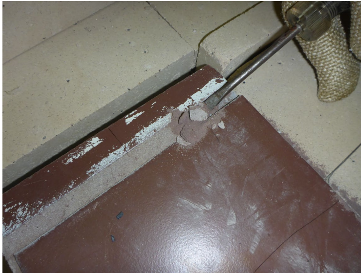
Figure 7.22: Removal of grout with a screwdriver after heating
