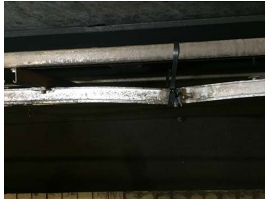
Aluminum wireway damage (Deformation at 450^{\circ}\text{C} (842°F)) (Melts at 600^{\circ}\text{C} (1,112°F))
