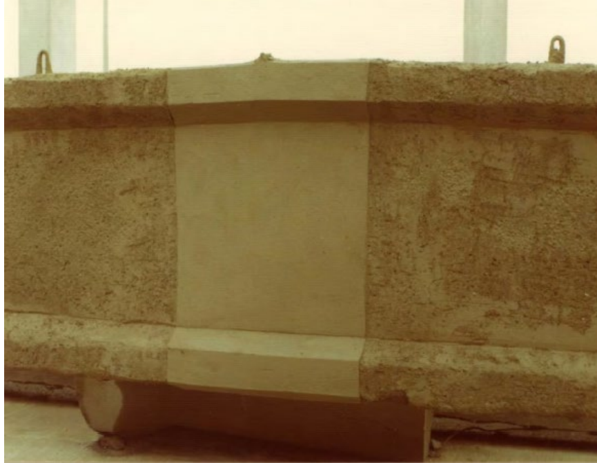
Figure 5.12: Midspan of girder after repair
