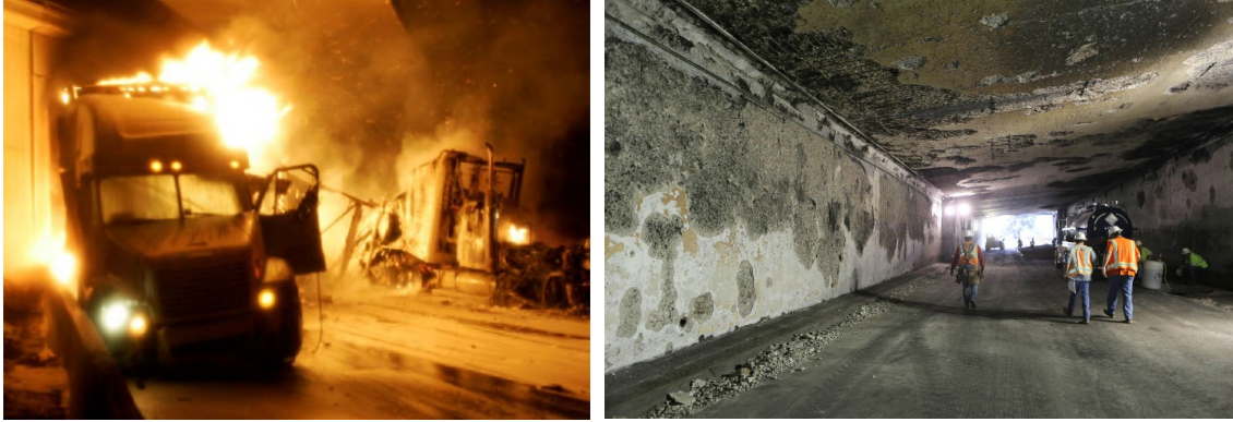
Figure 4.1: Picture taken during Newhall Pass fire event (L); post-fire condition of tunnel (R)
