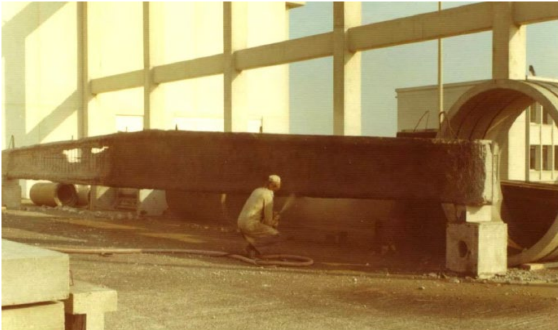
Figure 5.11: Application of shotcrete to damaged girder
