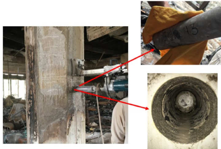
Figure 4.12: Extraction of concrete cores for compressive strength tests
