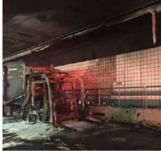
Wall tiles & lights (Temp. \geq 450^{\circ}\text{C} (842°F))
