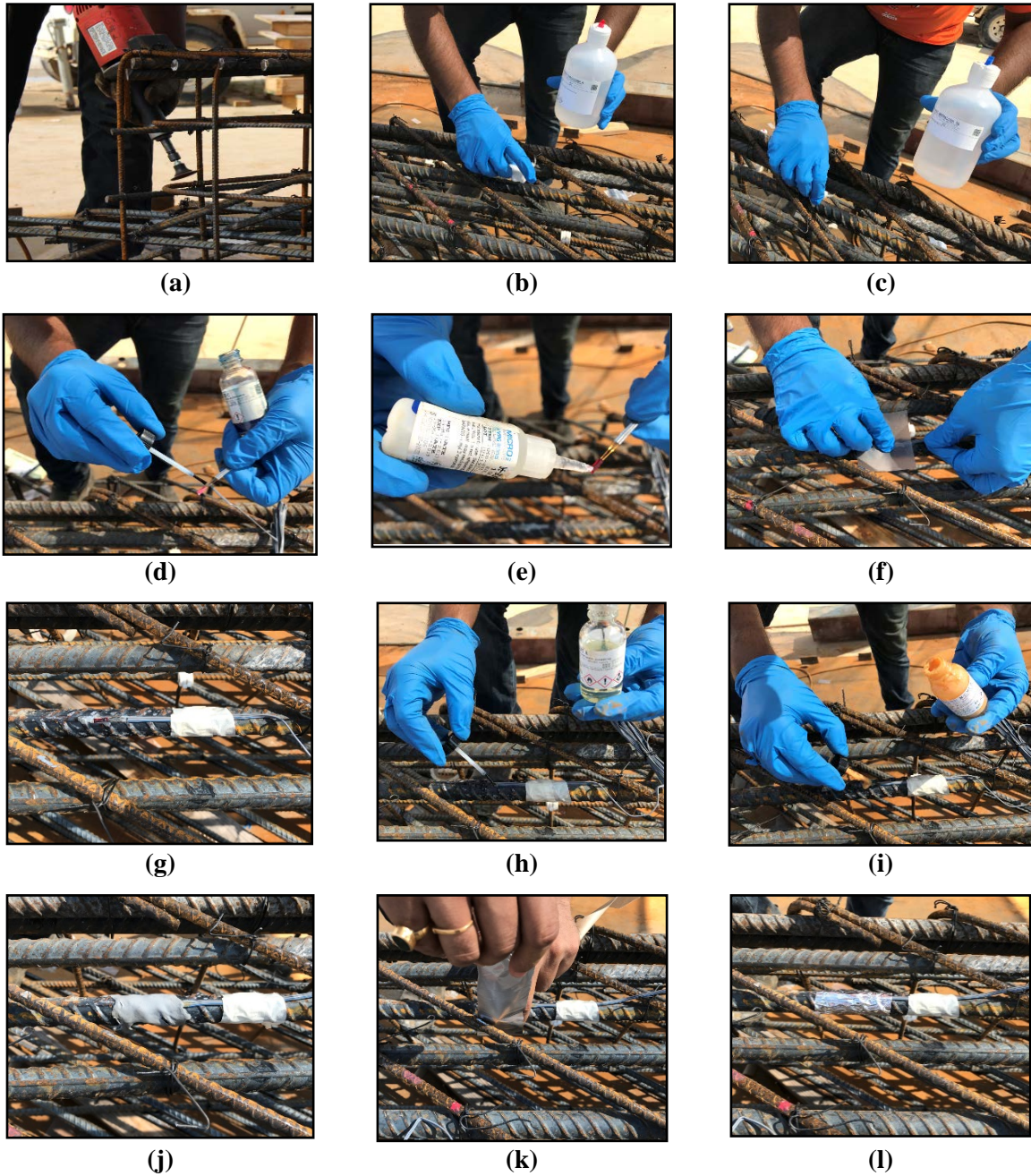
Figure 3.14. Strain Gauge Installation:
