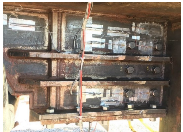
Figure 8. Exterior view of the shear bolts installed through the draft pocket
