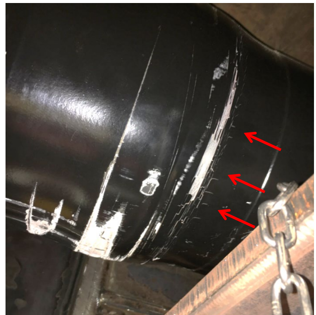
Figure 2. Cracked paint on the left side of the PBC deformation tube indicating tube crush
