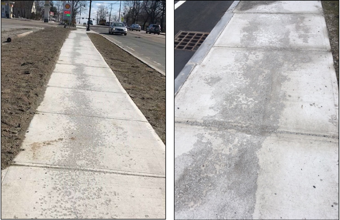
Figure 1.1: Examples of scaling degradation on Contract 90474, Medway (left), and Contract 101985, Fitchburg-Leominster-Lunenburg (right)
