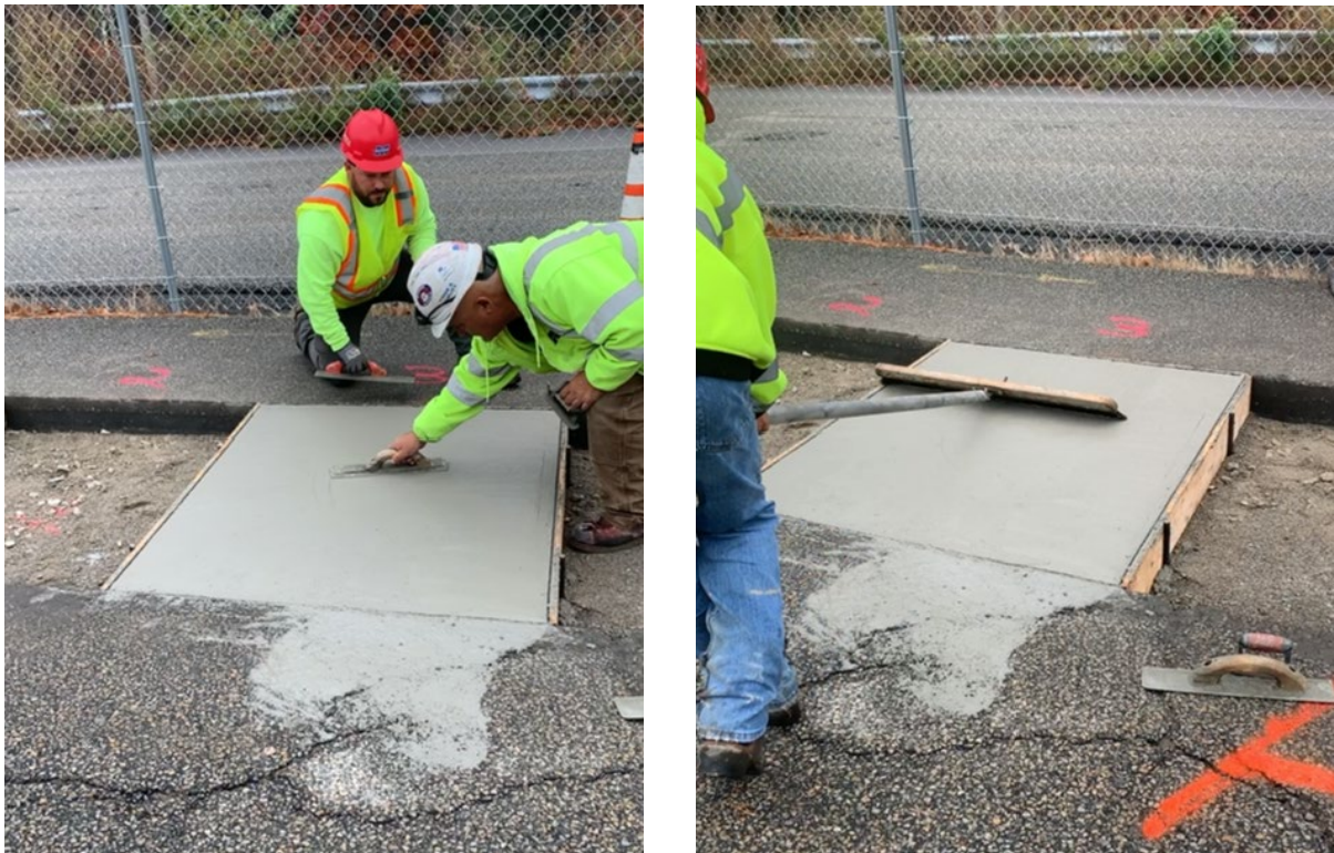
Figure 5.4: Best practices panels—magnesium float (left) and broom (right)
