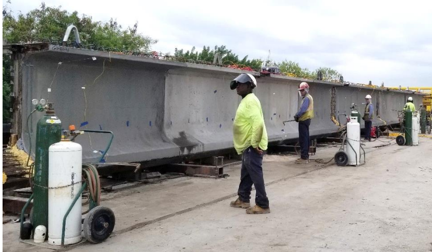
Figure 3-18 Construction crew in position for detensioning
