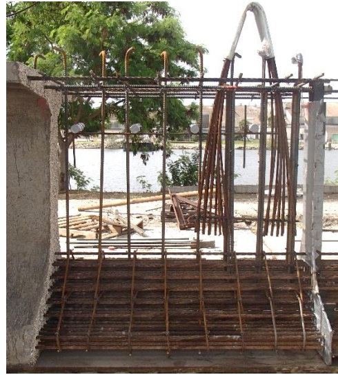
Figure 4-8 Installation of mild-steel reinforcement on UHPC section of the girder
