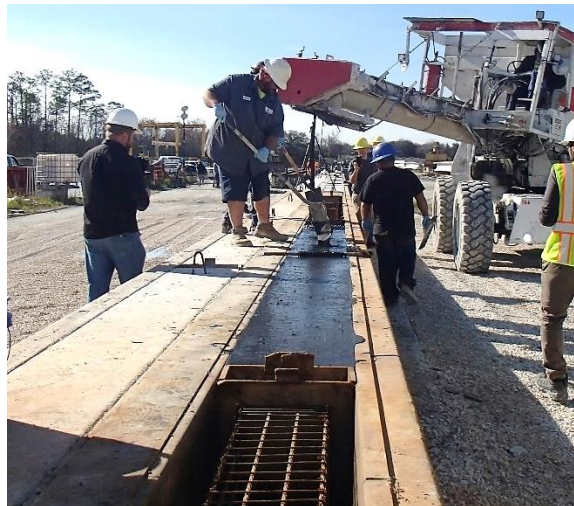
Figure 2-3 Precast piles made of UHPC
