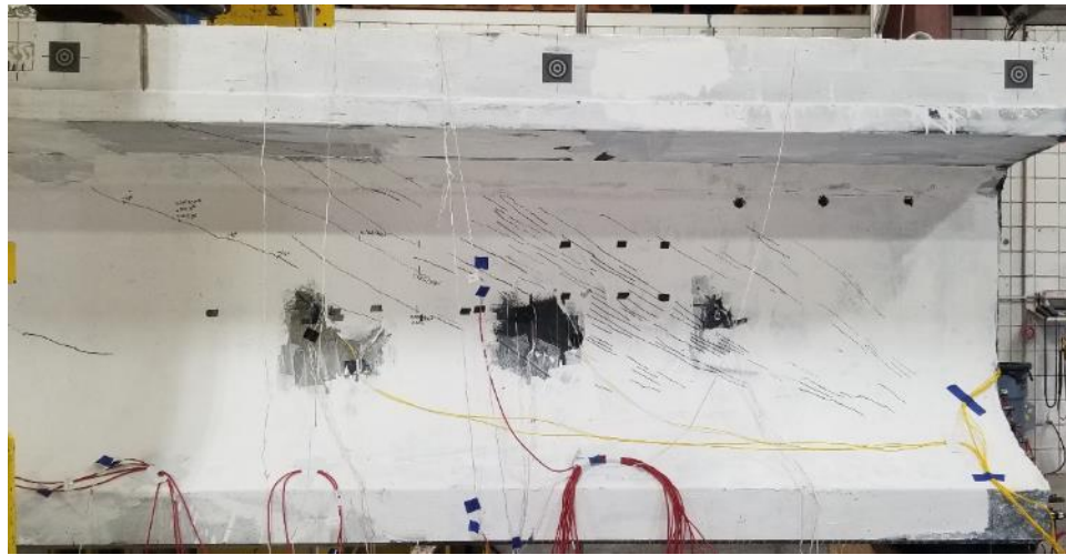
Figure 4-57 Cracking of G7-E2
