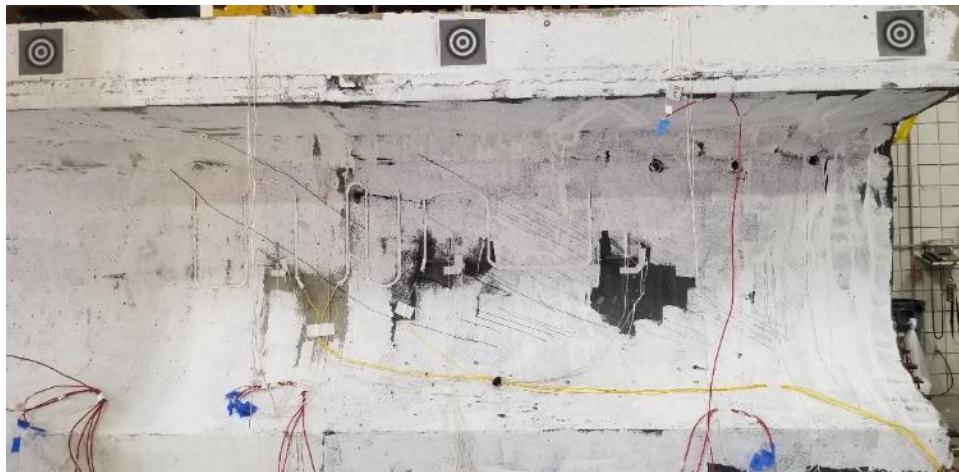
Figure 4-39 Cracking of G6-E2
