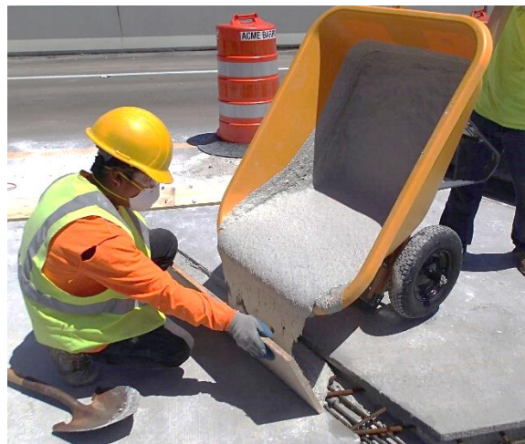
Figure 2-1 UHPC used for joints of deck panels
