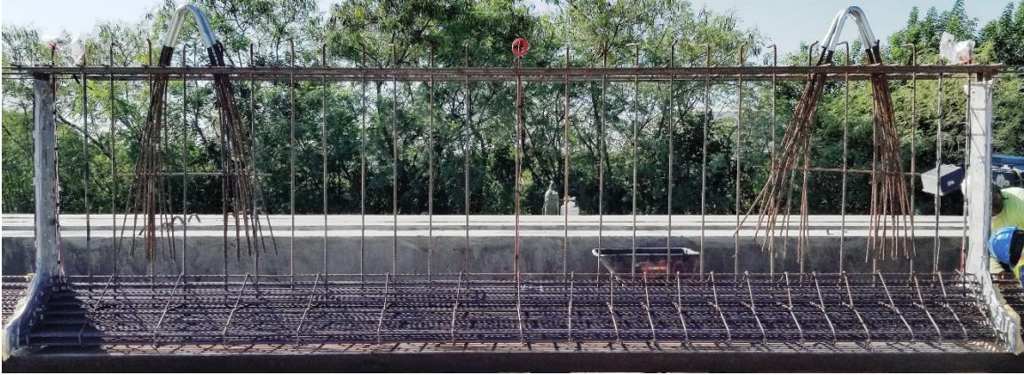
Figure 3-7 Mild-steel reinforcement in G3
