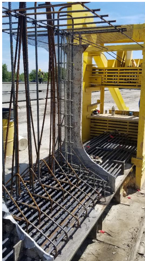
Figure E-3 Polyethylene mesh after installation
