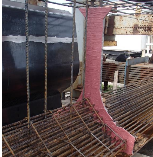
Figure 4-6 Application of concrete retarder on bulkheads
