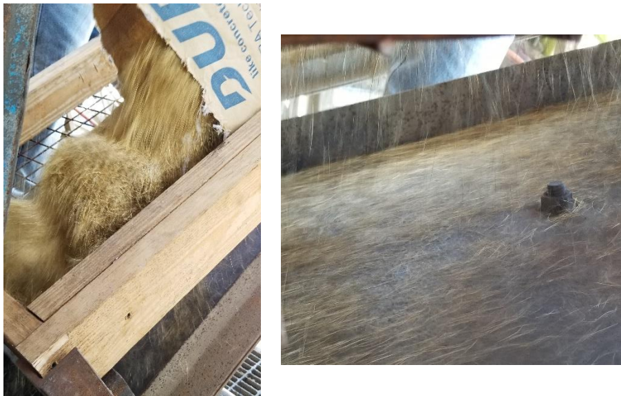
Figure 3-14 Steel fibers added to UHPC through a steel wire mesh
