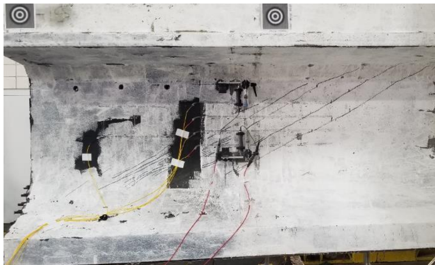
Figure 4-31 Cracking of G6-E1
