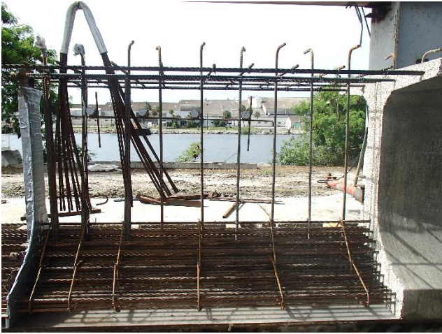
Figure 4-8 Installation of mild-steel reinforcement on UHPC section of the girder
