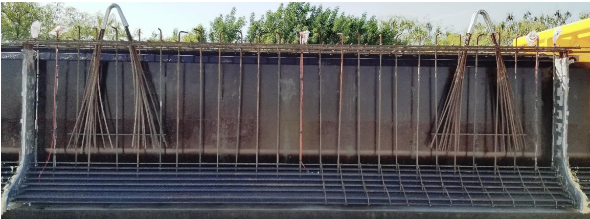
Figure 3-9 Mild-steel reinforcement in G5
