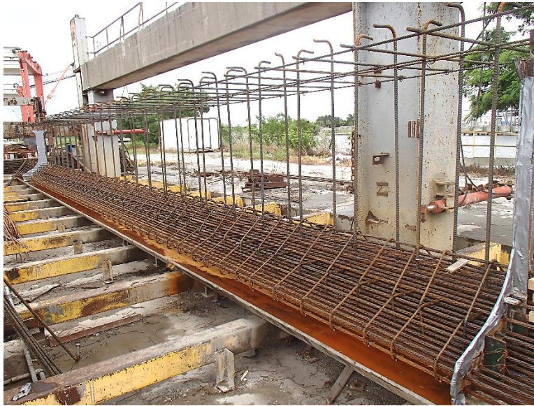
Figure 4-5 Installation of mild-steel reinforcement in SCC section
