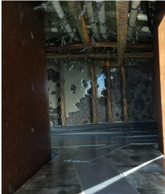
Figure E-4 Material that passed through the mesh after one hour of pour
