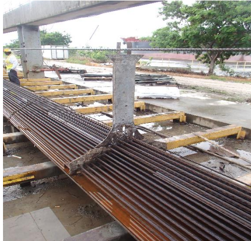
Figure 4-4 Placement of temporary bulkhead
