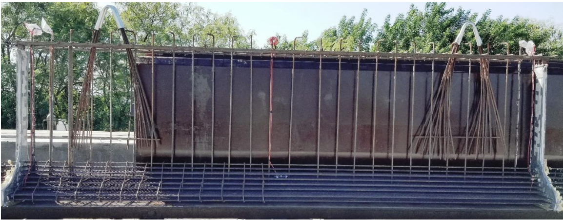
Figure 3-8 Mild-steel reinforcement in G4
