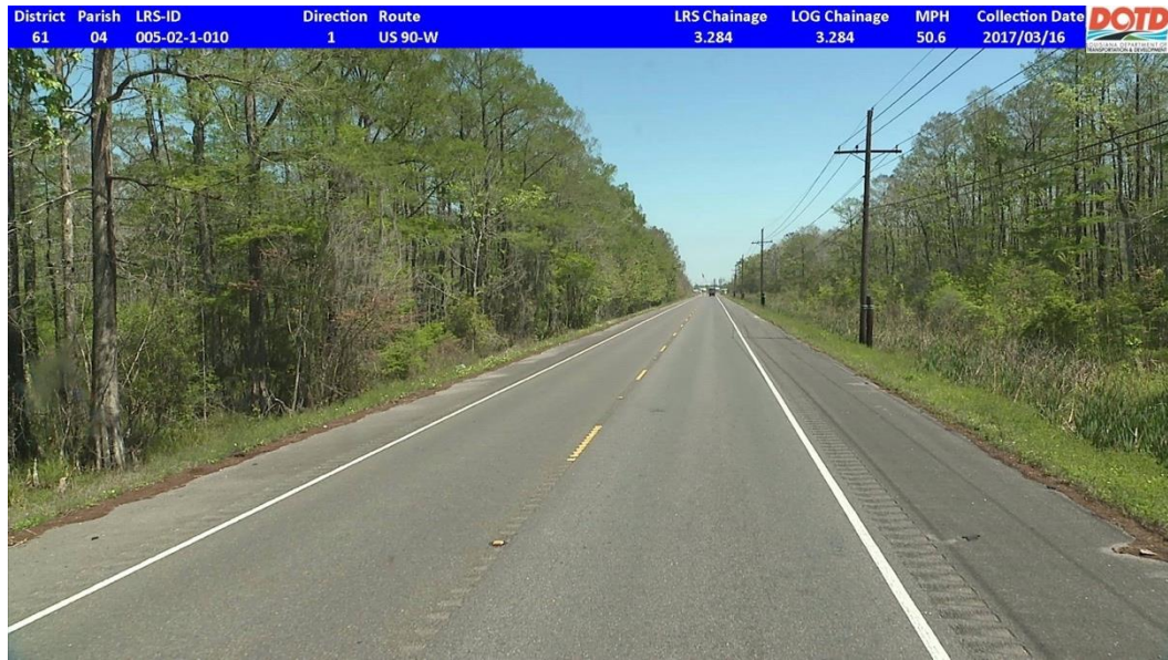
Figure 3. An Illustration of a Two-Lane Section with RS Extracted from “ivisionRoadware”
