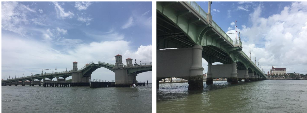
Figure 10.81. Existing main span bascule piers of Bridge of Lions (left); approach spans Pier 14 closest decreasing in number into the distance (per plan numbering).
