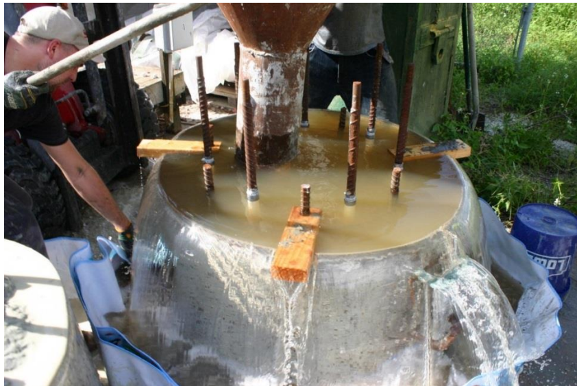
Figure 2.1 Natural slurry (water) exiting the form during concreting.
