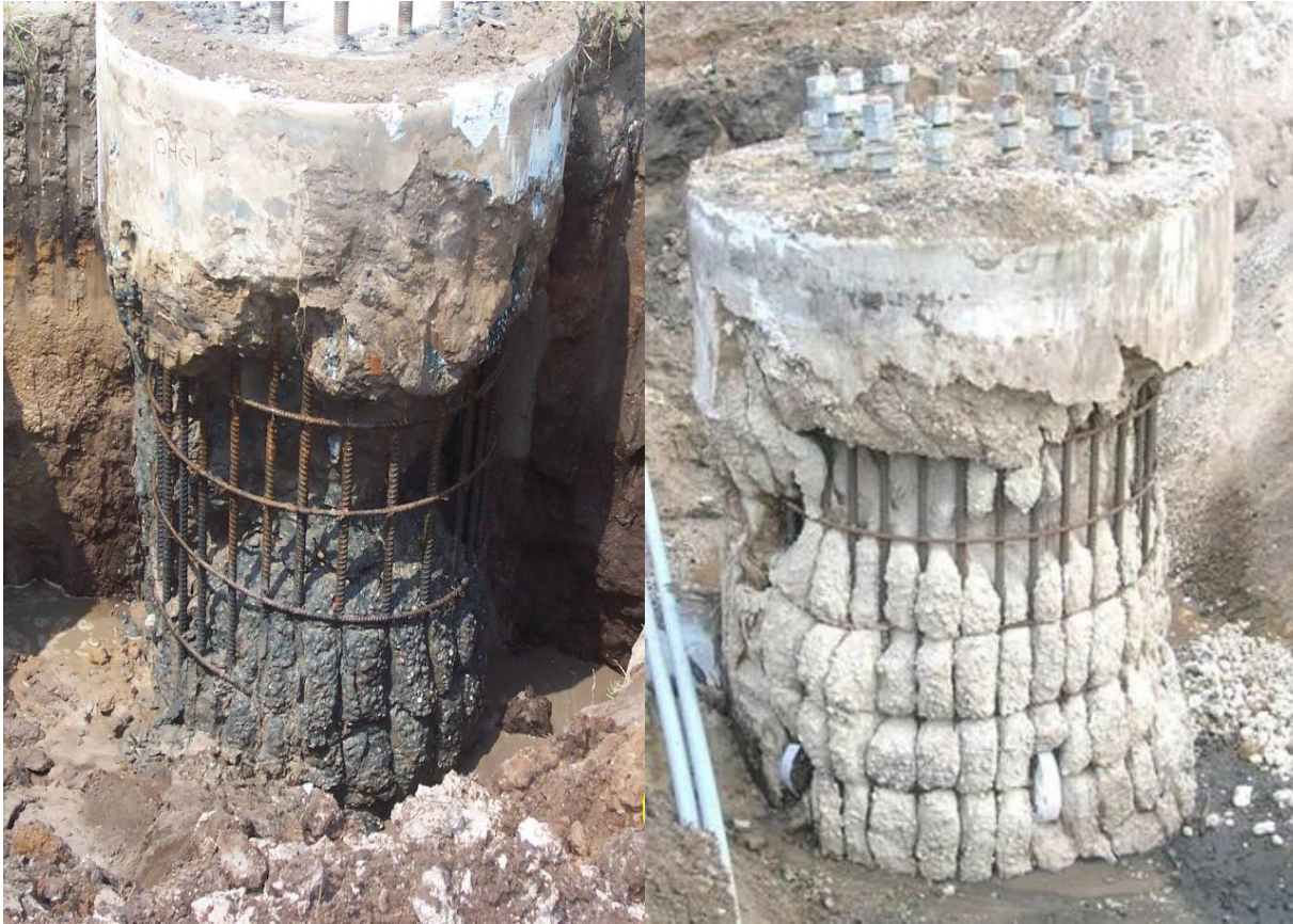
Figure 2.9 Concrete buildup inside the cage that provides lateral pressure to fill the cover.
