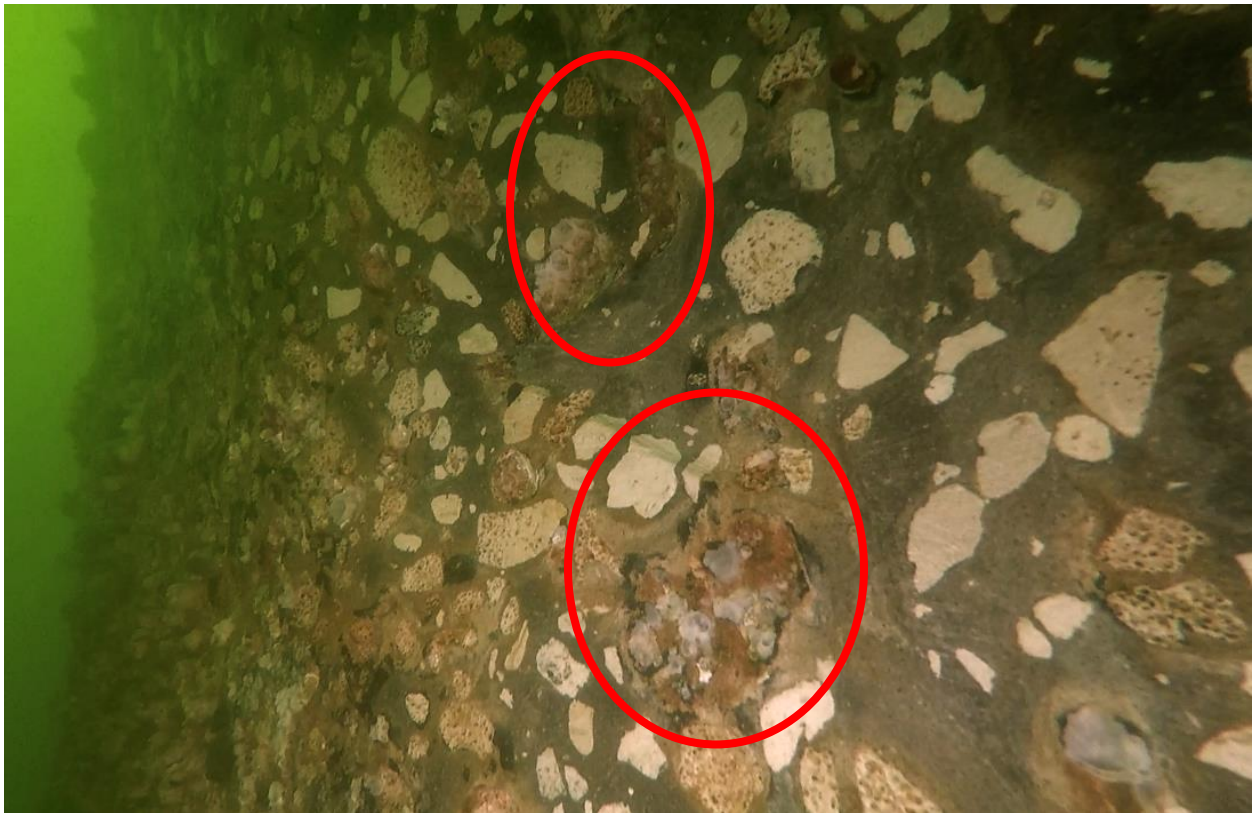
Figure 10.26 Cleaned portion of 84-4 on the southeast side of the shaft, circled sections indicate small voids in concrete filled by barnacles.
