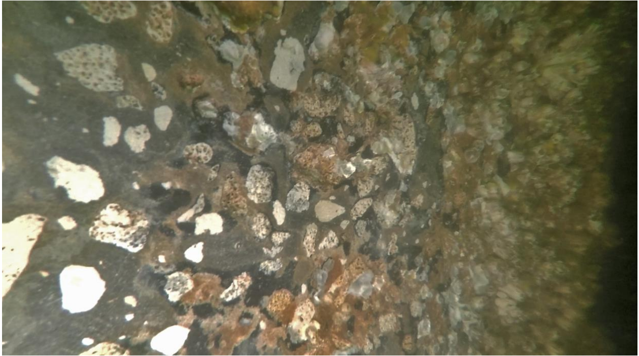
Figure 10.25 Shaft 84-4 partially cleaned, note clean concrete going into layer of barnacles.
