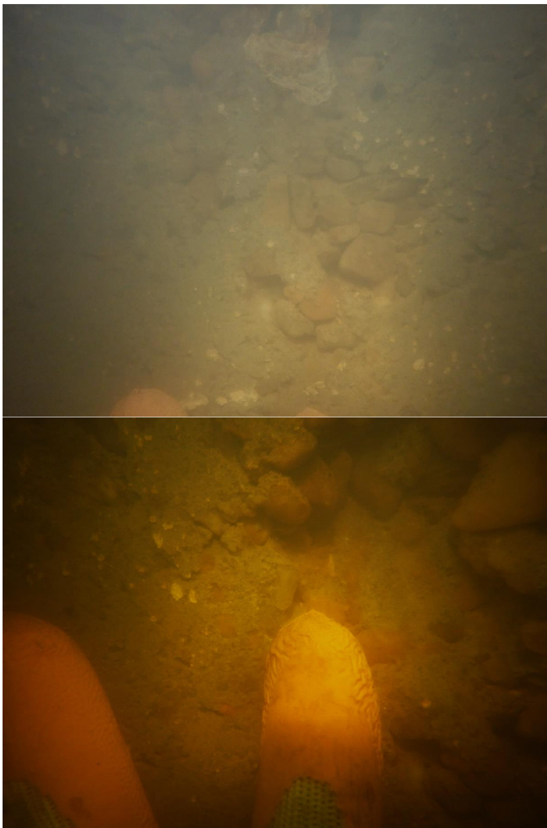
Figure 10.71 Images of Shaft 58-2 with the casing removed from the upper portion of the shaft demonstrating quilting and poor surface quality .
