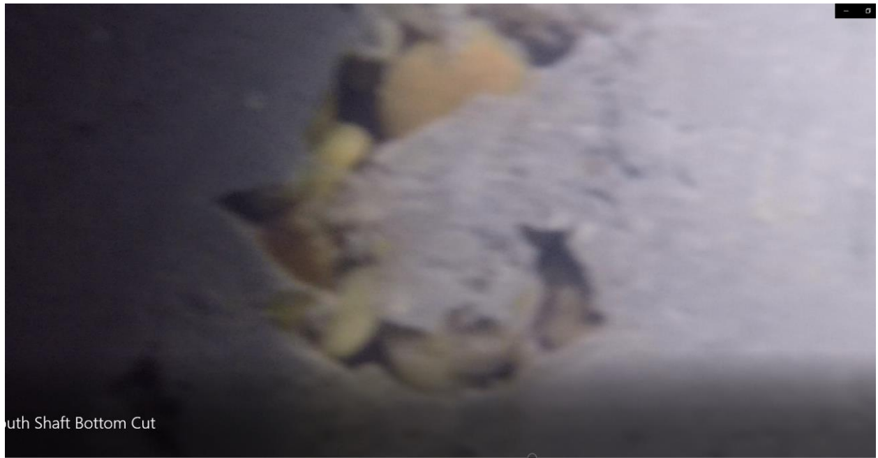
Figure 10.72 Shaft 58-2 with the casing removed from the lower portion of the shaft .
