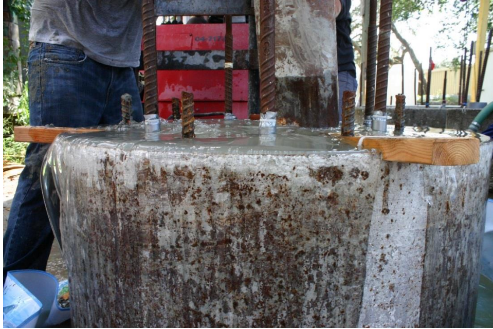
Figure 2.4 Polymer slurry exiting the form during concreting.
