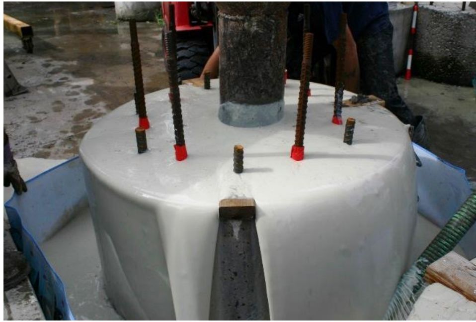
Figure 2.3 Attapulgite slurry exiting the form during concreting.
