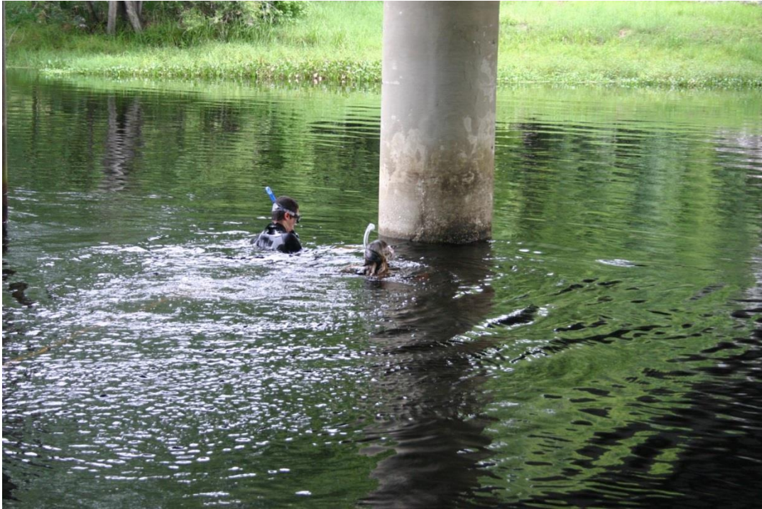
Figure 10.54 Diver follow-up to further review column-to-shaft interface.
