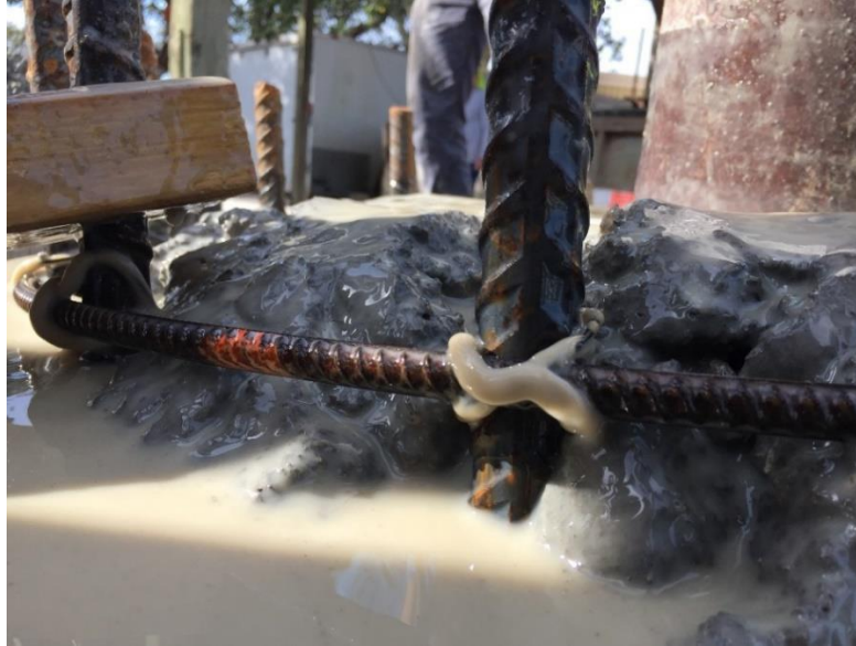
Figure 12.3 Bentonite coating on reinforcement and trapped around tie-wire.
