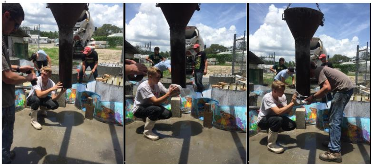
Figure 3.13 Tremie pipe preparation; placement of cap (left), covering of cap with plastic (center), taping of plastic around (not to) tremie pipe (right).
