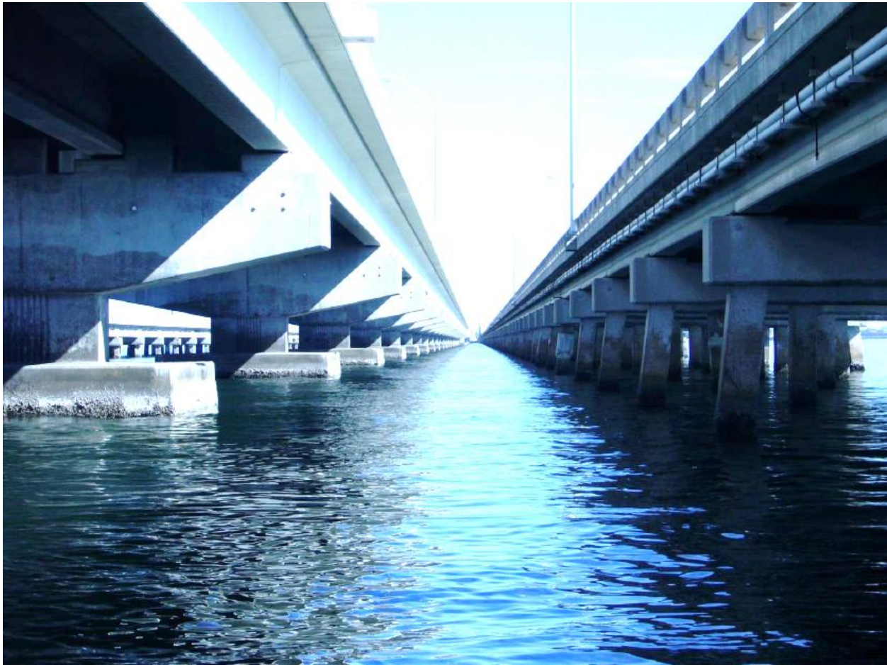
Figure 10.1 Newer cap and column pier design (left); older pile bent piers (right).
