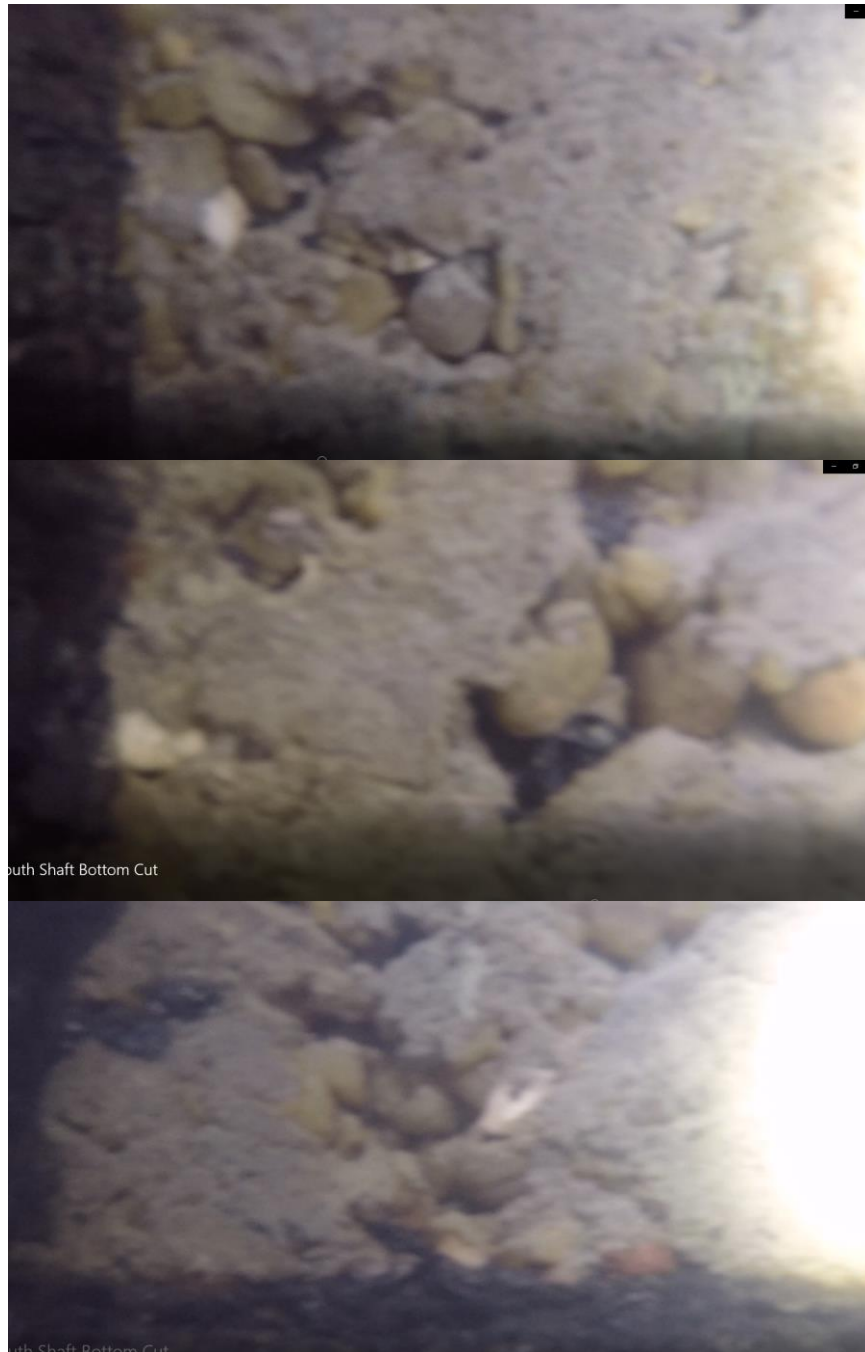
Figure 10.76 Shaft 59-2 with the casing removed from the lower portion of the shaft.
