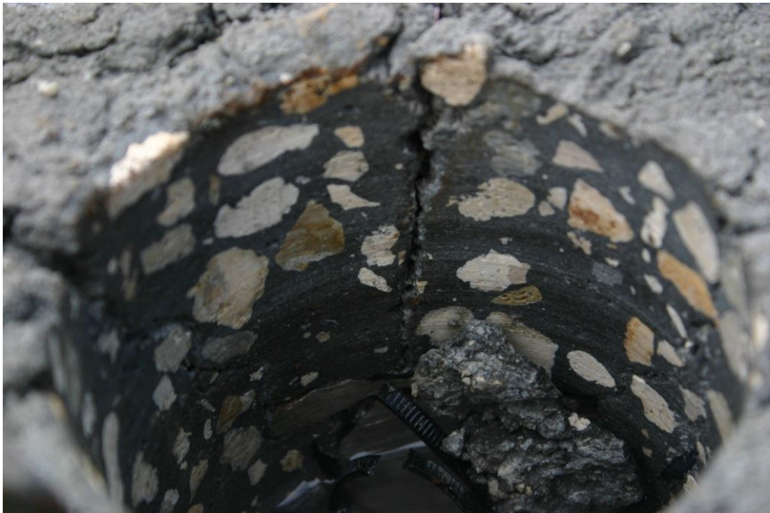
Figure 5.3 An empty core hole showing the surface crease extending to the reinforcing steel.
