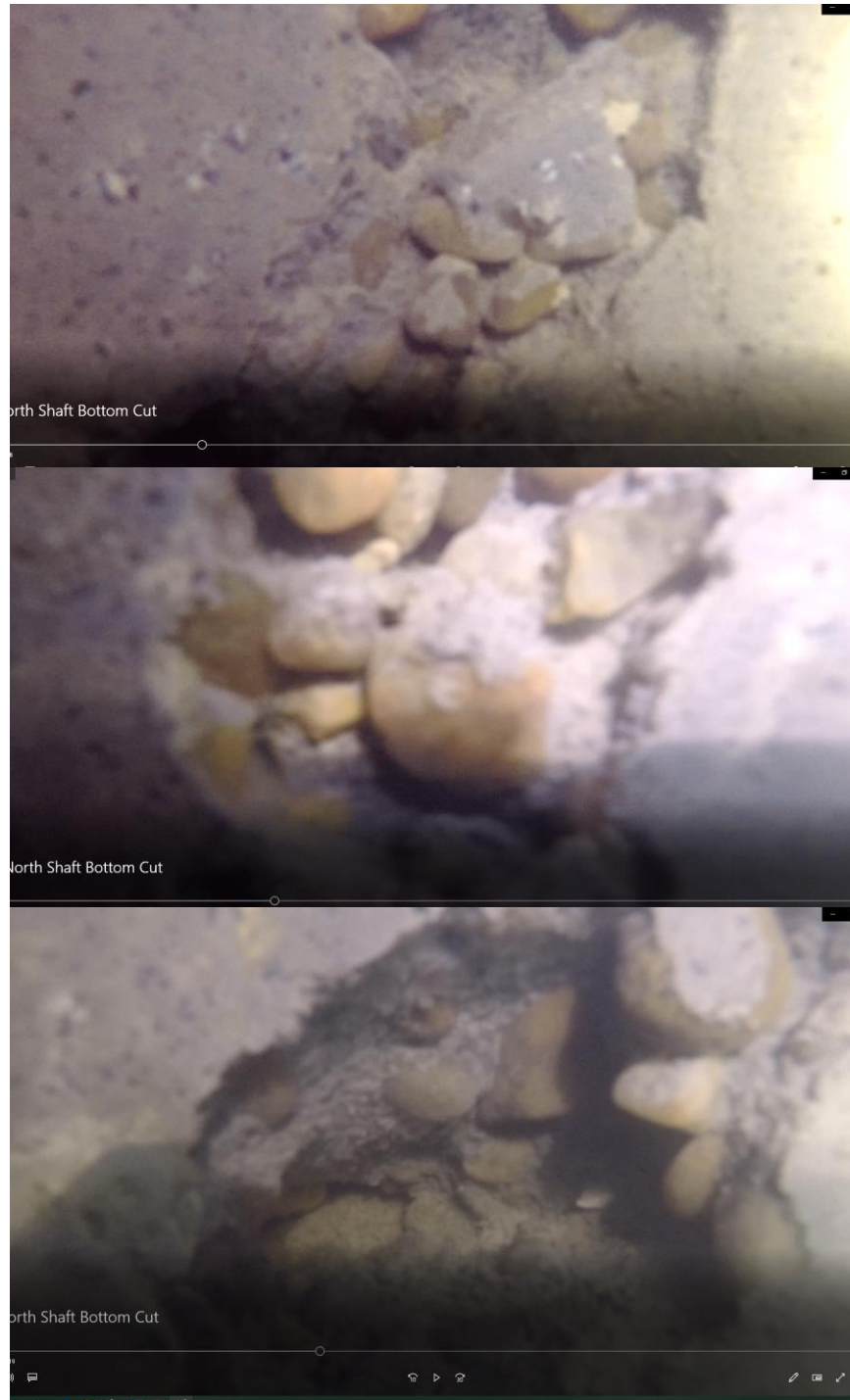
Figure 10.74 Shaft 59-1 with the casing removed from the lower portion of the shaft.
