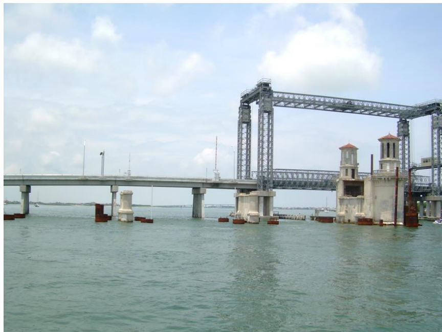
Figure 10.80 West Bascule (Pier 15; right), Piers 14 and 13 moving to the left with four 8-ft shaft casings shown from south looking north during rehabilitation.
