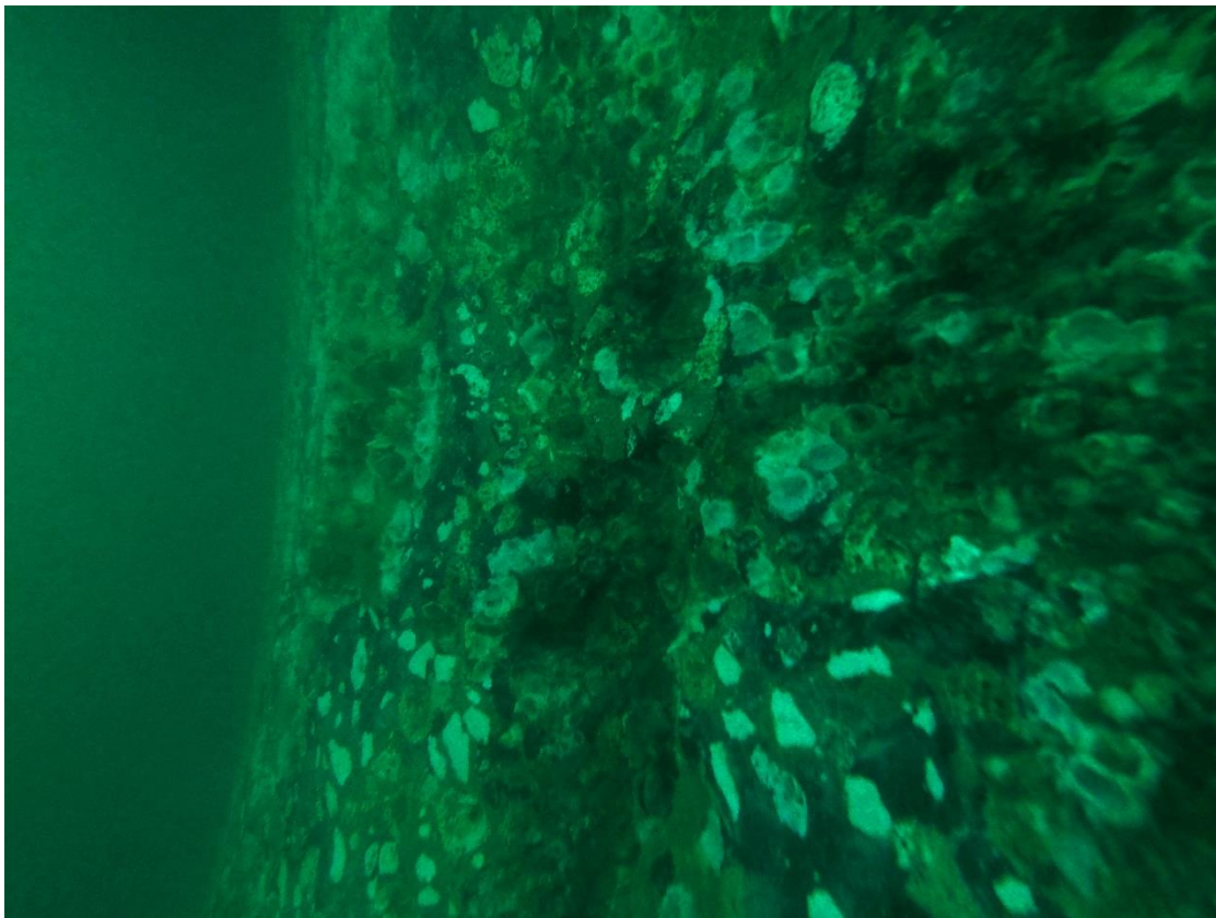
Figure 10.23 Large void found on the south side of 71-4.
