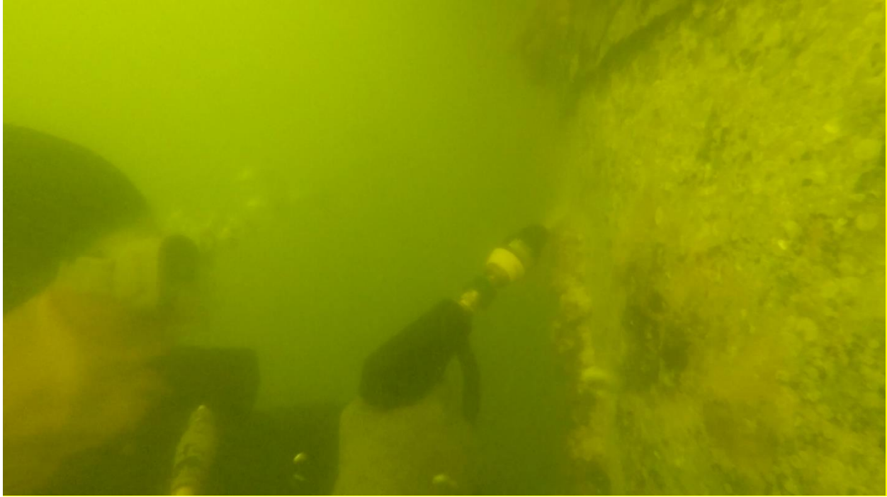
Figure 11.5 Pressure Washing Shaft Surface
