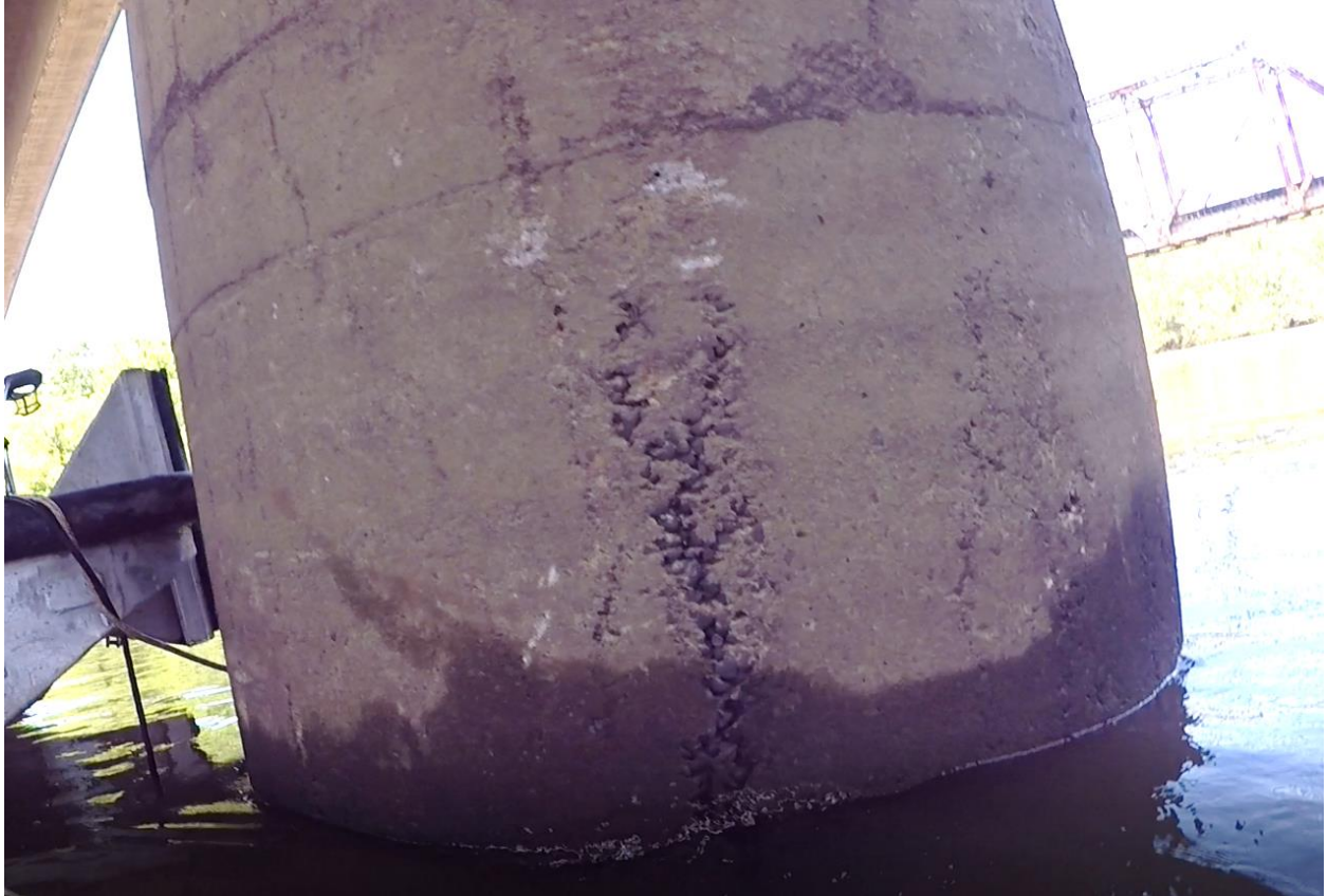
Figure 10.102 Shaft 15-1 upper casing had already been removed.
