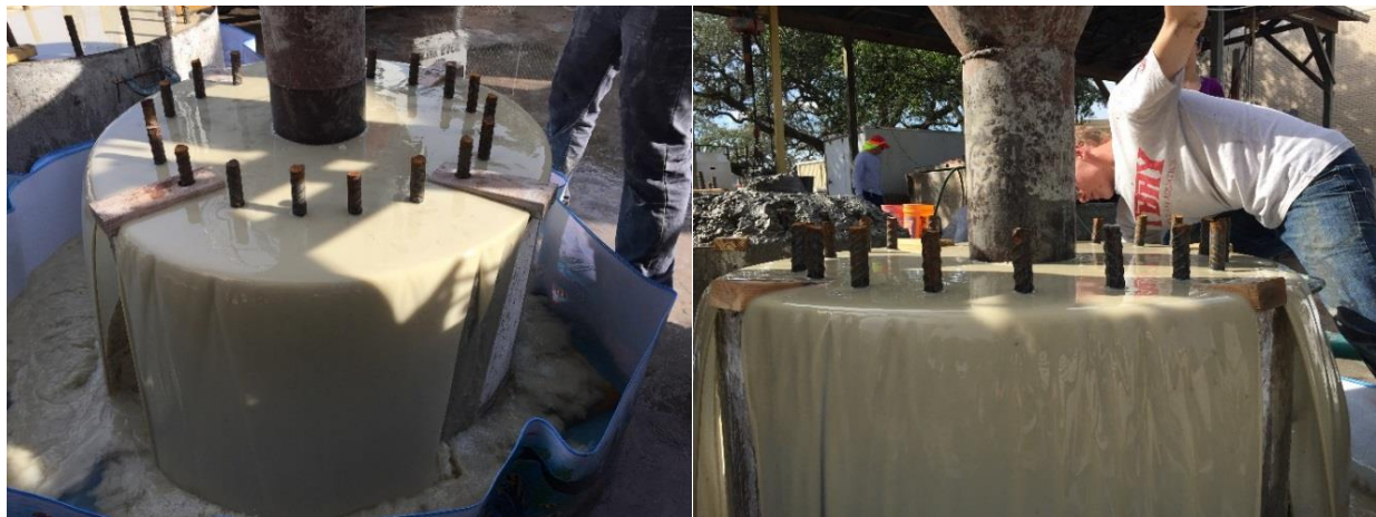
Figure 2.2 Bentonite slurry exiting the form during construction.
