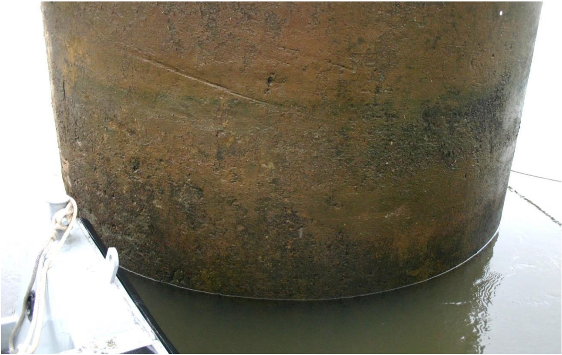
Figure 10.66 East side of test shaft 8 pre-cleaning.
