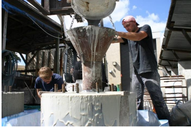
Figure 3.14 Displacement of slurry through the concreting process.
