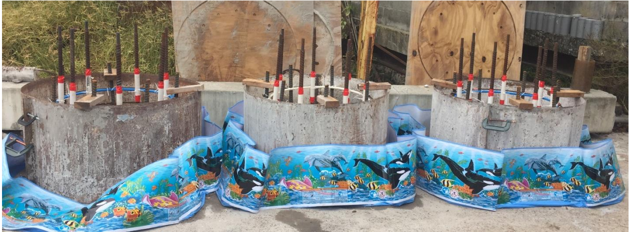
Figure 3.1 Forms set up prior to slurry and concrete placement.
