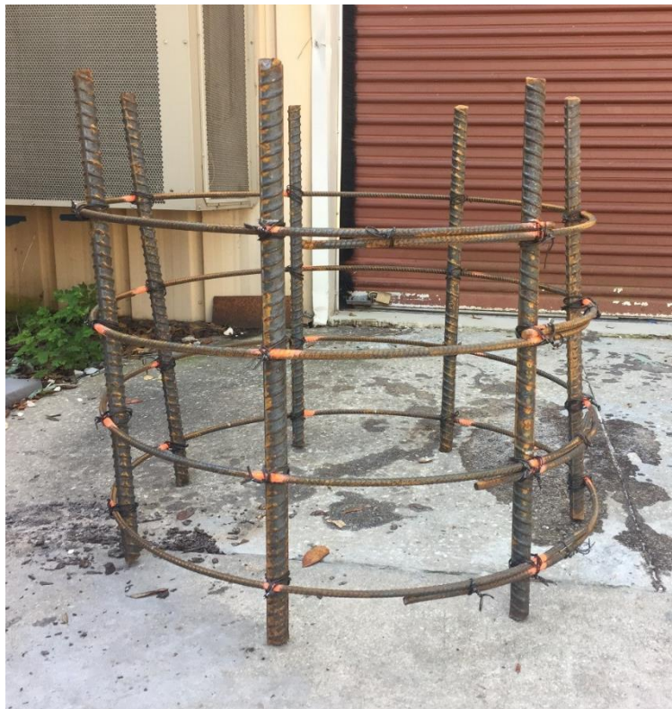
Figure 3.3 Outer seven longitudinal bars attached to the inside of the transverse reinforcement.
