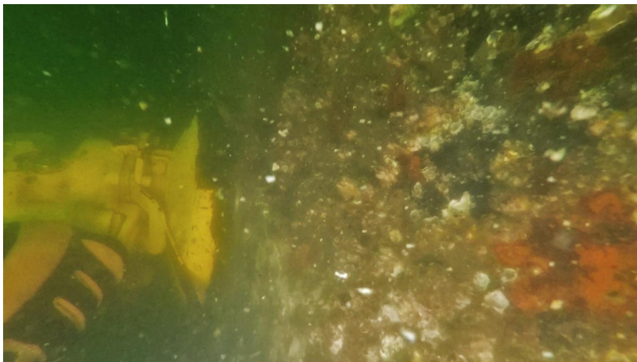
Figure 10.33 Shaft 94-4 during cleaning with the grinder.
