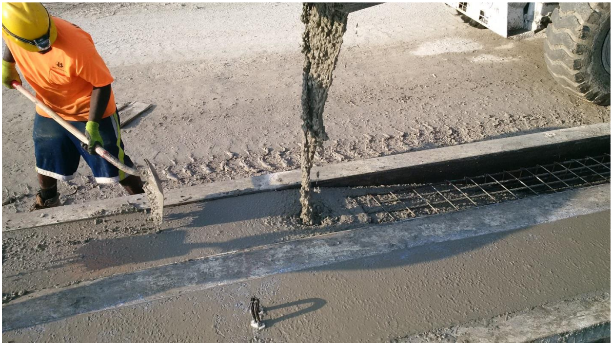
Figure 1.8 SCC used to cast prestressed piles requires almost no finishing as it pours out level.
