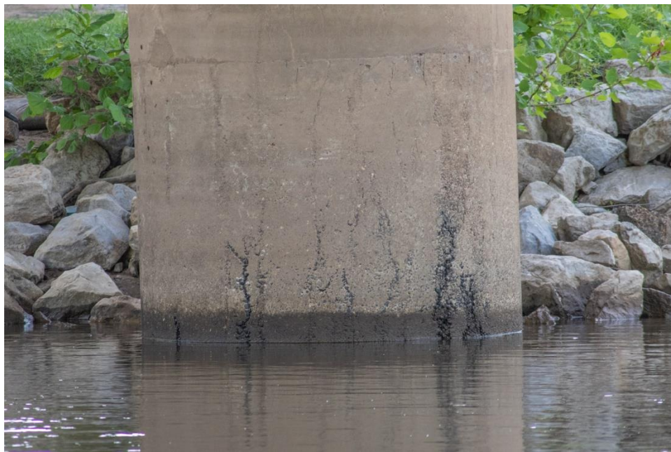
Figure 10.95 Drilled shafts displaying mattressing creases.
