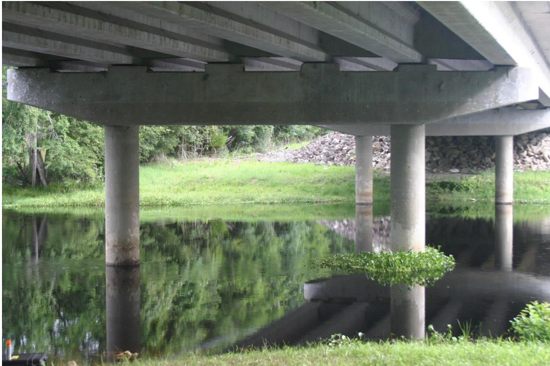
Figure 10.52 Four water column-to-shaft structures.
