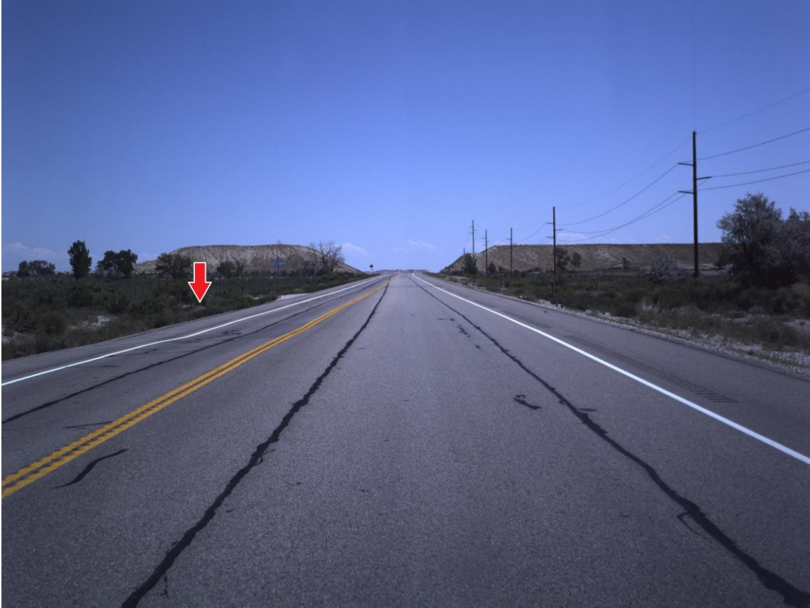
Figure 1.1 Photograph showing a visible “dip” in the negative direction of travel as indicated by the red arrow (Courtesy of UDOT/Mandli Communications)
