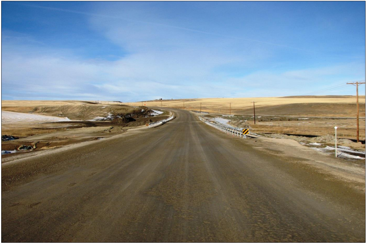
↑ Overview (north) of the completed GRS bridge installation.
