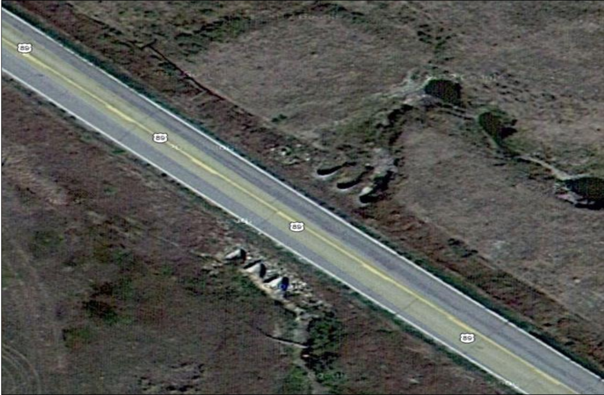
↑ Aerial view of preexisting culvert prior to installation of the GRS structure.
