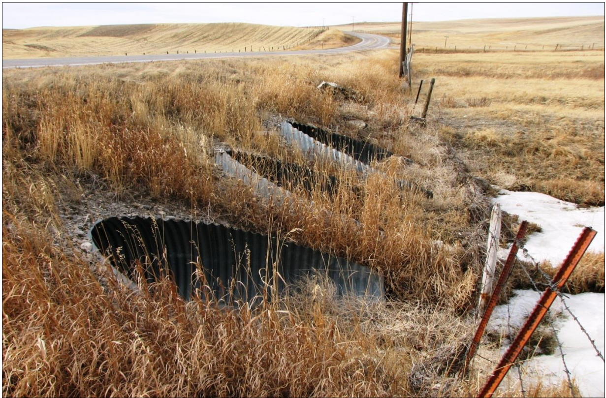
↑ Eastern side of corrugated steel pipe (CSP) culverts (view north).
