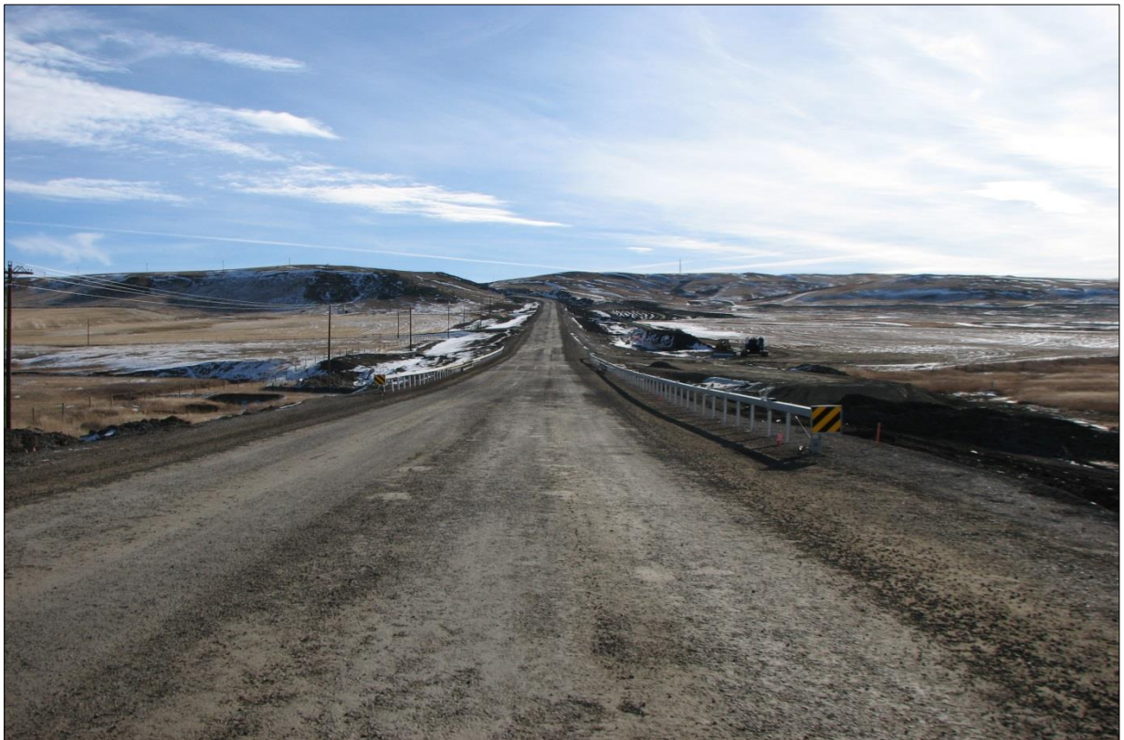
↓ Overview (south) of the completed GRS bridge installation.
