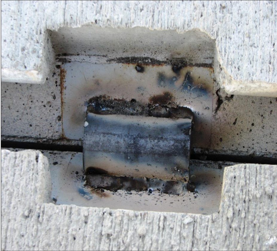
← Sample image of rod to plate completed weld.
