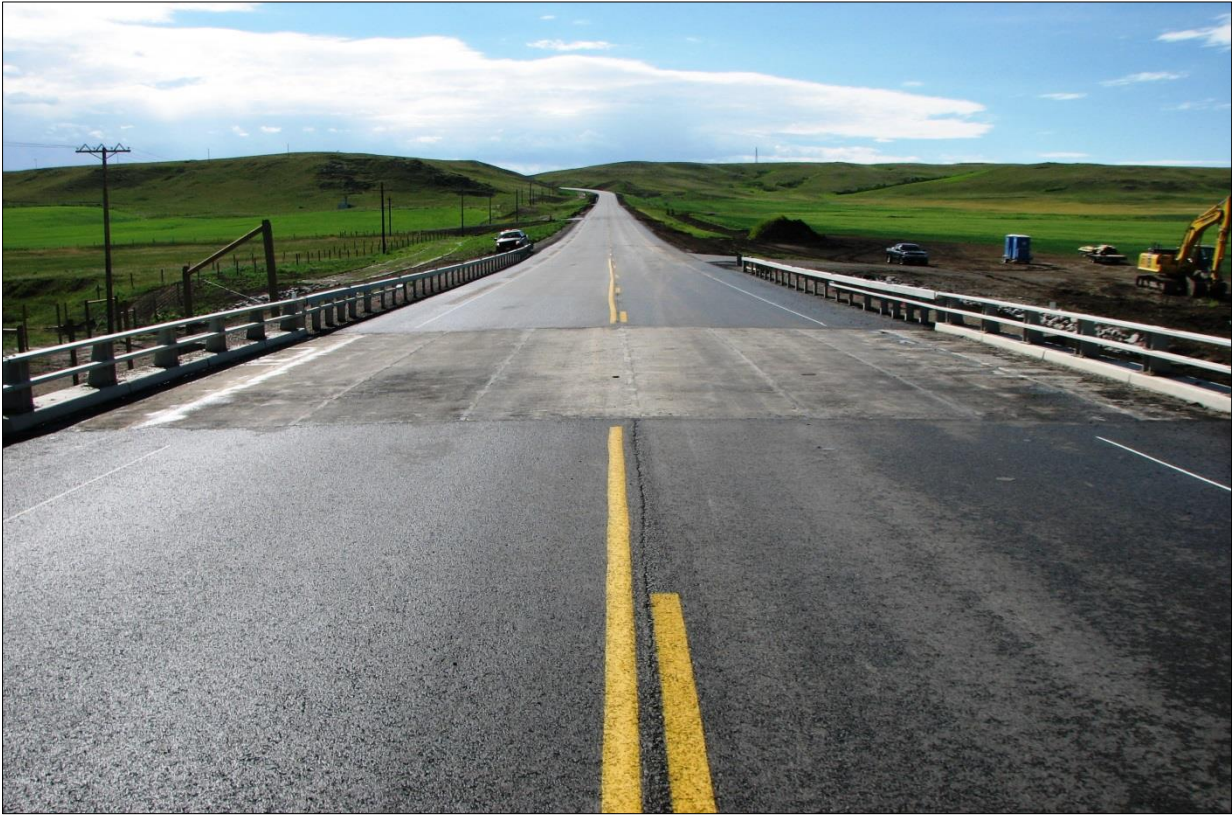
↑ Completed GRS structure; view south.
