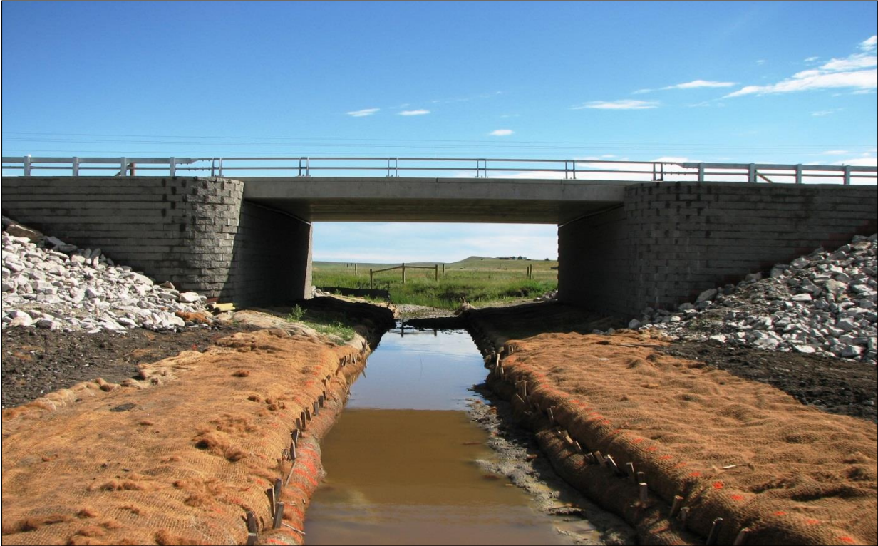
↓ Completed GRS structure; upstream view - east.
