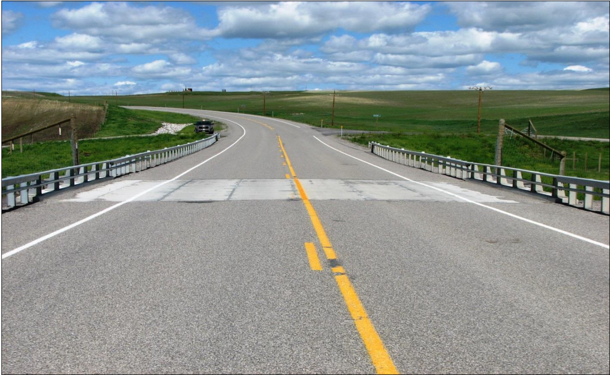
↑ Top view image of structure; view north.
