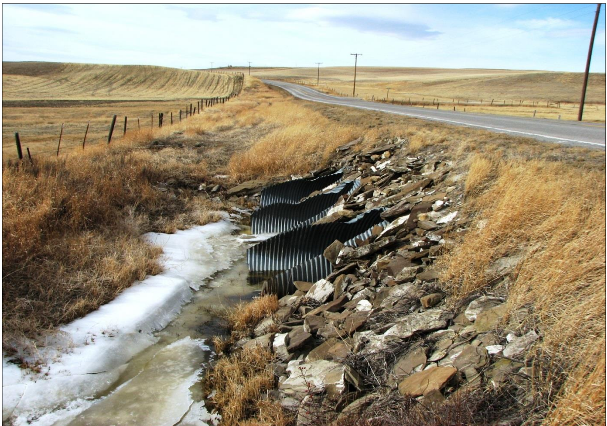
↑ Western side of culverts (view north).
