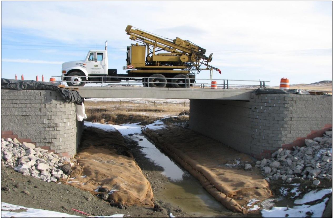
↑ View east of the completed GRS abutments and bridge installation. The truck on deck is the recently arrived crew to install the approach guardrails.
