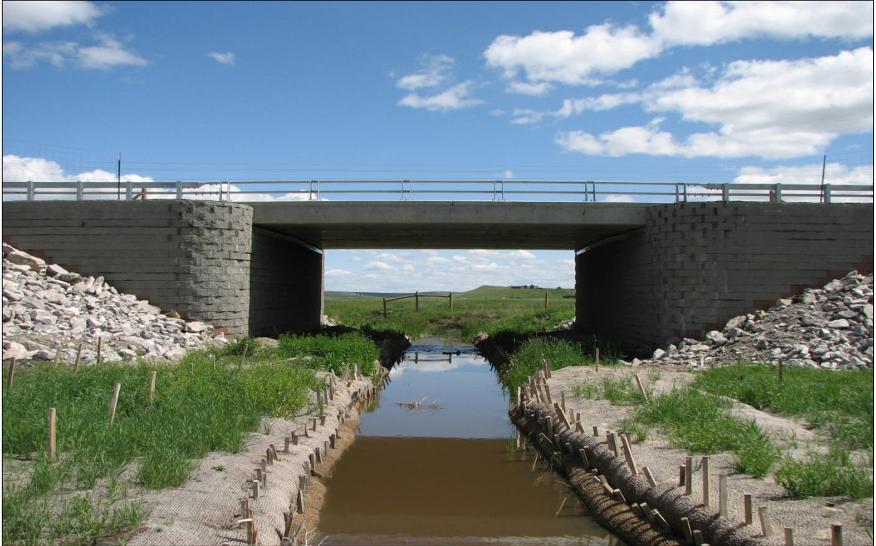
↓ Side view image of structure; view east.
