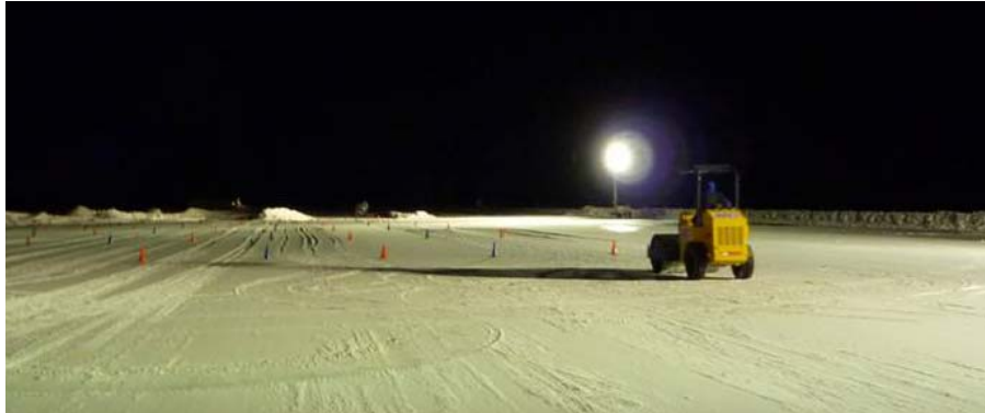
Figure 40: Compacting test sections with a smooth-drum compactor.
