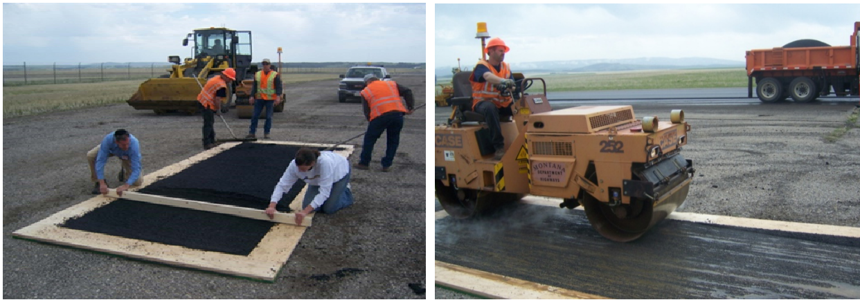
Figure 2: Screeding (left) and compacting (right) asphalt in plywood form.
