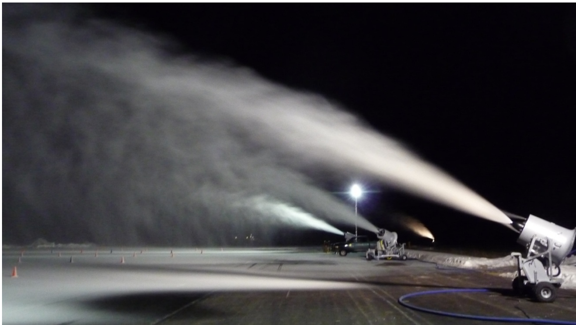
Figure 32: TRANSCEND snowmaking system in operation.
