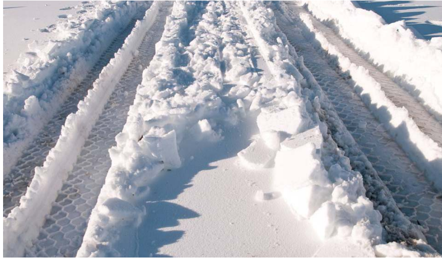
Figure 47: Deep snow compacted using the plow truck.
