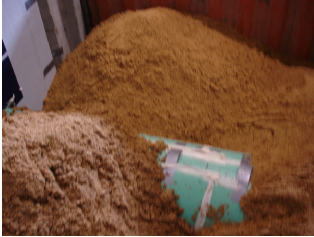
Step 7. Backfilling with sand.
