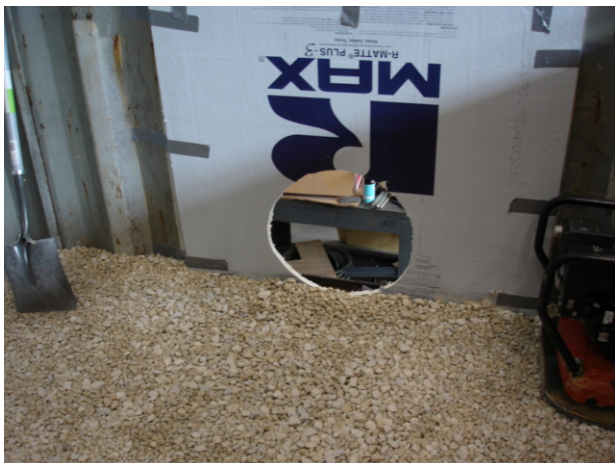
Step 5. Deposit gravel bedding layer.
