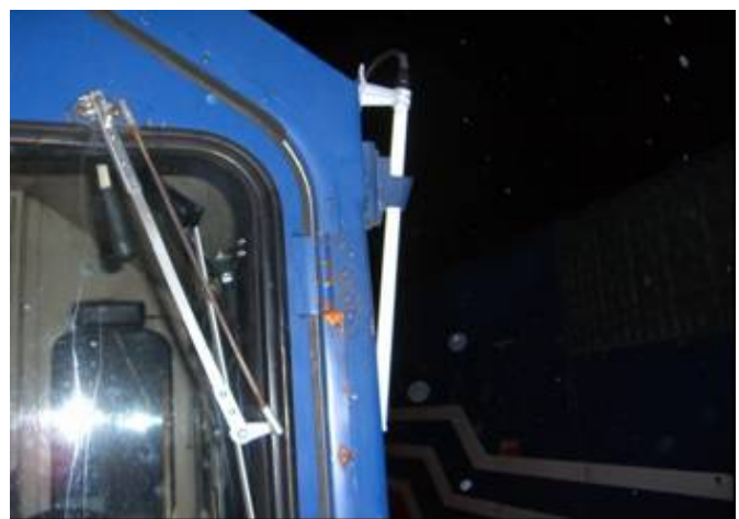
Figure 26: Antenna Installation on Locomotive V02
