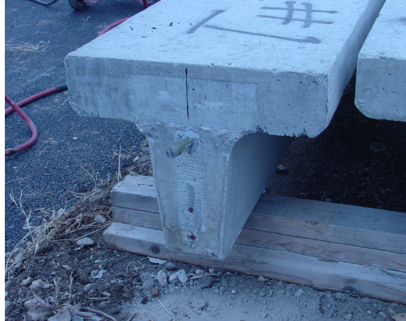
FIGURE 3.7. Inserted side bar used for flipping beams over.
