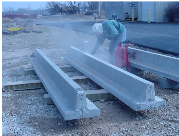
FIGURE 3.8. Concrete surface preparation by sandblasting.
